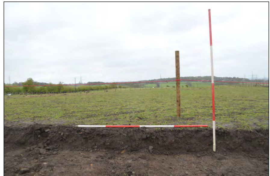
Photo 08. WNW facing section of the finished excavation area subject to watching brief (scales visible = 2 x 2m).
