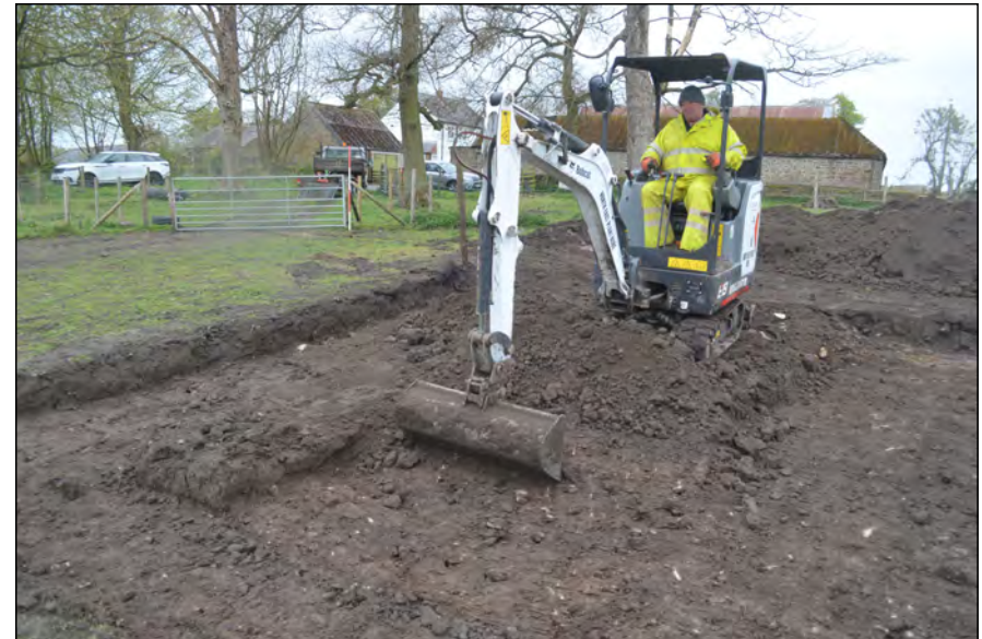
Photo 04. View looking WSW across the southern part of the watching brief site during excavation.
