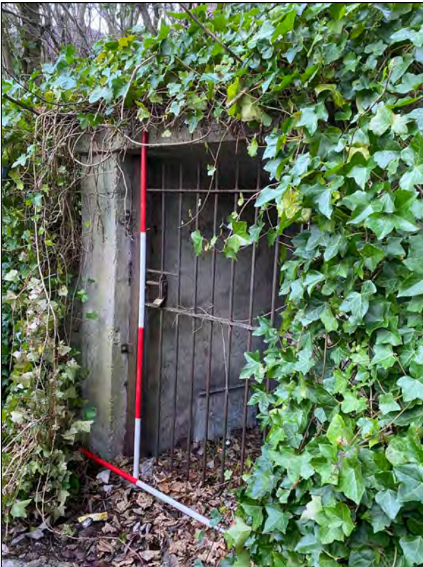
Photo 02. View of bunker entrance, looking south.
