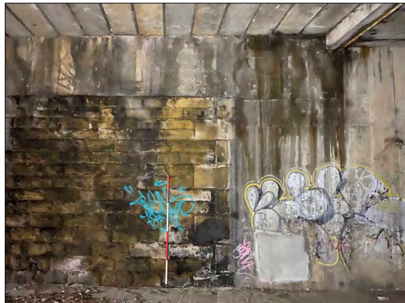
Photo 03. View near the east end of the tunnel, looking south.
