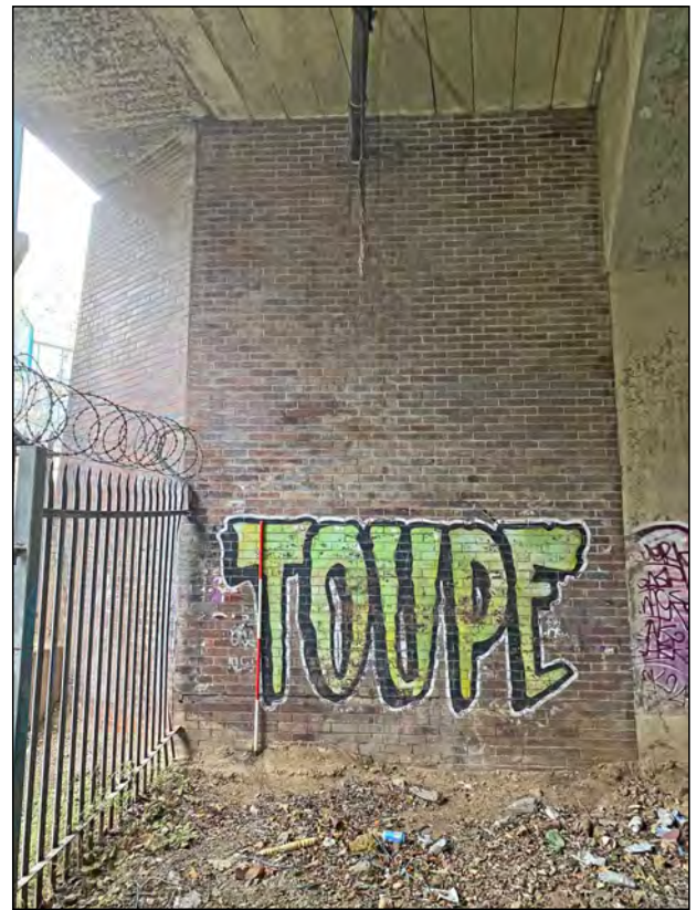
Photo 25. View looking north at the west end / entrance of the tunnel.
