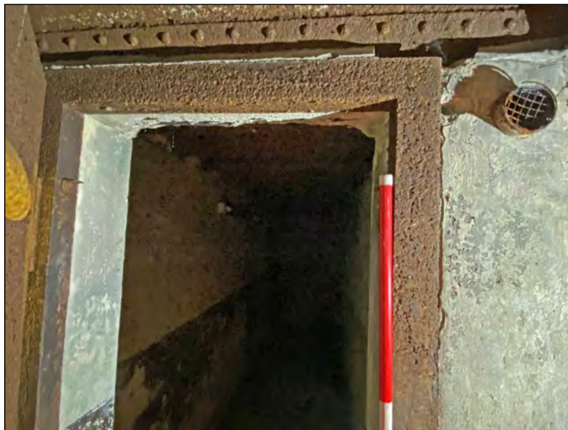
Photo 06. View of doorway surround at south-west end of entrance corridor.
