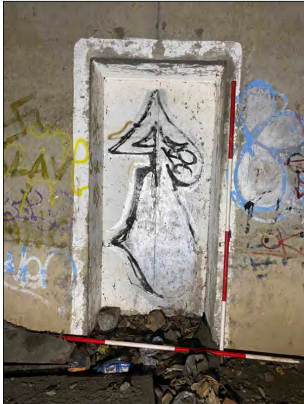
Photo 07. Detailed view of Retreat Alcove 1, looking north.
