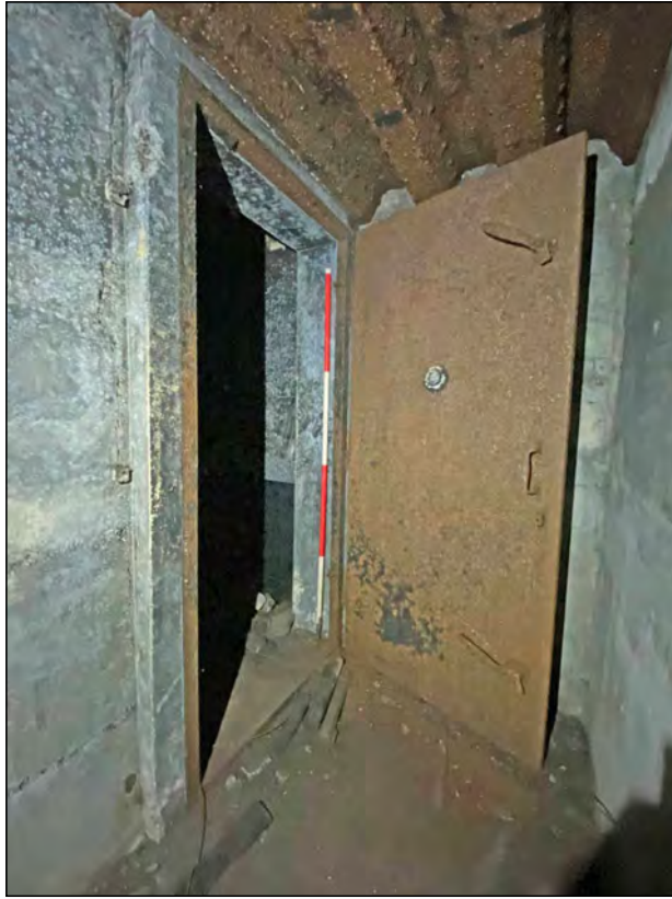
Photo 31. View of Room 2 entrance to exit corridor from steps.
