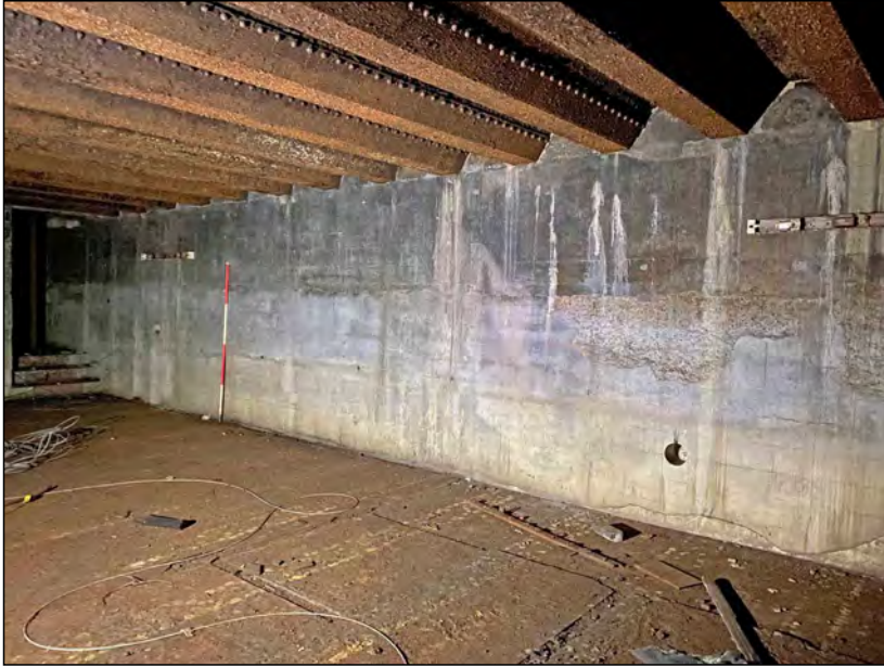
Photo 28. View of the west wall in Room 2.
