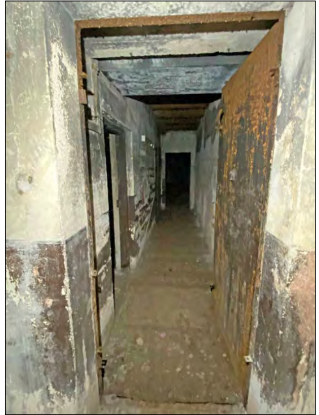
Photo 11. View of Room 1 and WC access corridor, looking SW.
