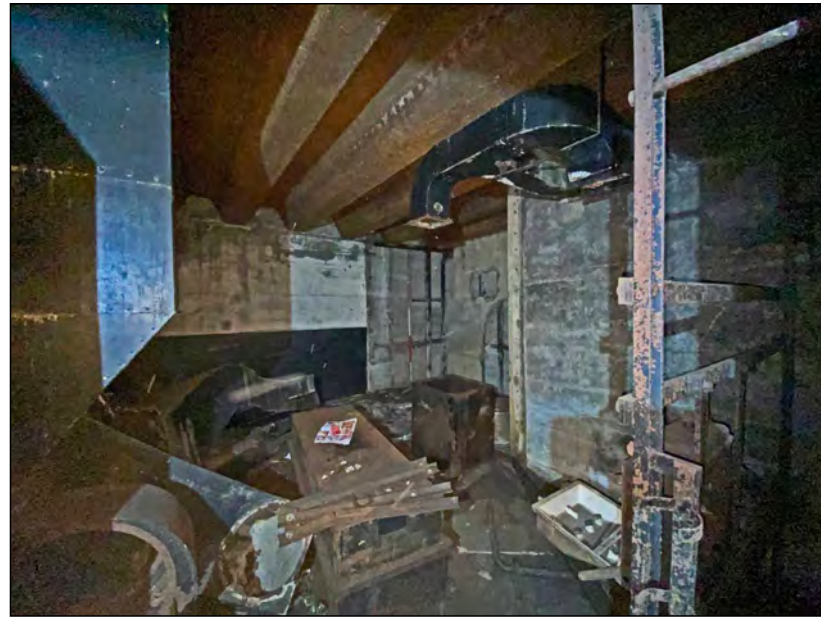
Photo 15. View of Room 1, looking east.
