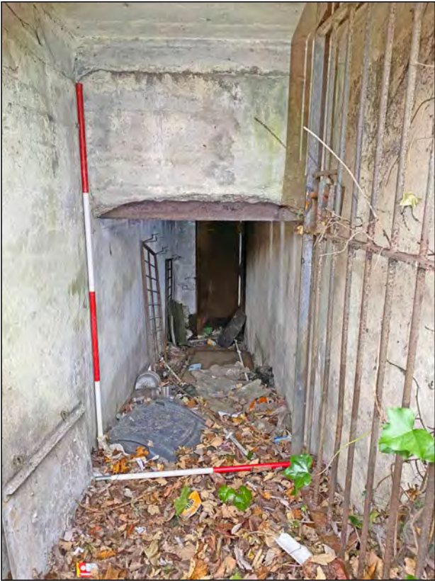
Photo 04. View of the entrance corridor, looking south-west.
