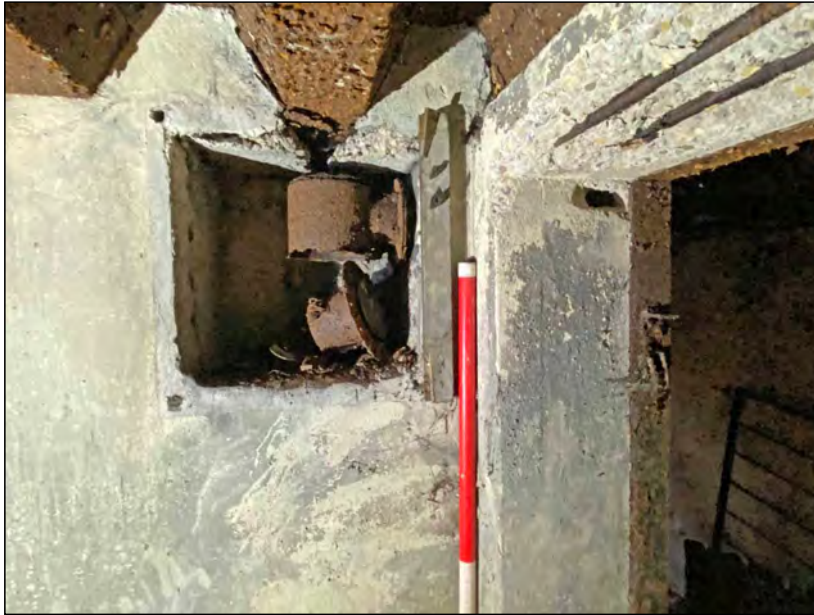
Photo 07. Inside door of internal SE-NW corridor.
