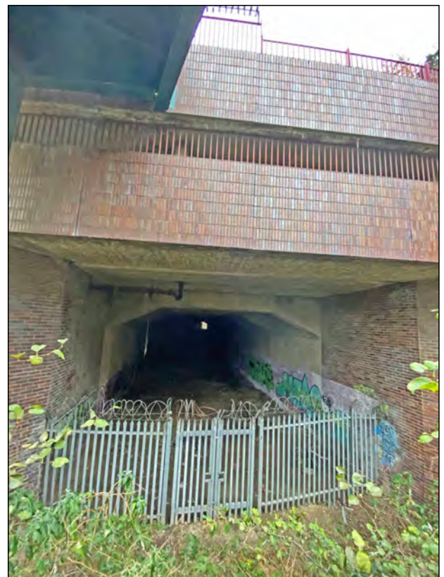
Photo 27. View looking east through the tunnel from the west end / entrance.
