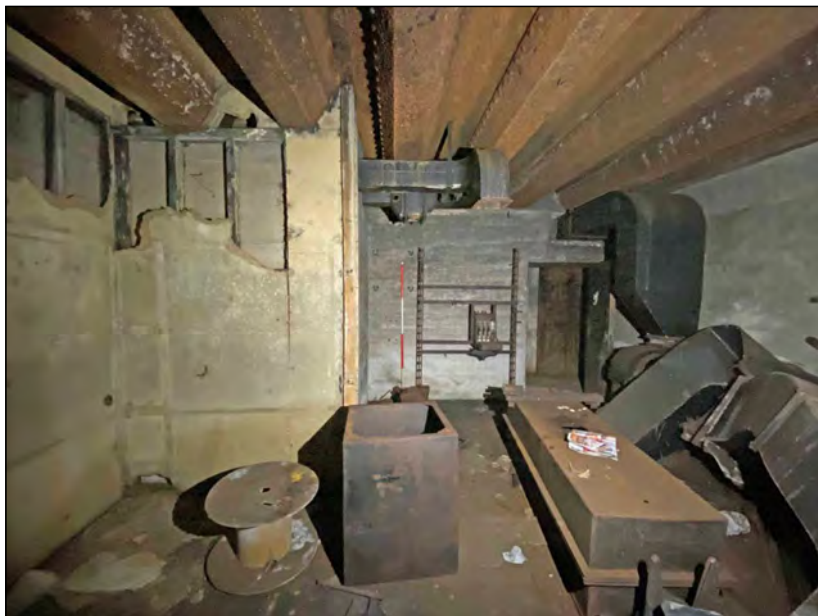
Photo 19. View of the west wall in Room 1.
