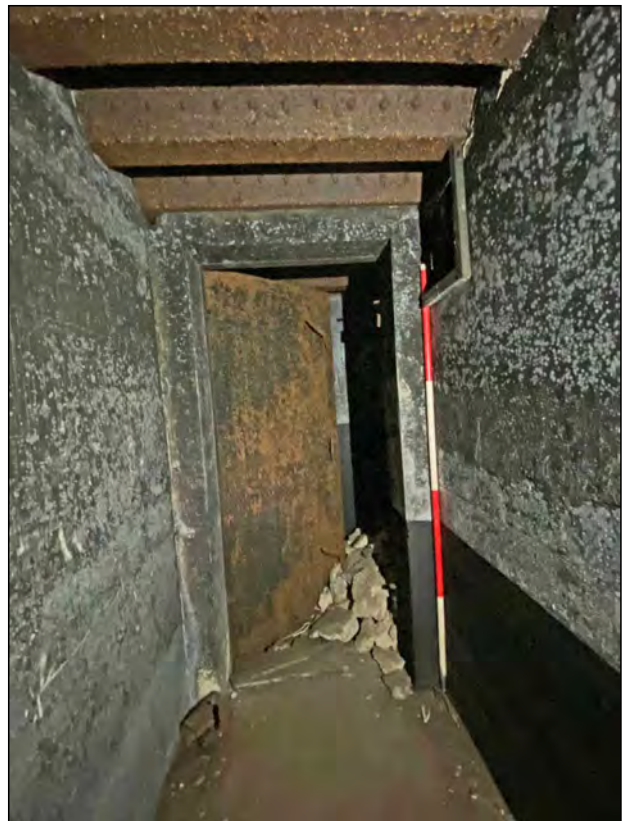
Photo 33. View of door at SE end of exit corridor.
