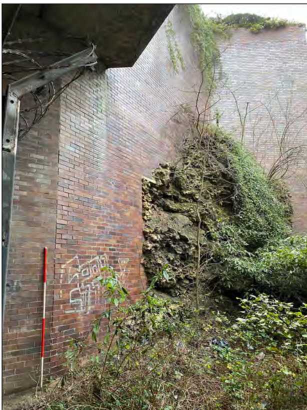
Photo 26. View looking south at the west end / entrance of the tunnel.
