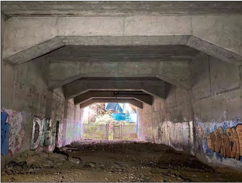
Photo 20. View looking west near the west end of the tunnel.
