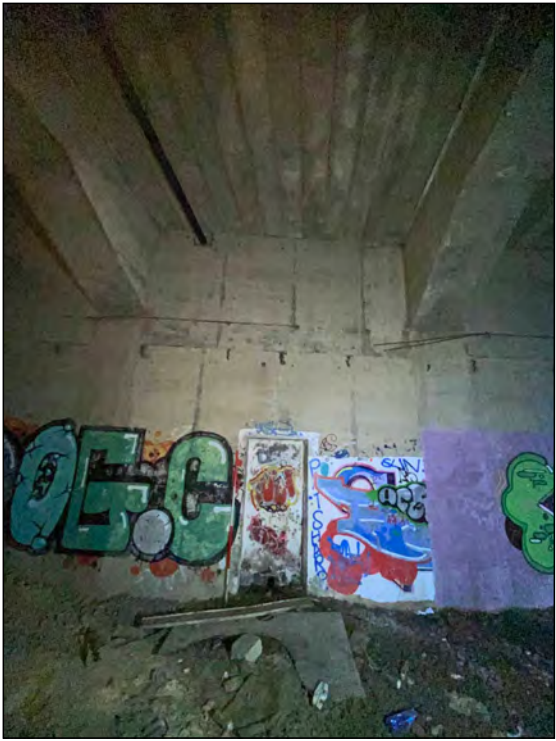
Photo 22. Broad view of Retreat Alcove 08, looking south.
