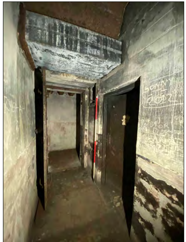
Photo 13. Entrance to Room 1 and WC access corridor, looking NE.
