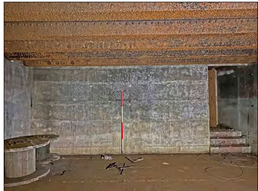
Photo 27. View of the south wall in Room 2.
