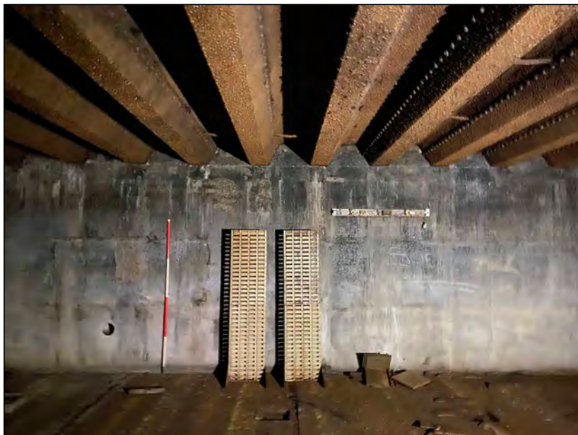
Photo 26. Alternative view of the east wall in Room 2.
