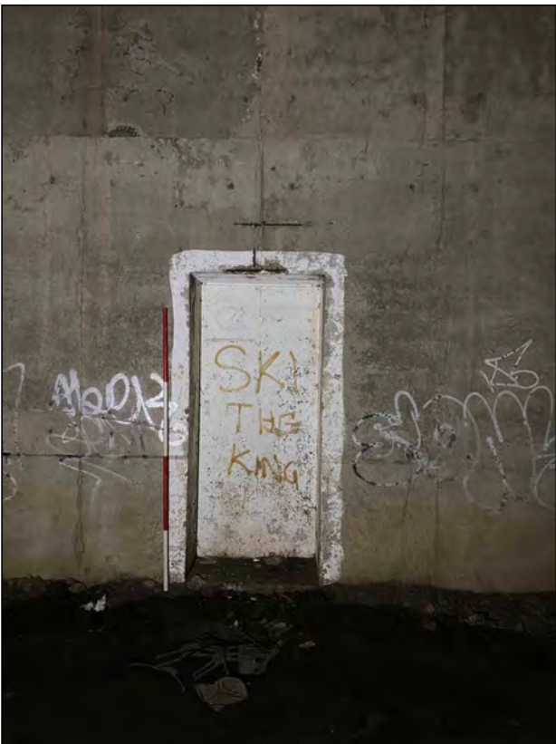
Photo 12. Detailed view of Retreat Alcove 03, looking north.
