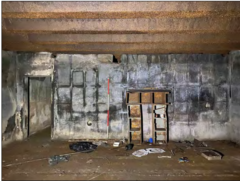
Photo 24. View of the north wall in Room 2.
