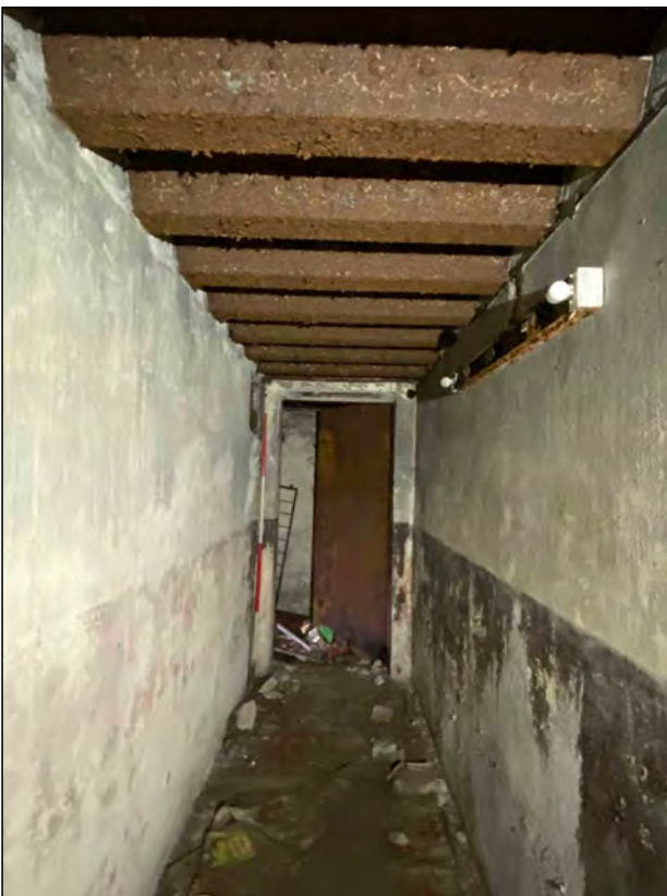
Photo 08. View of internal corridor, looking SE.
