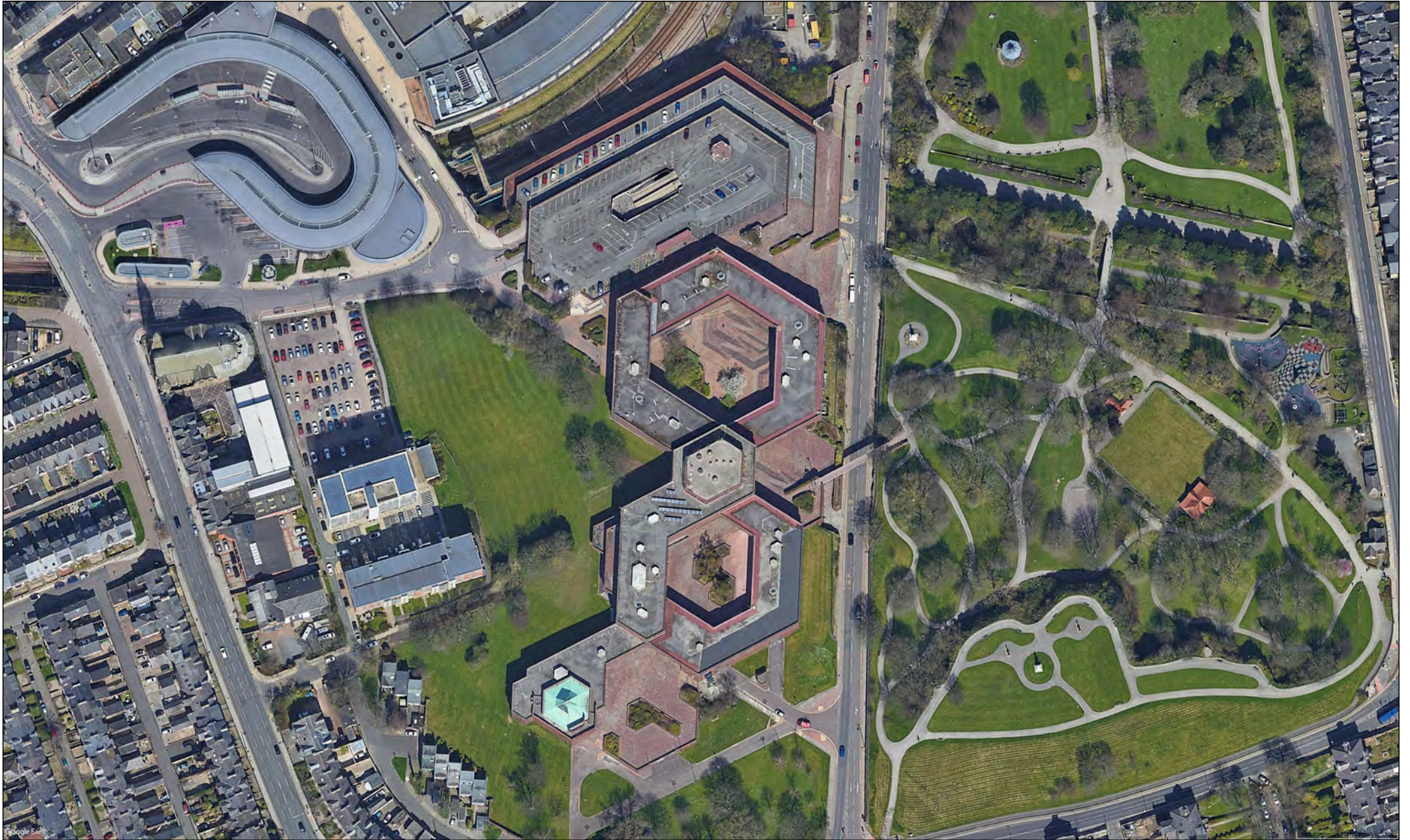
Illus. 16: Aerial view of Sunderland Civic Centre, April 2018. Courtesy of Google Earth.
