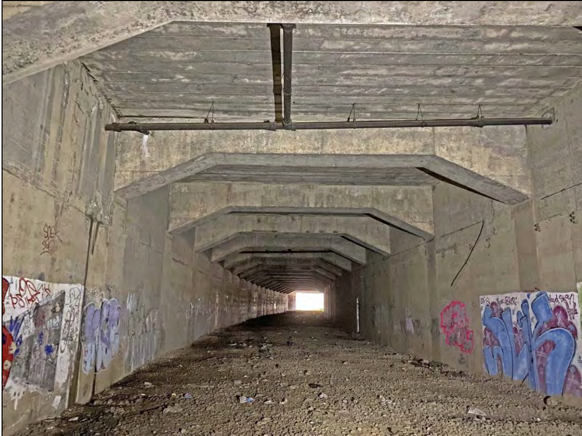
Frontispiece: Looking through the former railway tunnel beneath Sunderland Civic Centre, view looking east.
