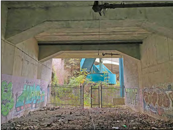
Photo 24. View looking west at the west end / entrance of the tunnel.
