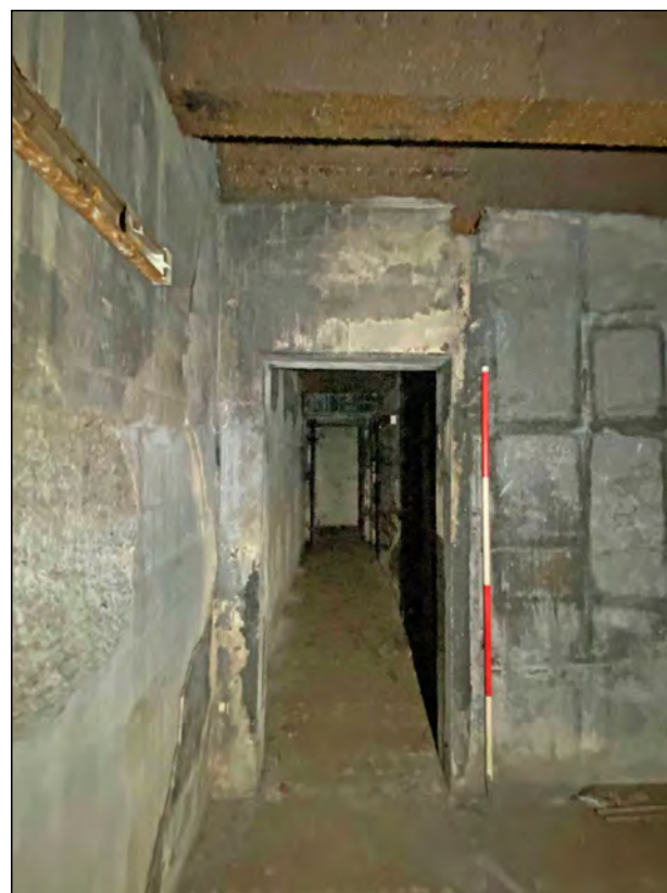
Photo 23. View of the entrance to Room 2 from NE-SW corridor, looking NE.
