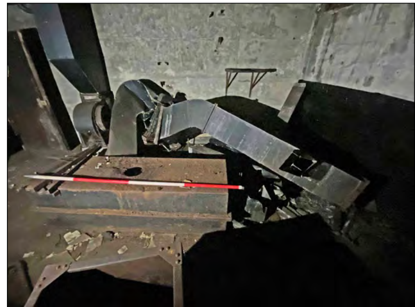
Photo 20. View of the north wall in Room 1.
