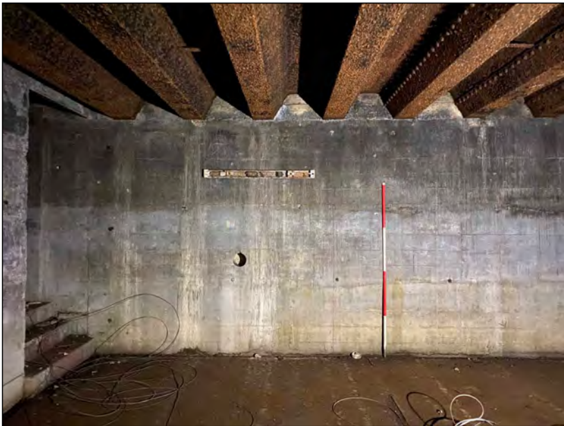
Photo 29. View of the south end of the west wall in Room 2.
