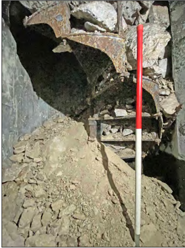
Photo 37. View of blocked spiral stair exit located at the SW corner of the bunker.
