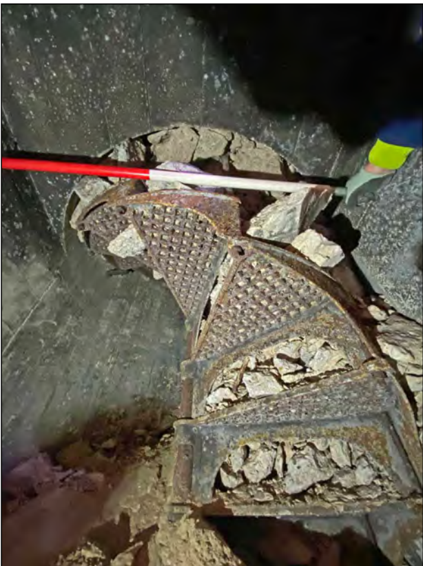
Photo 38. Looking upwards at blocked spiral stair exit.
