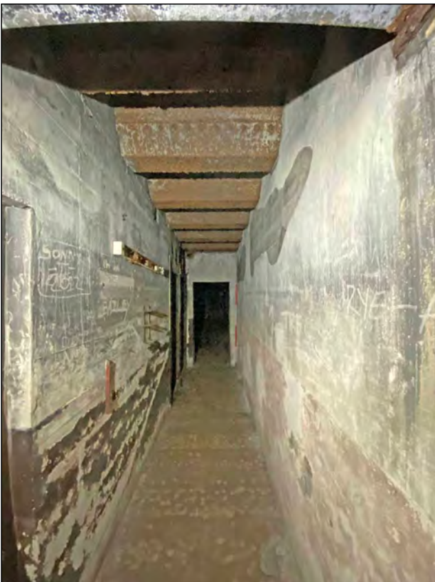
Photo 12. View of WC access corridor, looking SW.
