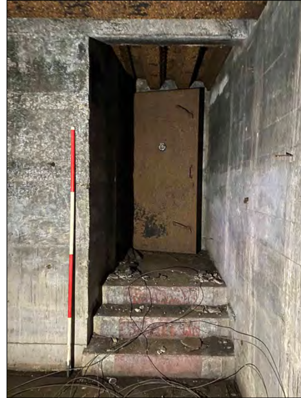
Photo 30. View of steps through the south wall of Room 2.
