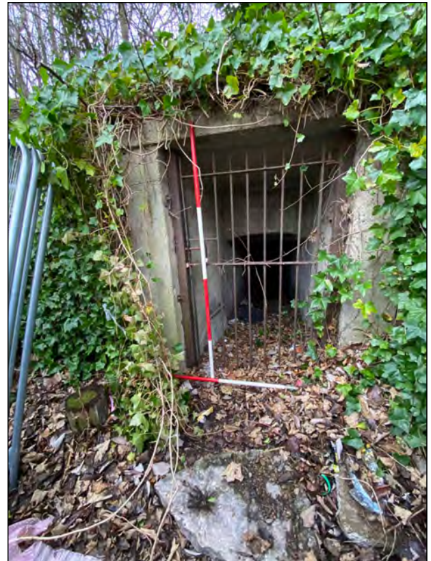
Photo 03. View of bunker entrance, looking south-west.
