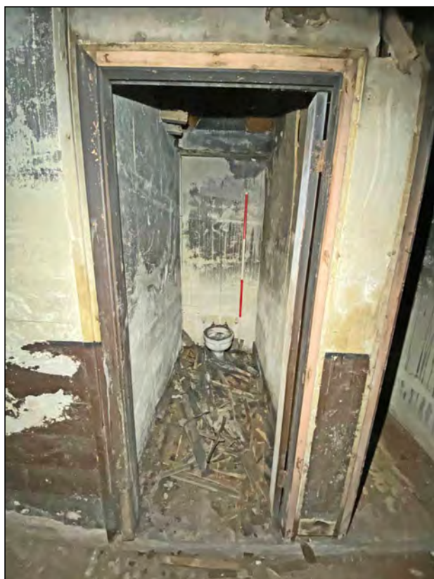
Photo 22. View of WC cubicle in NE-SW corridor, view looking SE.
