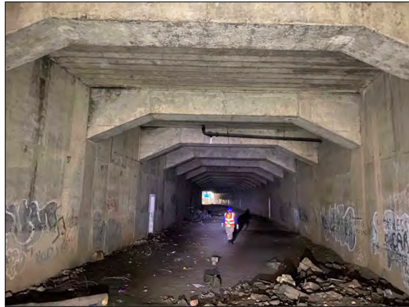
Photo 08. View looking west along the tunnel, from between Retreat Alcoves 01-02.
