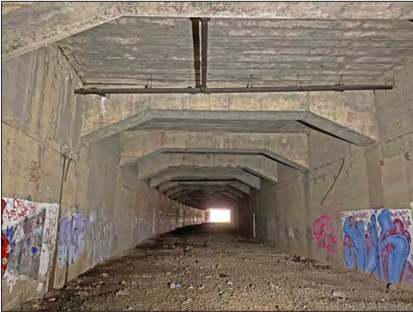
Photo 21. View looking east from near the west end of the tunnel.
