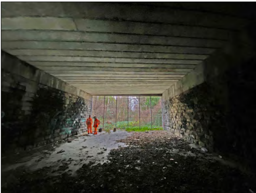
Photo 04. View looking east towards the east end of the tunnel.
