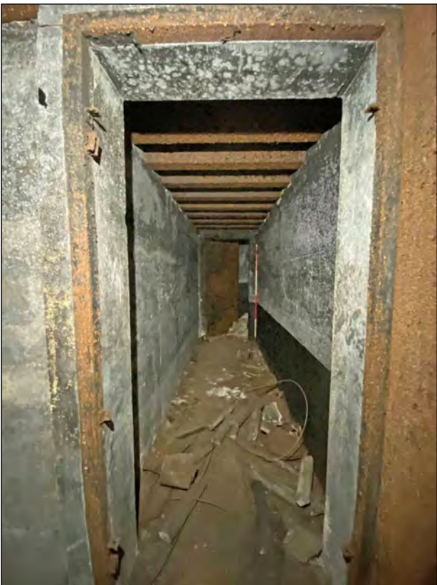
Photo 32. View of NW-SE exit corridor, looking SE.
