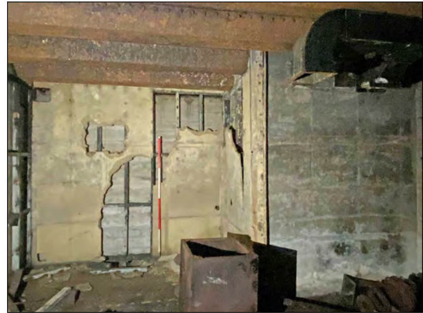
Photo 18. View of the south wall in Room 1.
