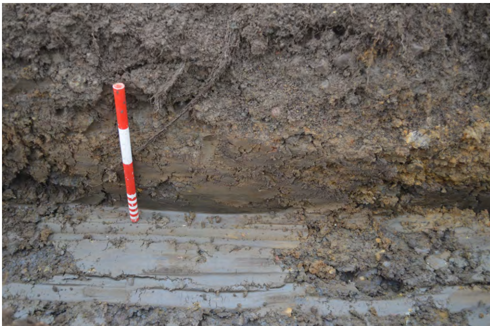
Photo 11. West facing view of north-south section of trench west of water treatment tank.
