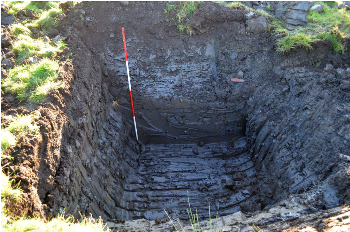
Photo 02. The pit for the water treatment tank, excavated to full depth.
