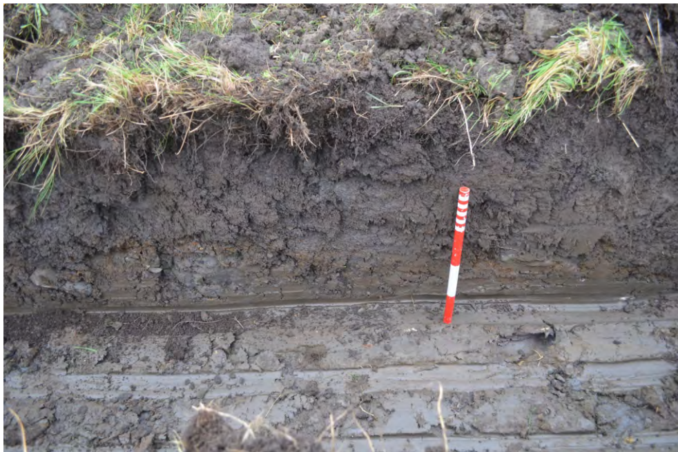
Photo 05. West facing view of section of trench east of water treatment tank.
