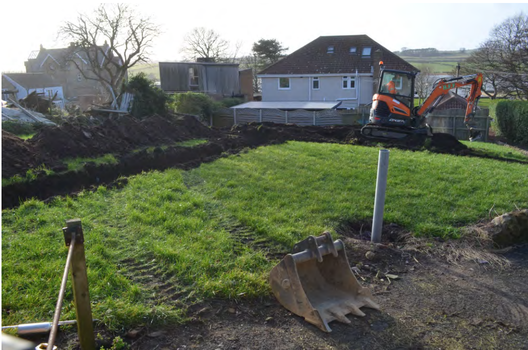
Photo 06. Overview shot, showing Trenches 1 and 2, south west view.
