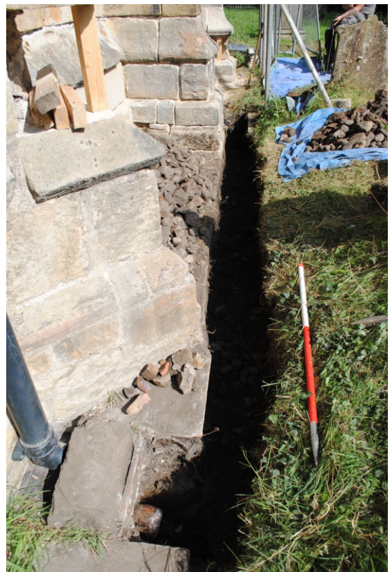
Photo 12. East view of pipe trench alongside the 'Lady Chapel'.
