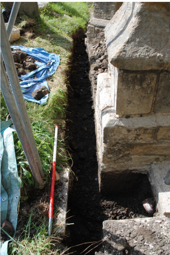
Photo 11. West view of pipe trench alongside the 'Lady Chapel'.
