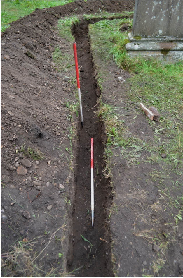
Photo 13. East view of pipe trench, east of the 'Lady Chapel'.
