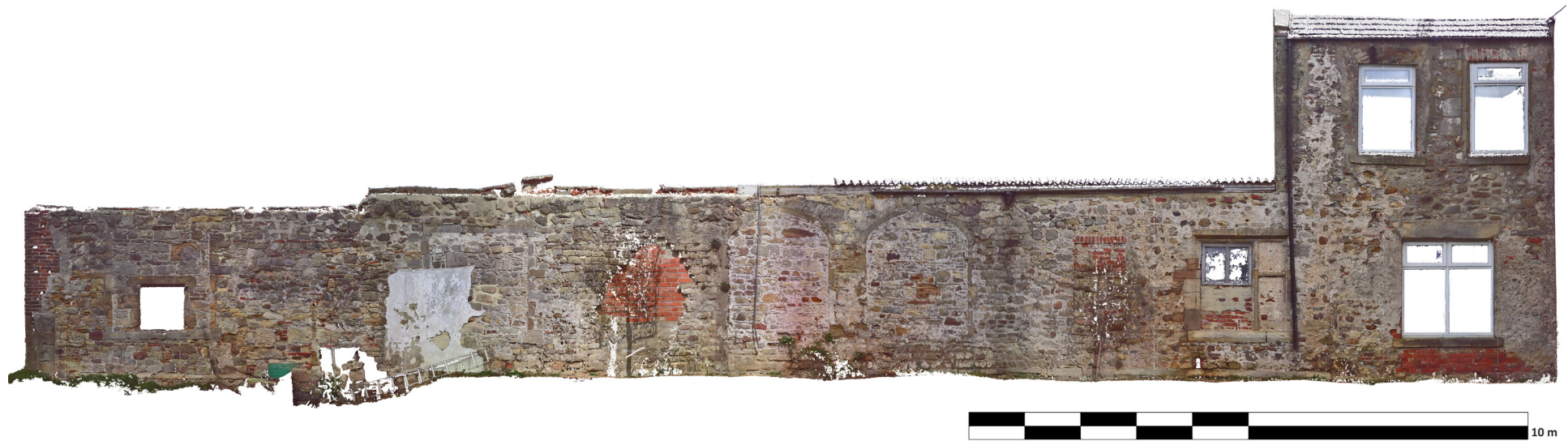
Illus. 14: Digital scan showing south facing elevation of south wall, The Chapel, Great Isle.
