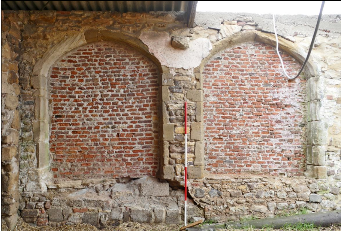
Frontispiece: View of blocked late-medieval four-pointed windows, with moulded surrounds and indications of tracery, located in the internal, north-facing elevation of the 'Chapel' Range.
