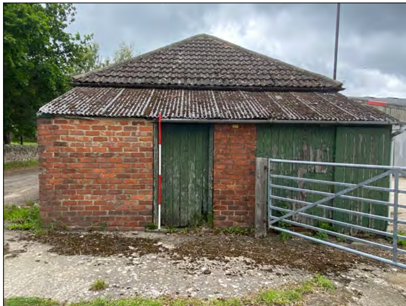
Photo 35. The south elevation of the detached brick-built north-west range, orientated N-S.
