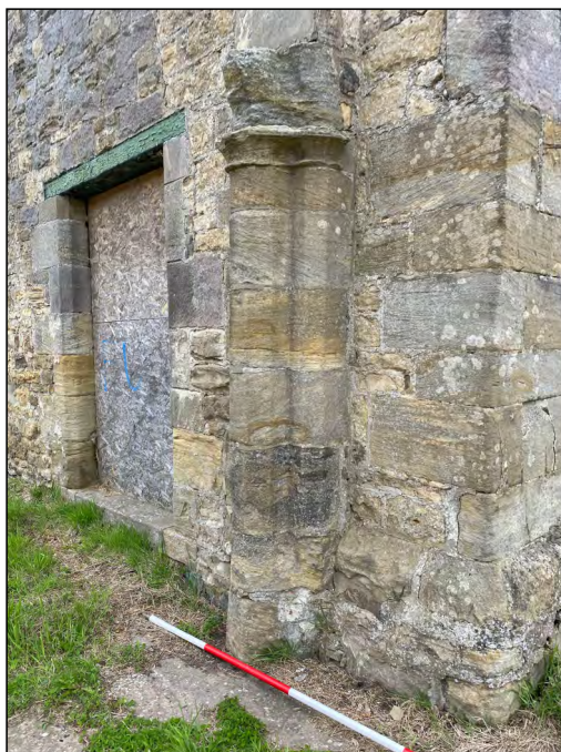
Photo 17. View from the north-east of the remains of a double-chamfered respond of an arch, springing eastwards at the north end of the east elevation of the 'old hall', with a shallow impost moulding below a single surviving voussoir.
