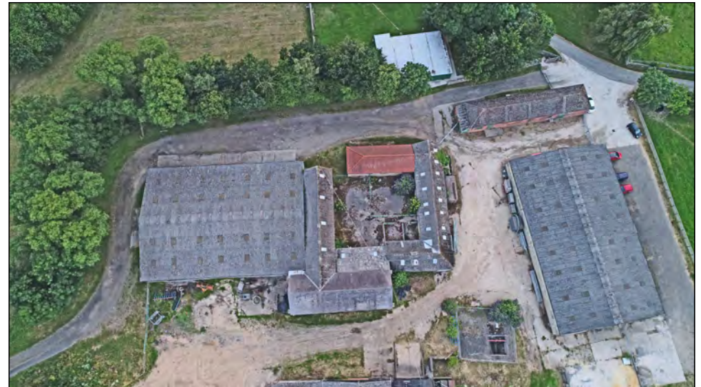
Photo 04. Near-vertical aerial view of Hall Farm from ESE.
