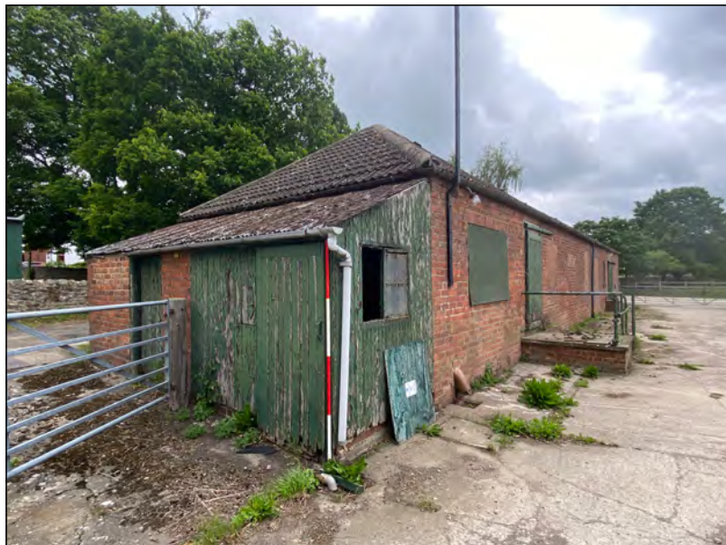
Photo 43. The south (left of view) and east elevations of the detached north-west range seen from the south-east.
