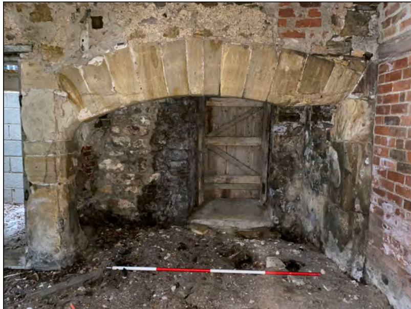
Photo 59. Fireplace in the south part of the internal face of the west wall of the 'Old Hall'.
