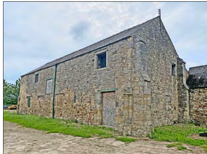
Photo 16. The north (right of view) and east elevations of the 'old hall' seen from the north-east.
