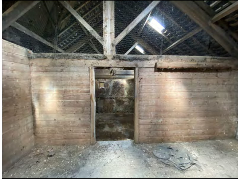
Photo 77. View north to the north end of the first-floor space.
