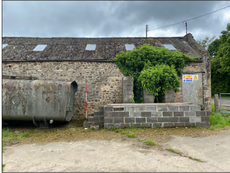
Photo 09. The west part of the north elevation to the north range
