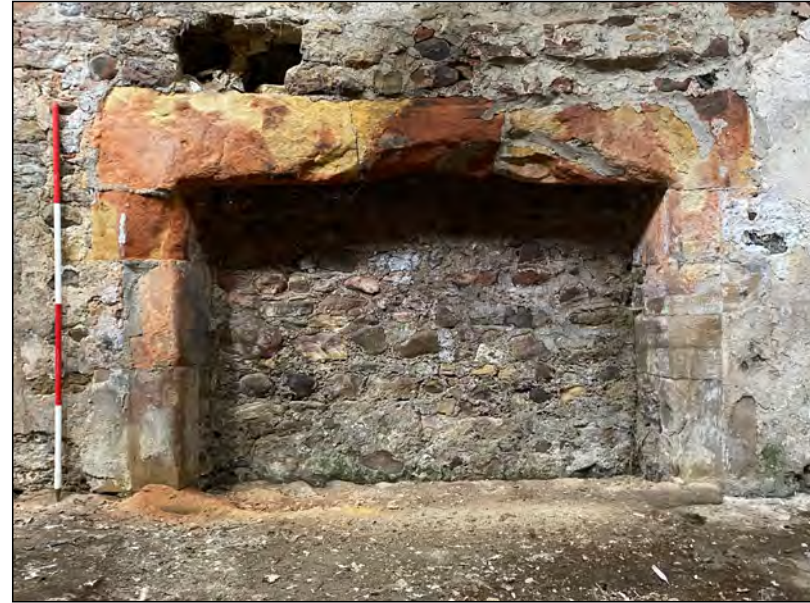
Photo 66. Fireplace in the N part of the internal (E-facing) W wall of the 'Old Hall', with signs of decay clearly visible in the mound of sand from the decayed lintel, particularly against the south jamb.
