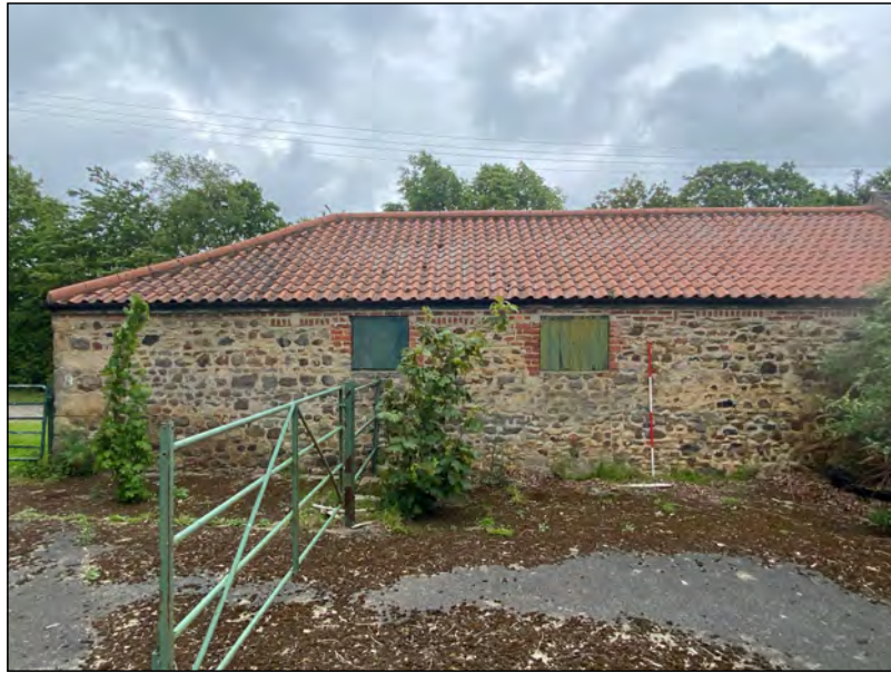
Photo 33. The west elevation to the west range of farm-buildings.
