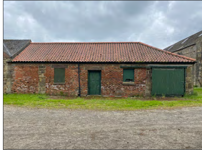
Photo 06. West elevation of the single-storey west range of farm-buildings
