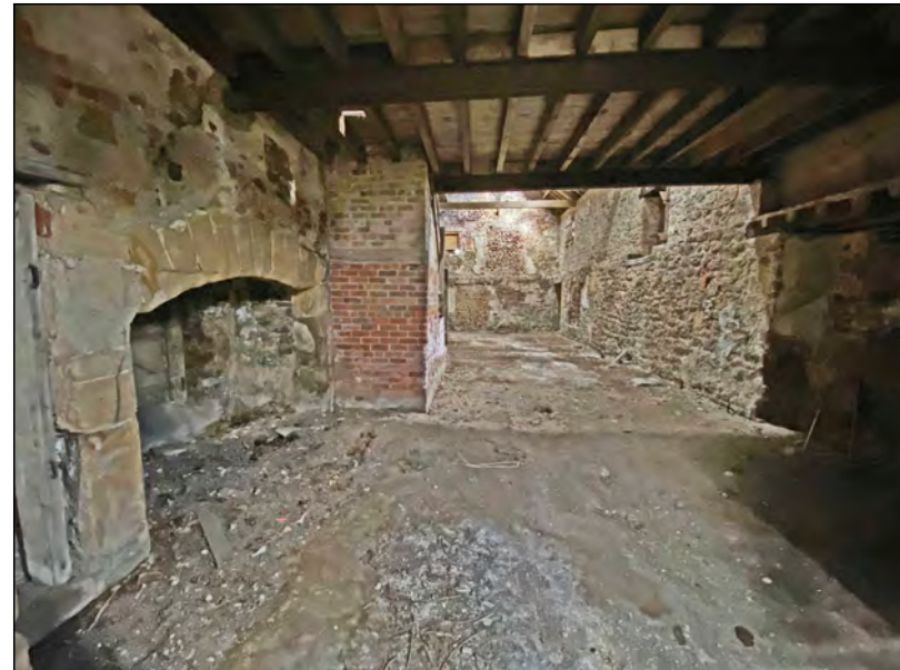
Photo 60. View NNE from the SW corner of the 'Old Hall' at GF level, showing fireplace in the S part of the internal W wall and modern brick-built stair beyond.
