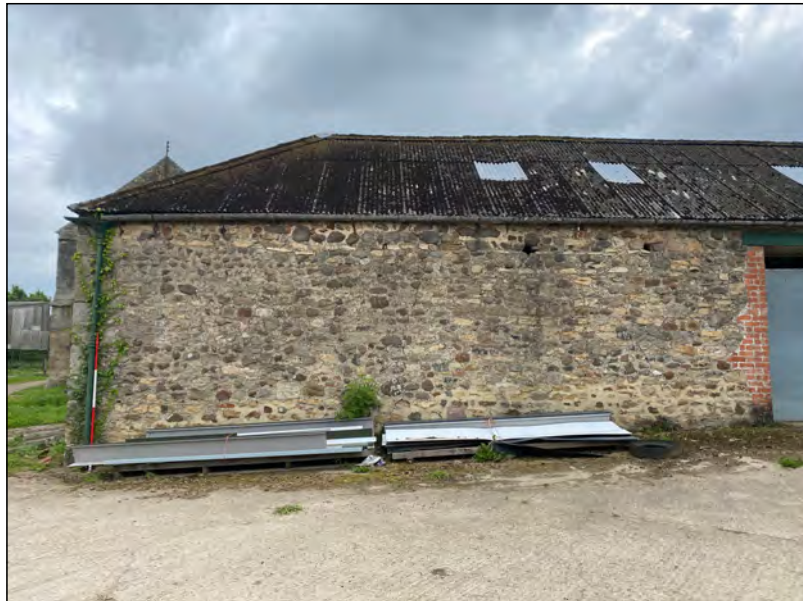
Photo 11. The east part of the north elevation to the north range
