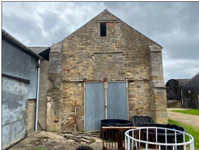
Photo 23. The south elevation of the 'Old Hall'.
