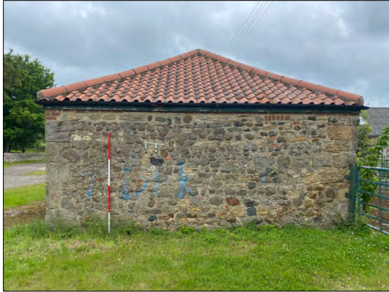
Photo 05. South gable elevation of the single-storey west range of farm-buildings
