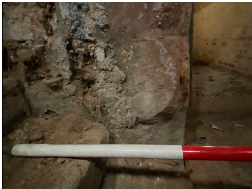
Photo 75. Possible column base now forming part of doorway surround to a passage into a first-floor entrance door at the top of stairs against the W wall.
