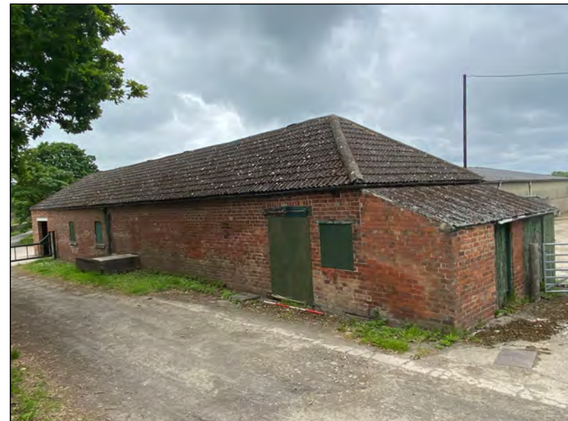
Photo 36. The detached brick-built north-west range viewed from the south-west, showing lean-to southern attachment.
