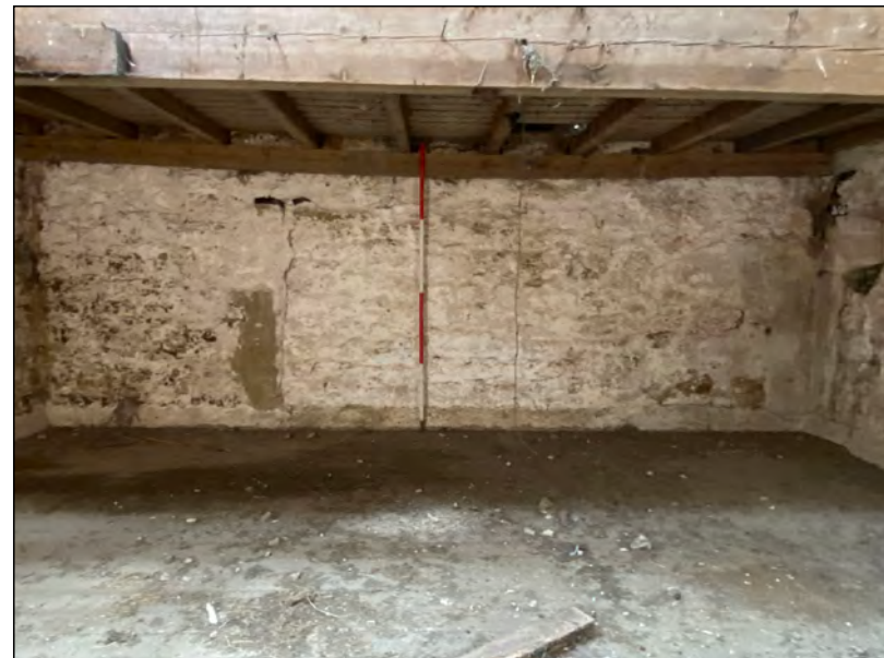
Photo 80. The north-facing internal face of the south wall at first-floor level.
