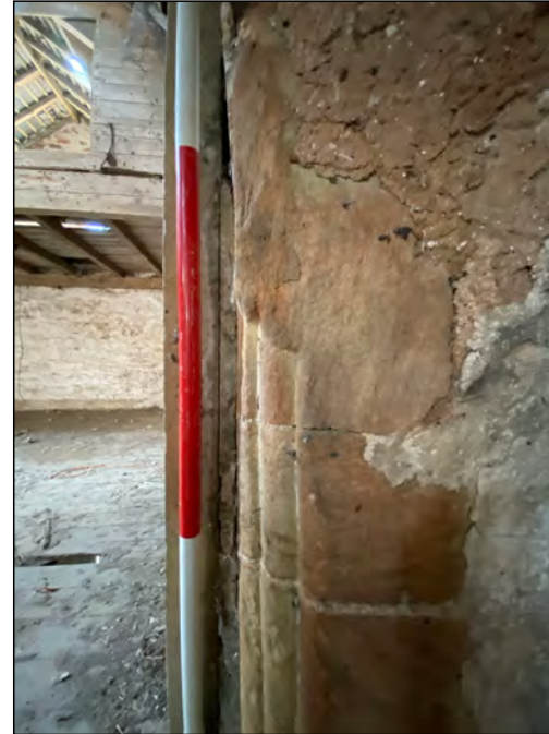
Photo 74. Detail of former fireplace jamb in the west wall, first-floor level.
