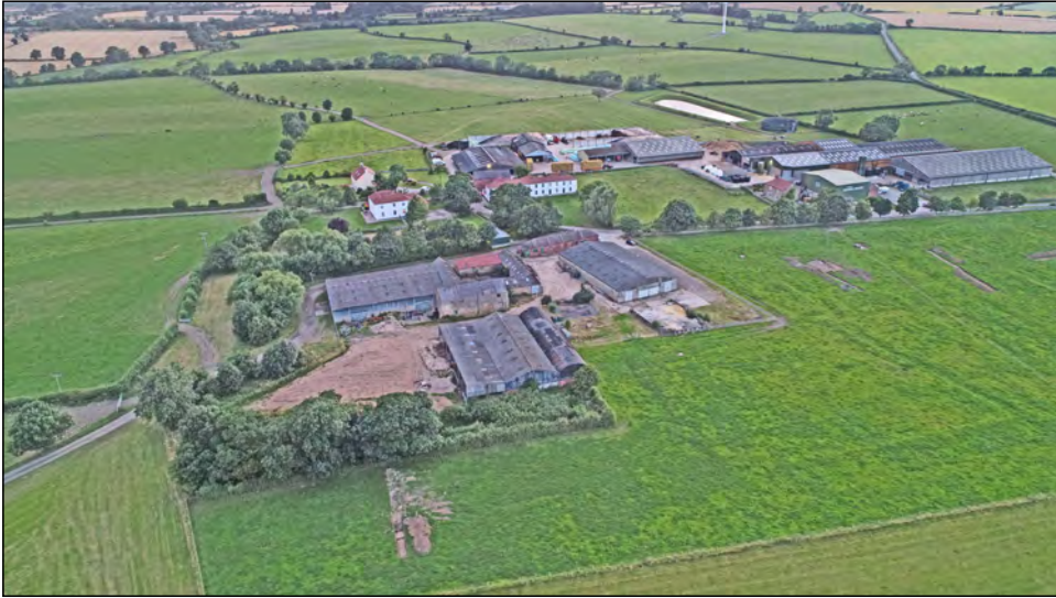
Photo 01. Oblique aerial view of Archdeacon Newton from the south-east, with Hall Farm in the foreground.
