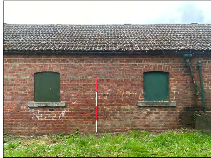
Photo 38. Windows in the central part of the detached, brick-built north-west range.
