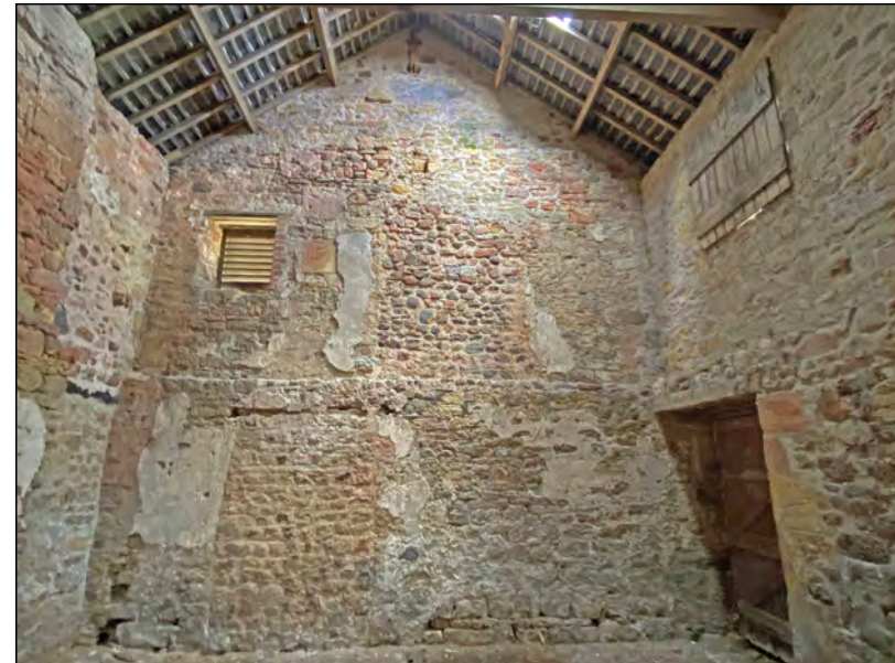
Photo 52. The south face of the north wall of the 'Old Hall'.
