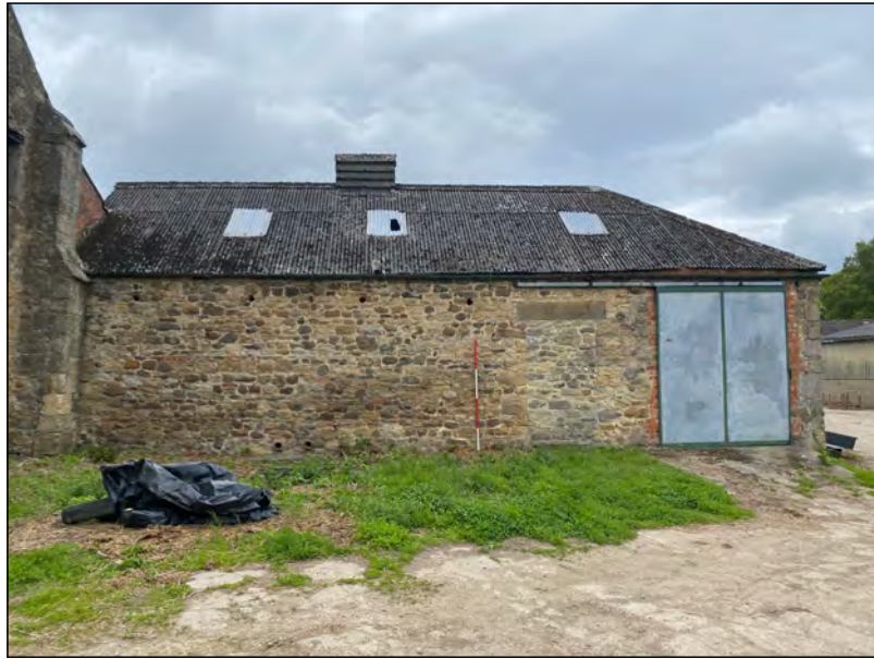
Photo 13. The east elevation of the east range.
