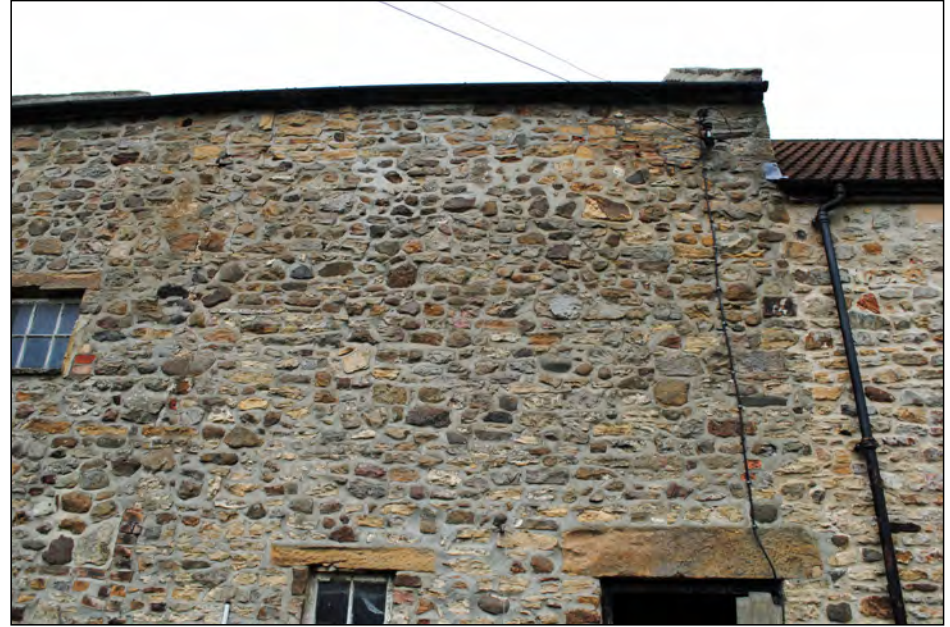
Photo 06. South-east facing elevation (upper right portion) of mill building.
