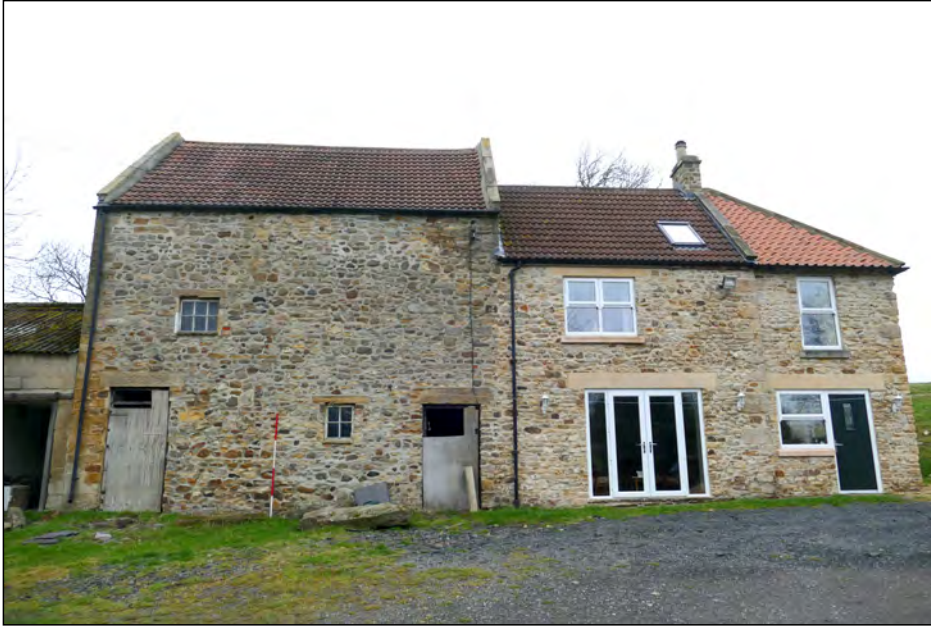
Photo 01. View looking north-west towards Middridge Grange Mill (left) and adjoining cottage (right).
