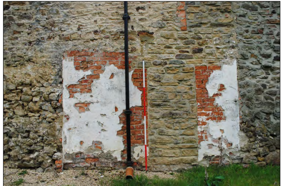
Photo 20. Detail of blocked doorways at the west end of the cottage north wall.
