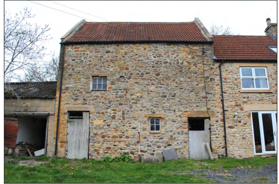
Photo 02. South-east facing elevation of the mill building.
