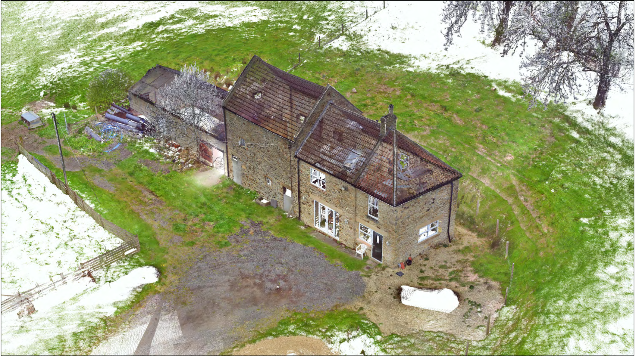
Illus. 15: Digital scan of Middridge Grange Mill, 3D view looking WNW, captured by Gianluca Foschi, April 2022.
