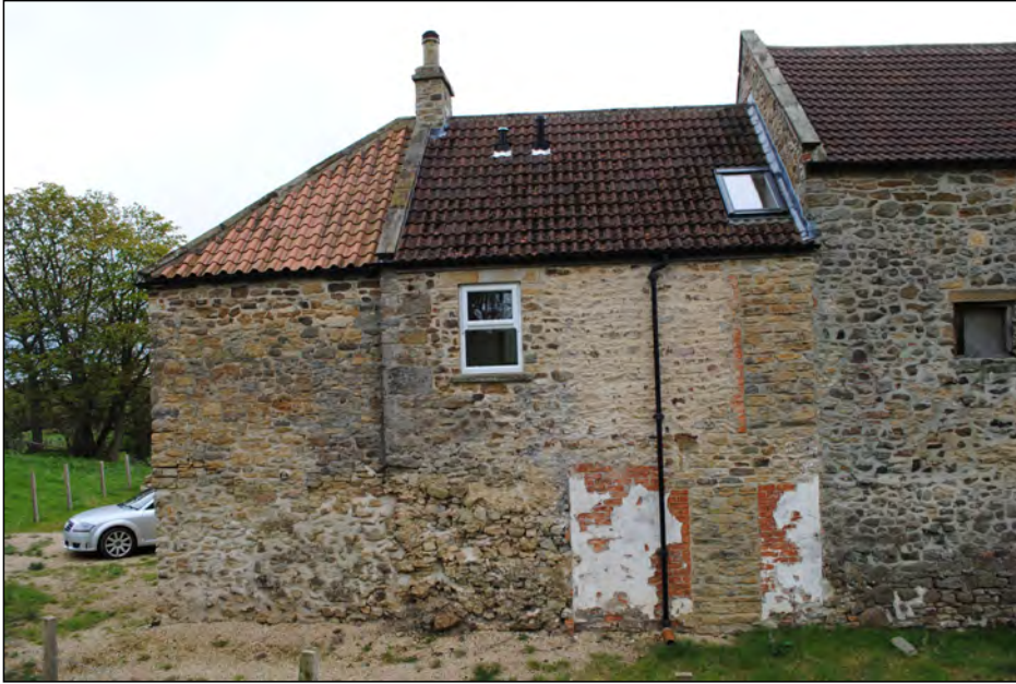
Photo 17. North elevation of cottage adjoining the mill.
