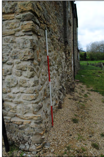
Photo 26. North-east view alongside the north wall of the mill-cottage.
