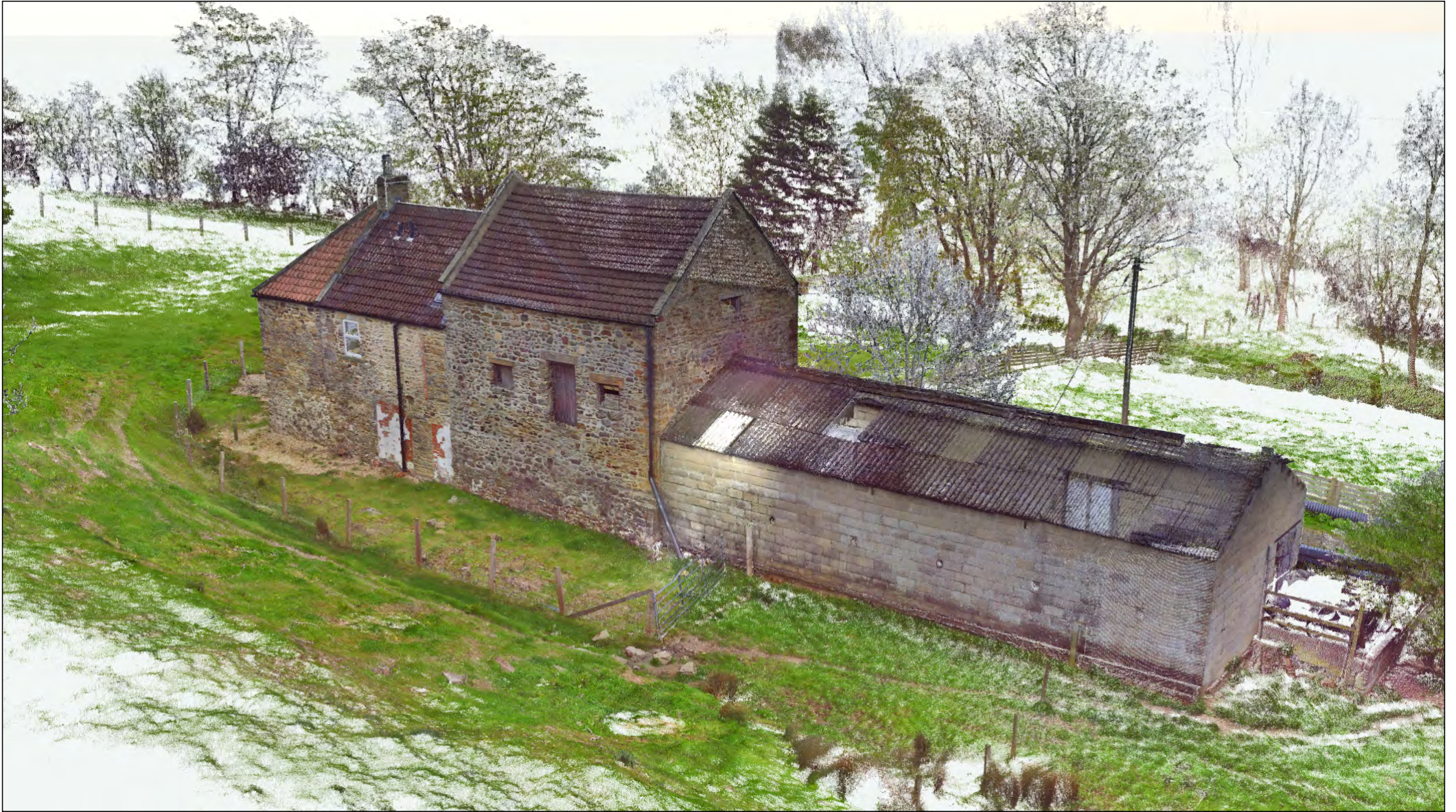
Illus. 16: Digital scan of Middridge Grange Mill, 3D view looking south-east, captured by Gianluca Foschi, April 2022.
