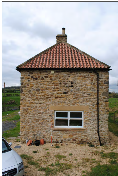
Photo 25. Detail of rough battered masonry in the lower part of the mill-cottage north wall, probably originally footings, exposed after modern landscaping work.
