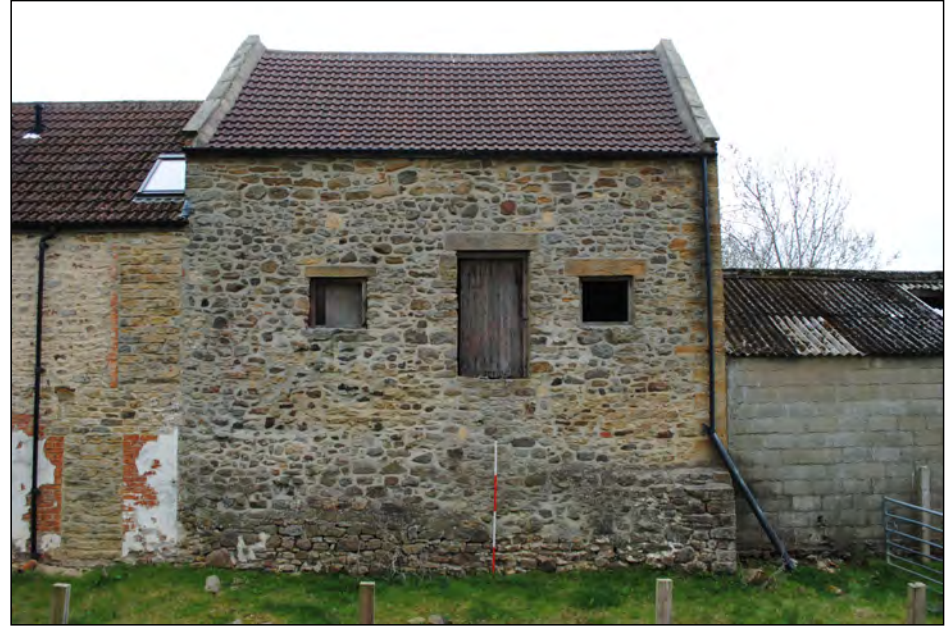
Photo 18. North elevation of mill.
