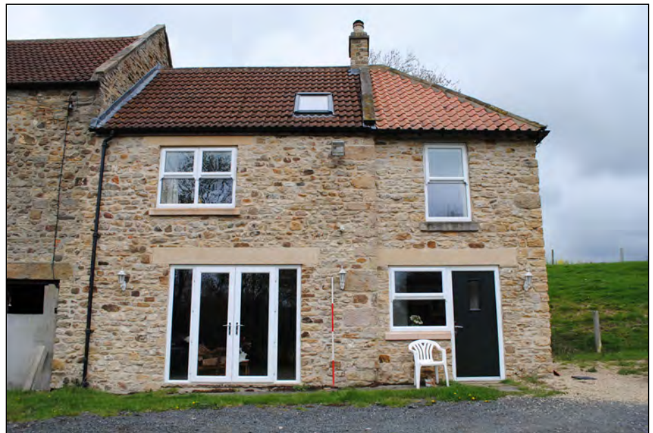
Photo 28. South elevation of the mill-cottage and its east bay extension.
