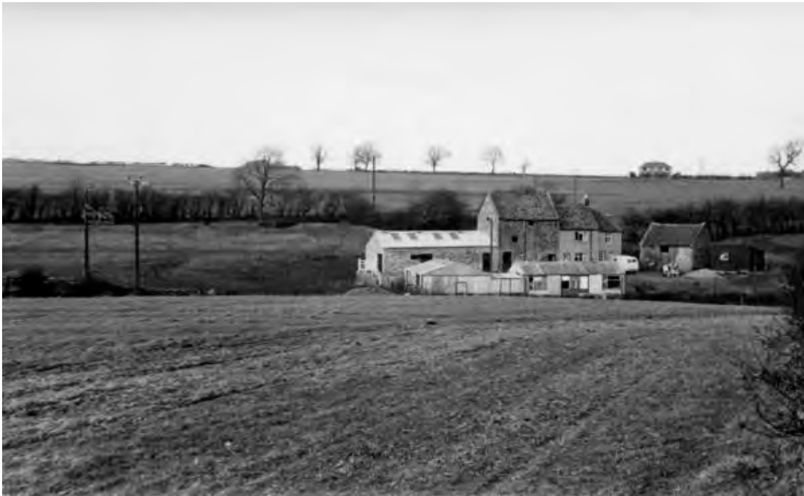
Illus. 17: View looking north-west towards Middridge Grange Mill in 1966.
