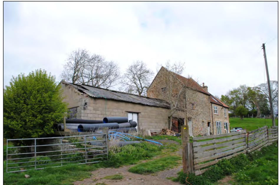
Photo 08. Broad view looking north-east across Middridge Grange Mill.
