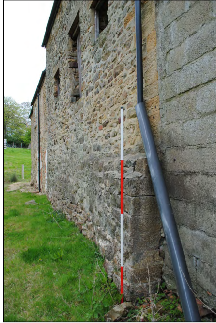
Photo 21. View looking east at projecting tooled-and-margined blocks, a remnant of the east side of the wheel pit, set against the west gable of the mill.
