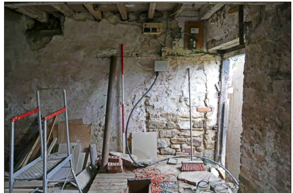
Photo 12. View looking north-east at east wall (interior) of mill.
