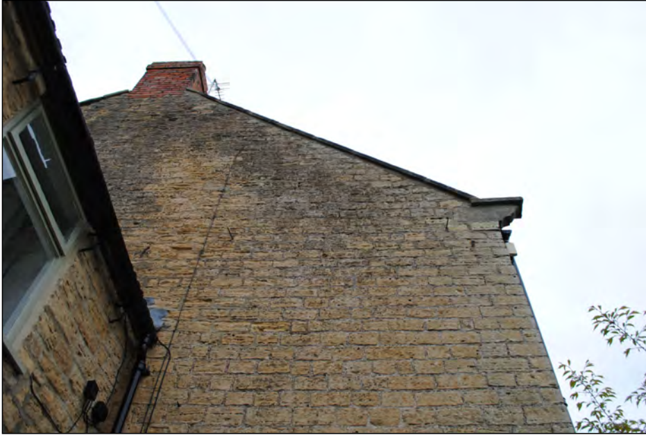
Photo 25. Upper part of north-west facing elevation of farmhouse.
