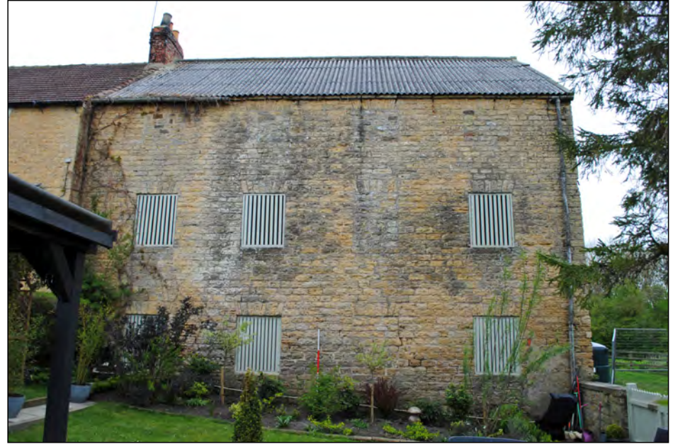
Photo 18. South-west facing elevation of the mill.
