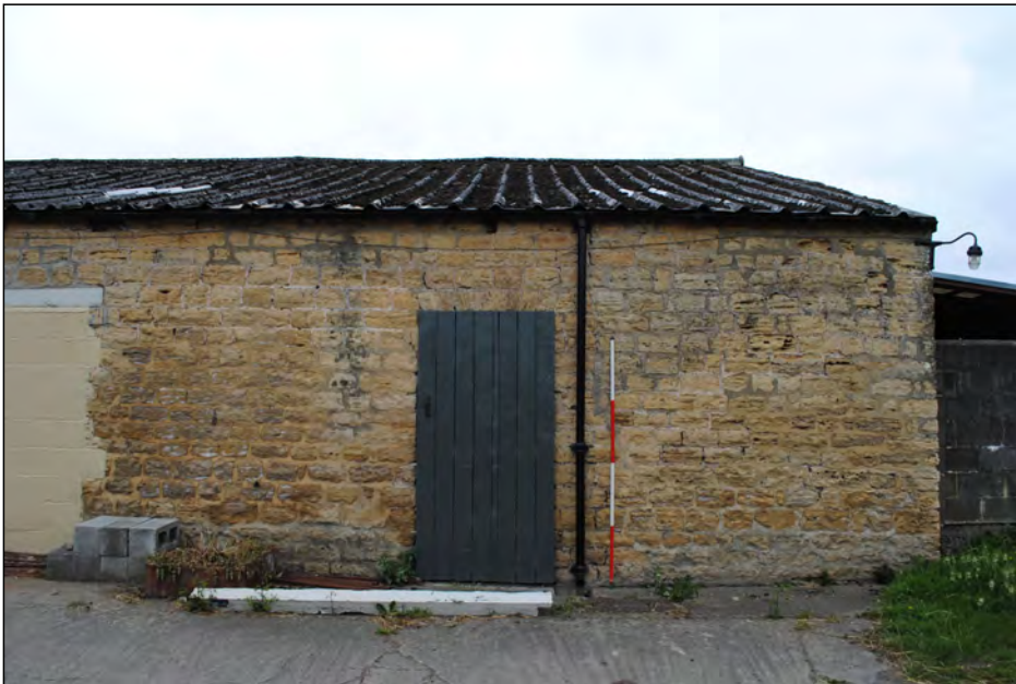
Photo 43. South-east facing elevation of stable block, NE end.
