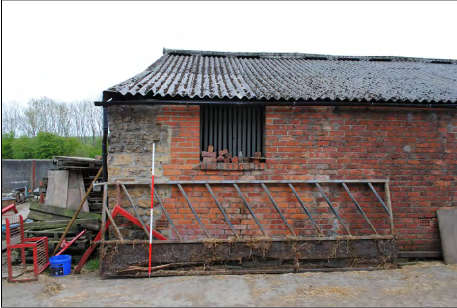
Photo 49. North-west facing elevation of stable-block NE end.
