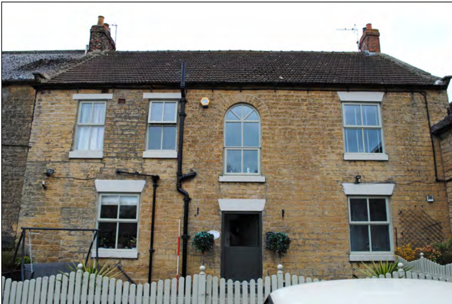
Photo 27. North-east facing elevation of farmhouse.
