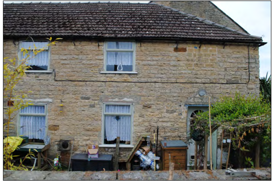
Photo 62. North-west facing elevation of cottage, SW end.
