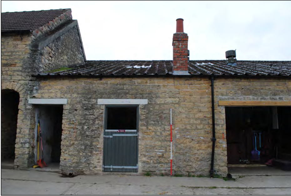
Photo 41. South-east facing elevation of stable block, SW end.
