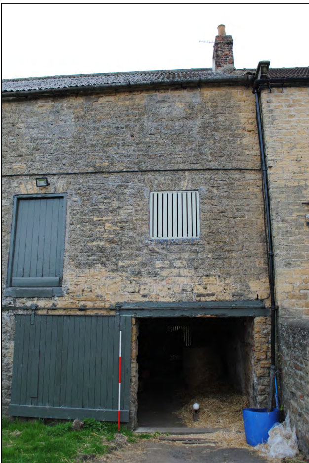
Photo 07. Detail of right portion of mill north-east facing elevation.
