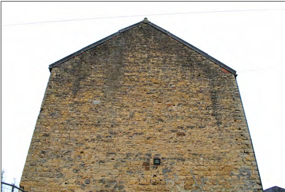
Photo 11. Detail of upper portion of mill south-east facing elevation.
