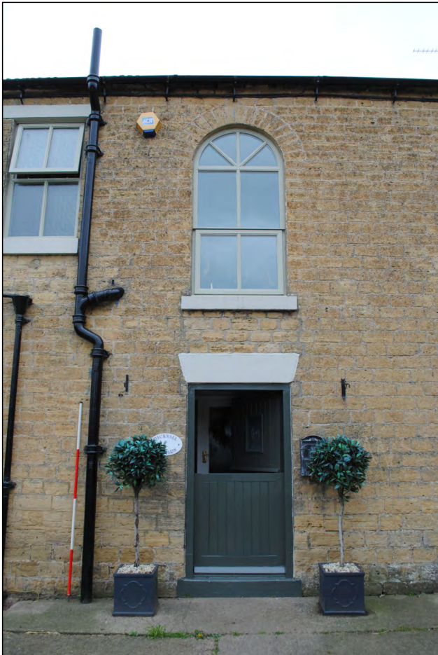
Photo 29. Detail of centre portion of north-east facing elevation of farmhouse.
