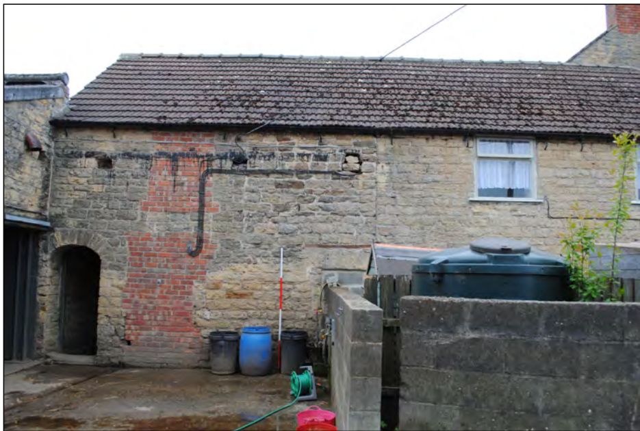
Photo 59. North-west facing elevation of cottage, centre area.
