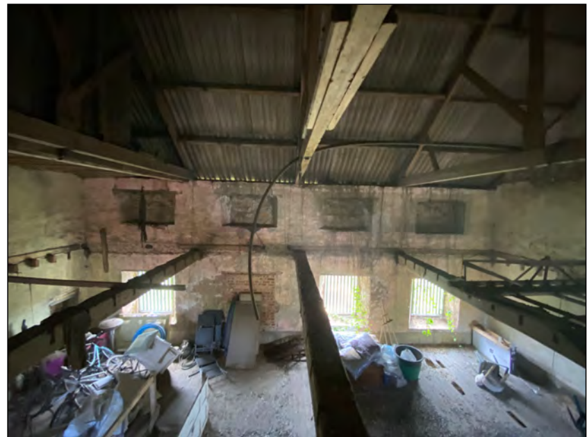
Photo 96. Mill interior, view looking south-west at roof-space and along beams to support former second floor.
