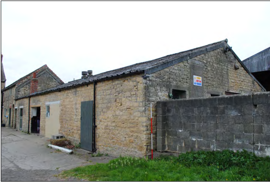
Photo 45. View looking WNW towards the SE corner of the stable block.
