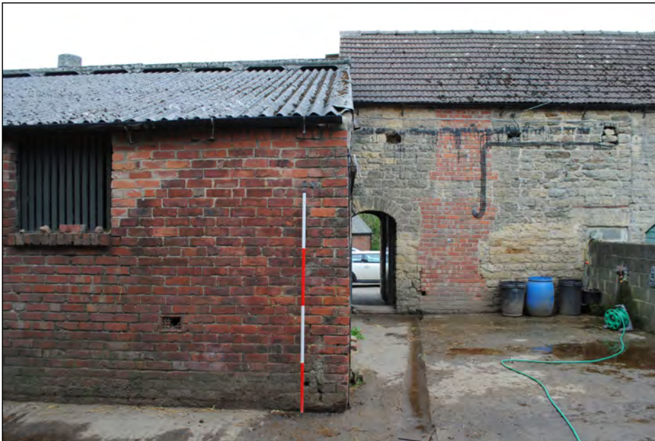
Photo 51. North-west facing elevation of stable-block SW end.
