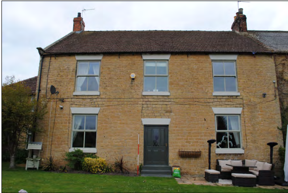
Photo 21. South-west facing elevation of the farmhouse.
