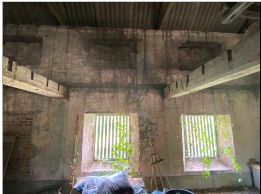
Photo 84. Mill interior (first floor), south-west facing elevation (SE end).
