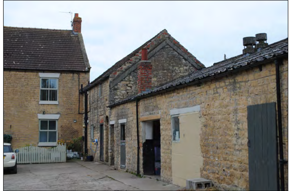
Photo 38. View looking west along SE wall of stable block towards NE gable of cottage, with earlier roof-line of stables? visible.
