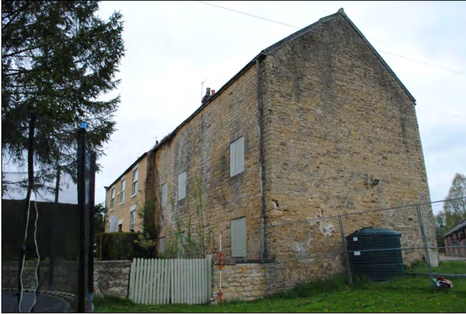
Photo 17. View looking NNE towards the SW corner of the mill.
