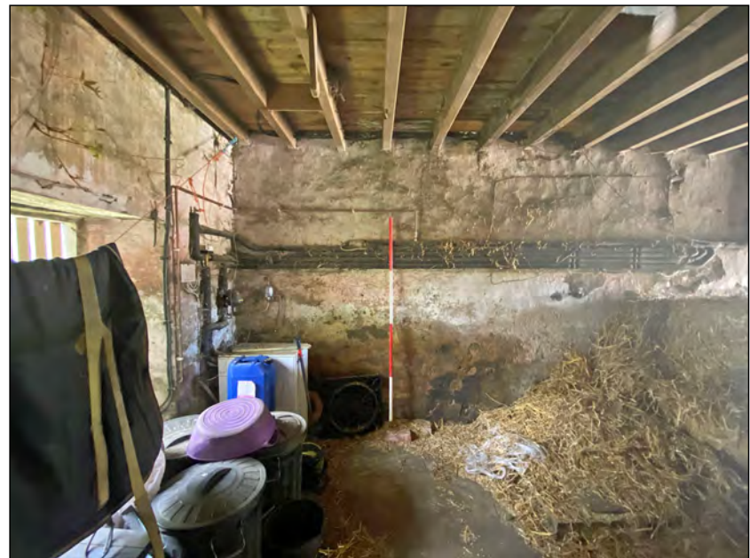
Photo 72. Mill interior (ground floor), south-east facing elevation (SW end).
