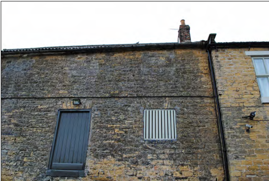
Photo 03. Detail of upper-right portion of mill north-east facing elevation.
