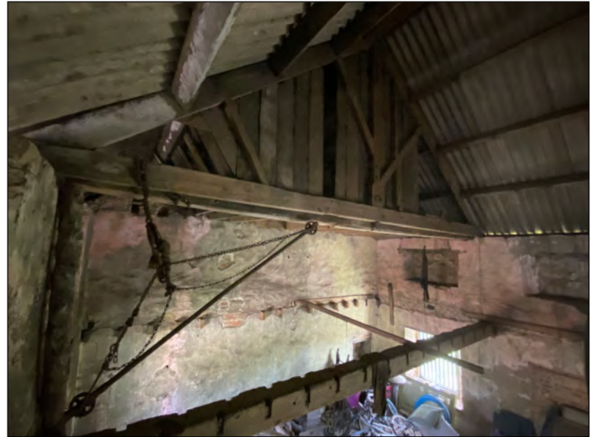
Photo 98. Mill interior, view looking SSW towards the south corner of the former second floor, with hoist mechanism between beams.
