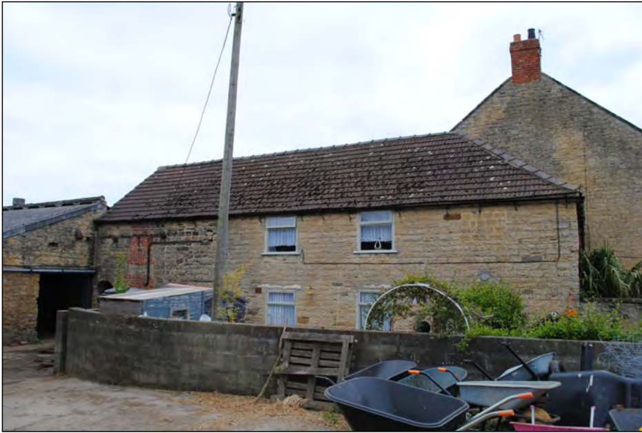
Photo 61. View of cottage looking south-east towards its NW facing elevation.
