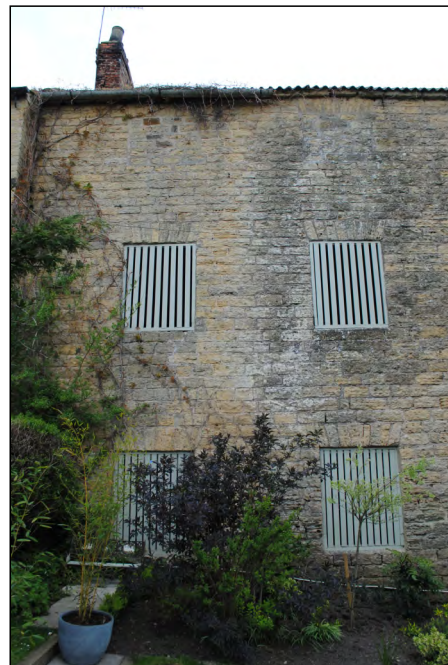
Photo 19. Detail of left portion of south-west facing elevation of the mill.
