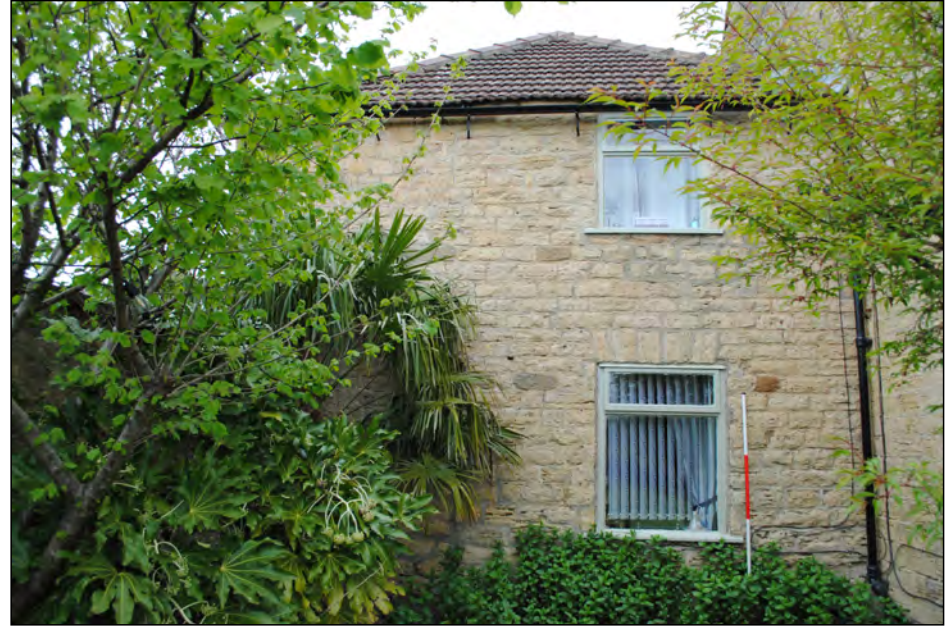
Photo 26. South-west facing elevation of adjoining cottage.
