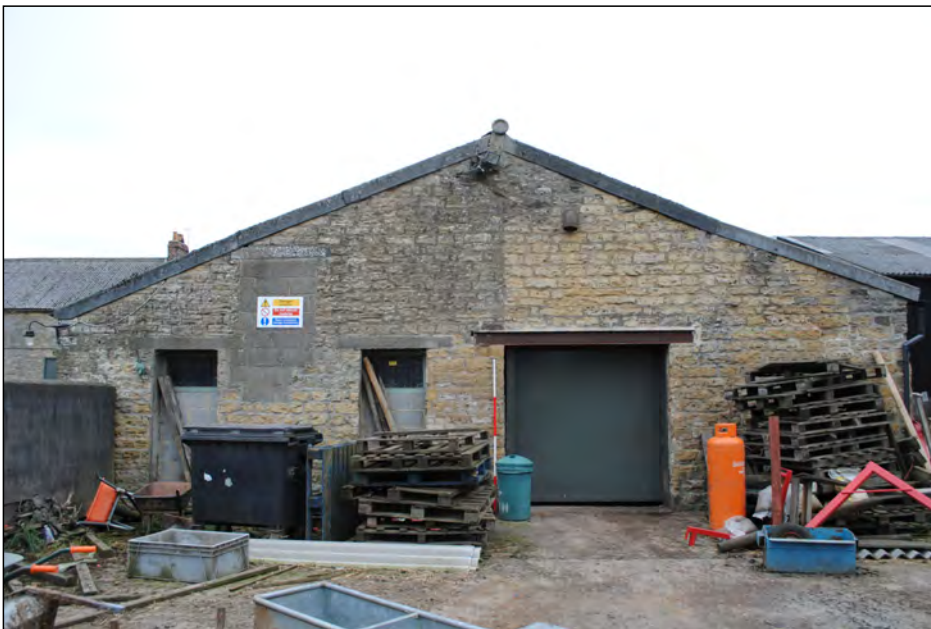
Photo 47. North-east facing elevation of the stable block.
