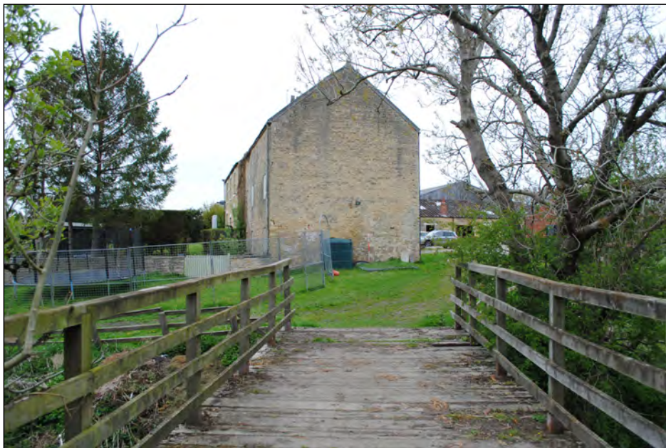
Photo 15. View looking NNW from the footbridge towards the mill.
