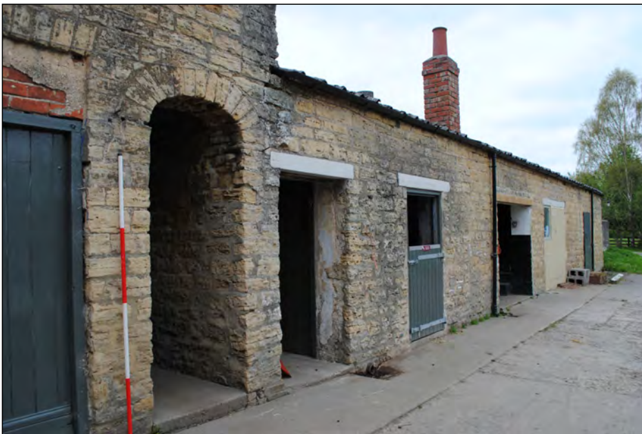
Photo 35. View looking north across passage arch, between cottage and stables.
