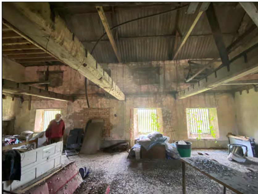
Photo 83. Mill interior (first floor), south-west facing elevation (broad).
