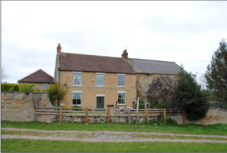
Photo 65. Broad view looking approximately east towards the farmhouse.
