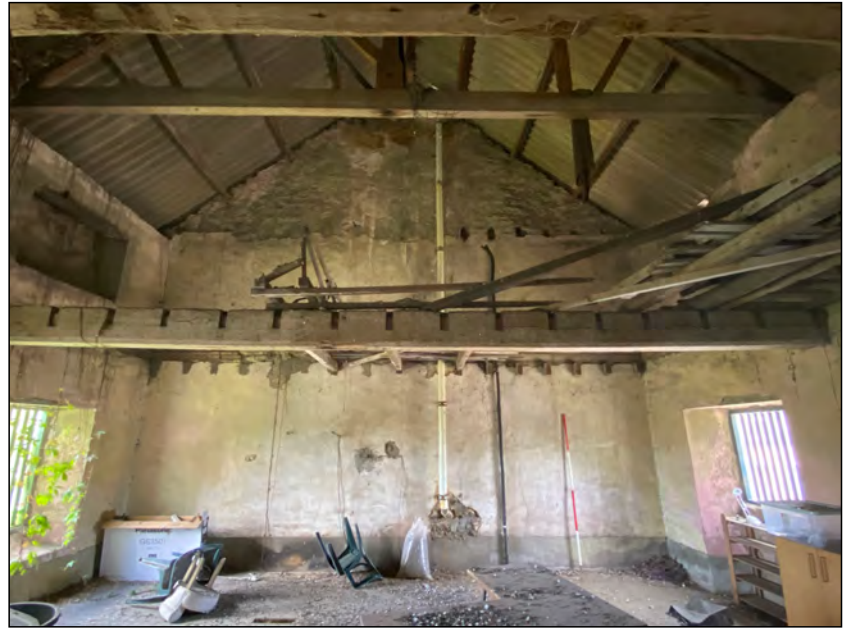
Photo 82. Mill interior (first floor), south-east facing elevation.
