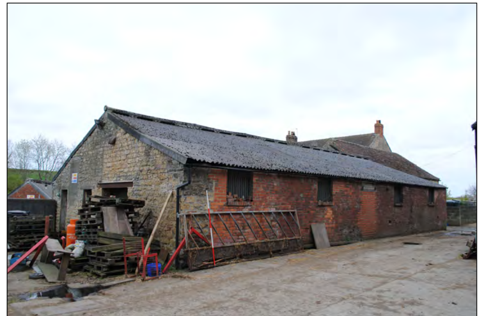
Photo 48. View looking SSW across the NW wall of the stable block.
