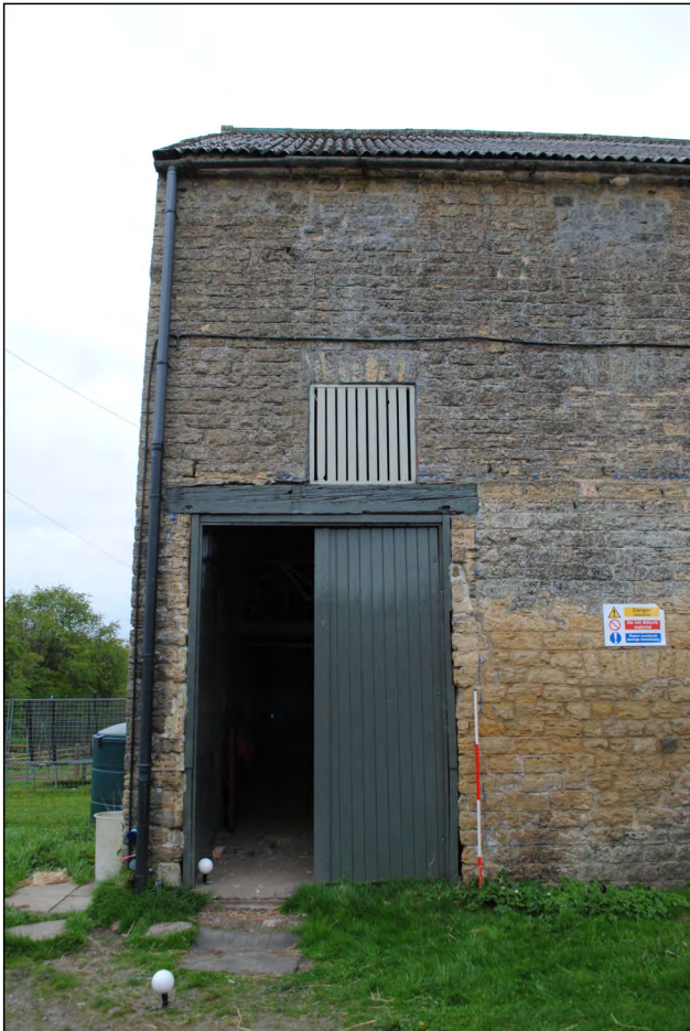
Photo 05. Detail of left portion of mill north-east facing elevation.
