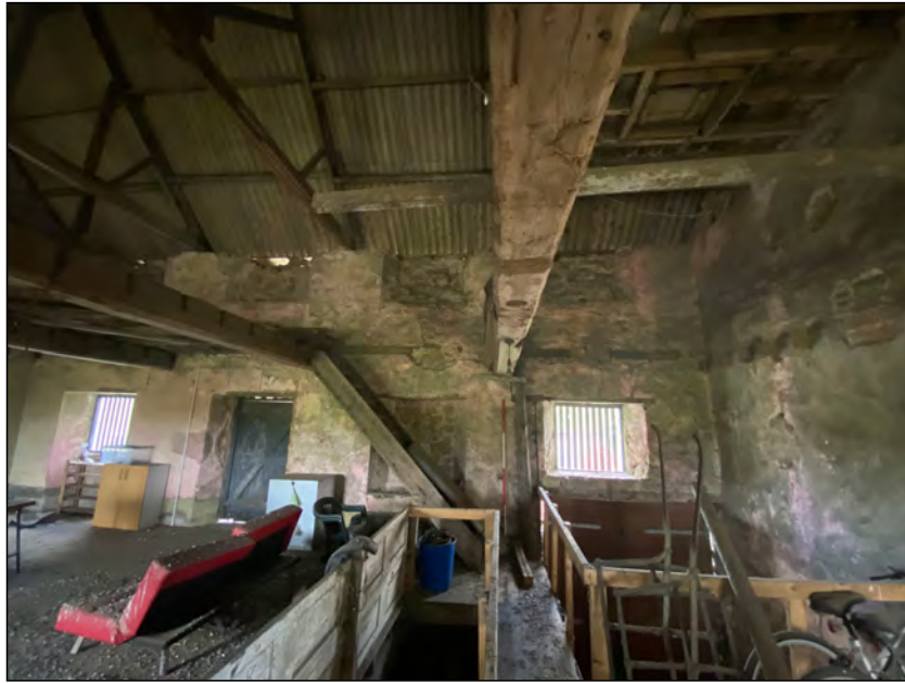
Photo 89. Mill interior (first floor), south-west facing elevation (SE end).
