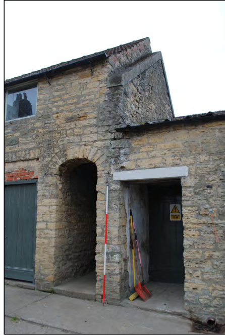
Photo 37. View looking north-west towards passage arch between cottage and stables, with NE gable of cottage and earlier roof-line of stables? visible.
