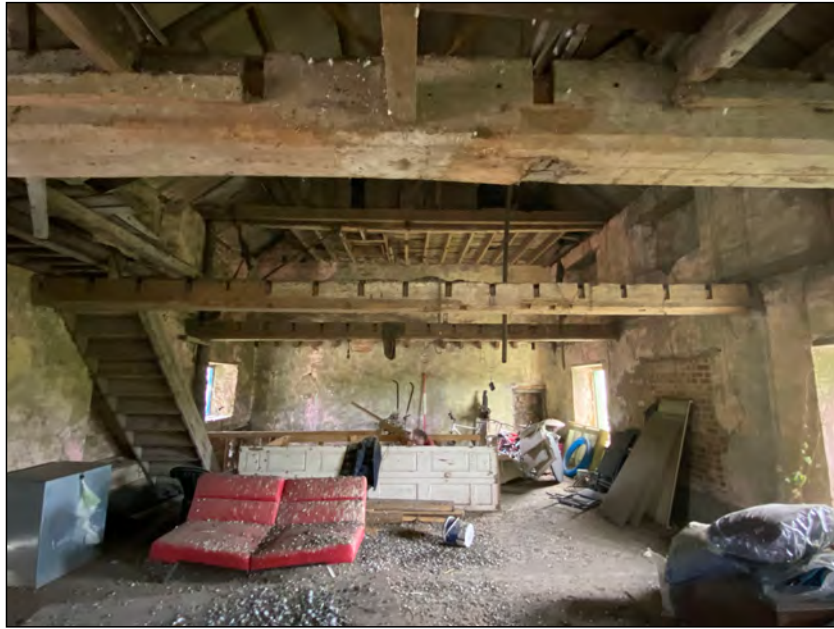
Photo 85. Mill interior (first floor), view looking south-east.
