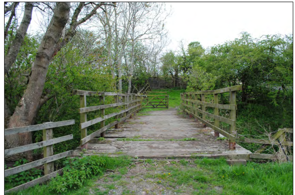
Photo 16. View looking SSE towards the footbridge, south of Ricknall Mill Farm.
