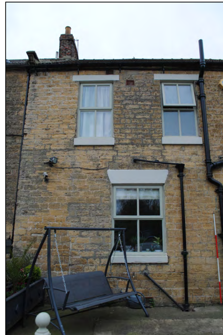
Photo 28. Detail of left portion of north-east facing elevation of farmhouse.
