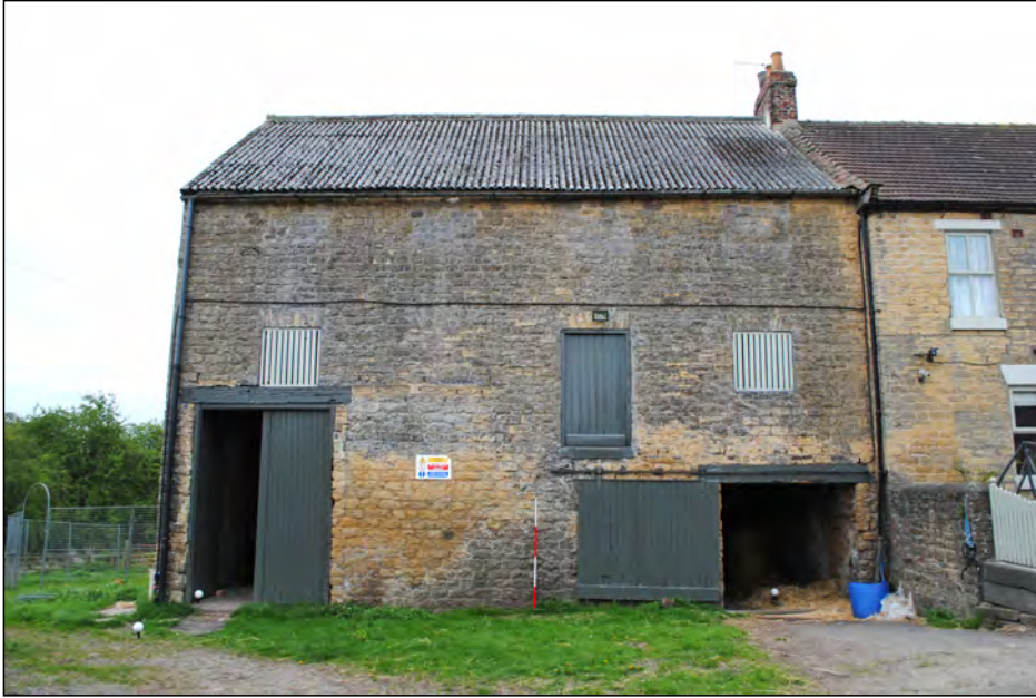
Photo 01. North-east facing elevation of the mill.
