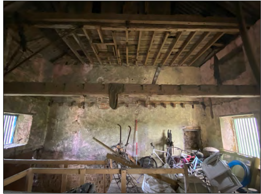
Photo 86. Mill interior (first floor), north-west facing elevation.
