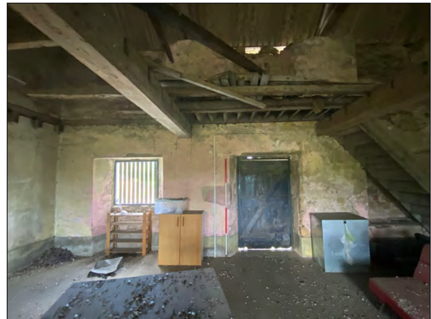
Photo 92. Mill interior (first floor), south-west facing elevation (NW end).
