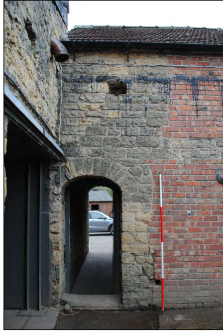
Photo 57. North-west facing elevation of passage arch between cottage and stables.
