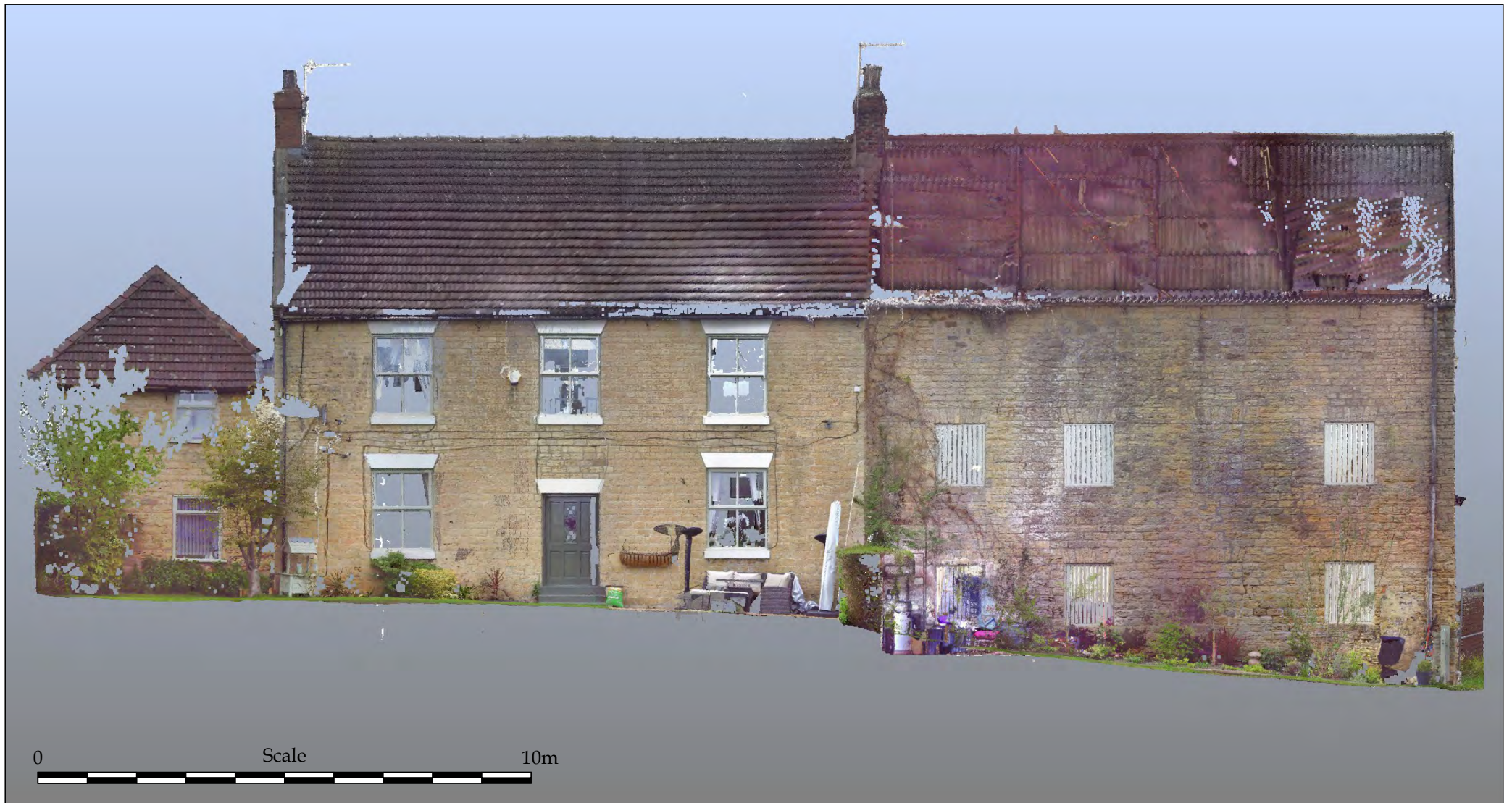
Illus. 10: Digital scan showing south-west facing elevation of Mill, Farmhouse and adjoining cottage at Ricknall Mill Farm.
