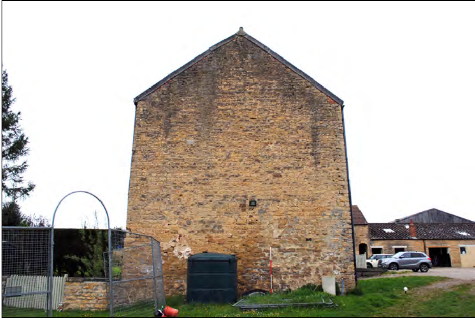
Photo 09. South-east facing elevation of mill SE-gable.
