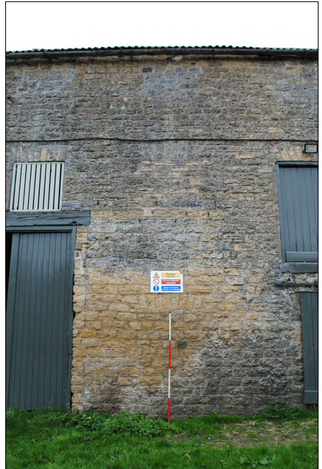
Photo 06. Detail of centre portion of mill north-east facing elevation.
