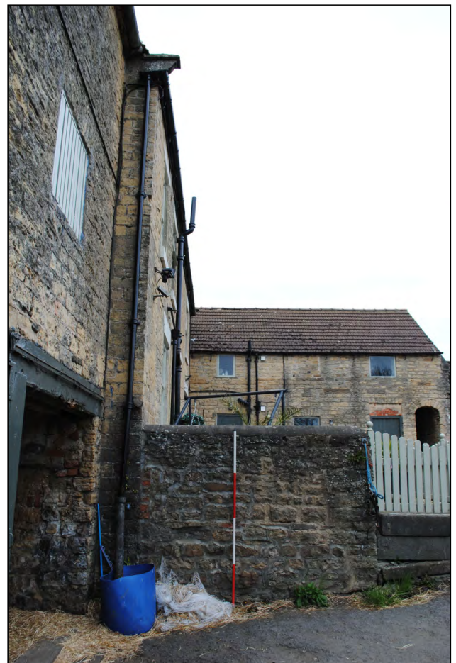
Photo 08. View looking NW at yard boundary wall extending NE from the SE corner of the farmhouse.
