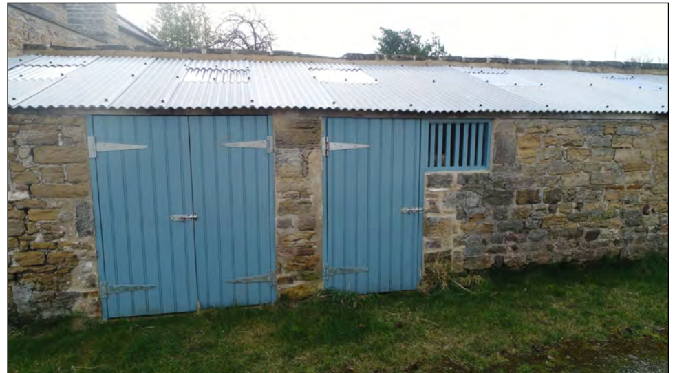
Photo 44. North facing elevation of the central-east end of the outbuilding range.
