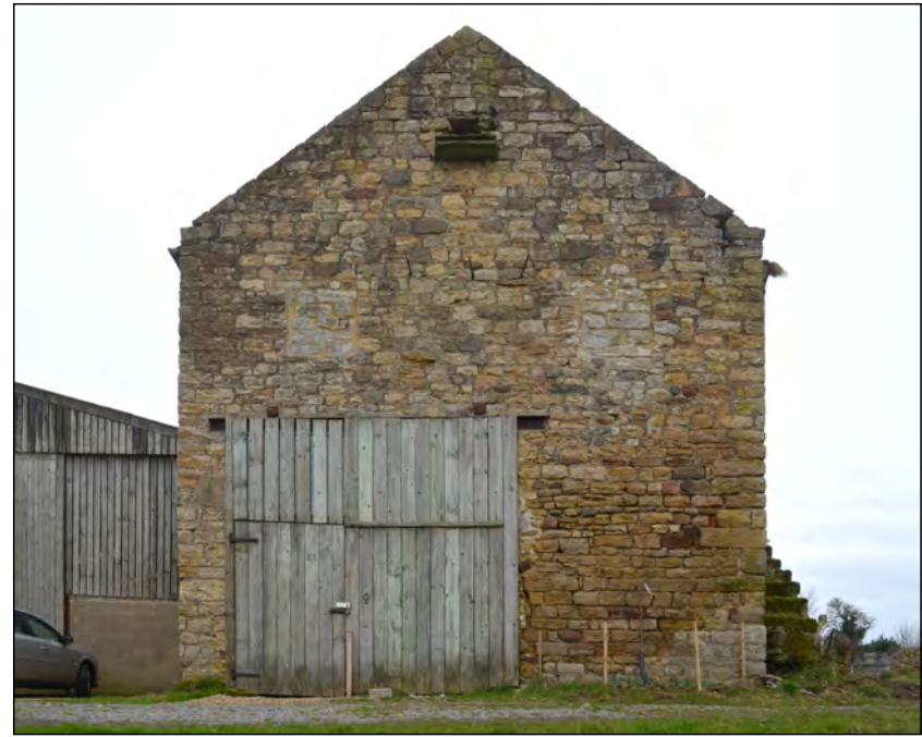
Photo 22. View looking west in February 2020, at the east gable of the Eastern Building in the north range, prior to renovation work.
