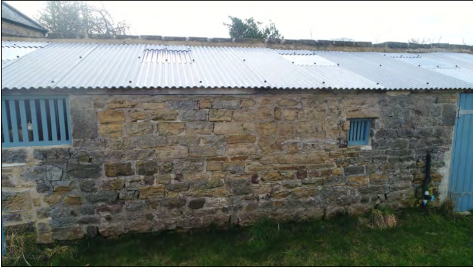
Photo 45. North facing elevation of the central portion of the outbuilding range.
