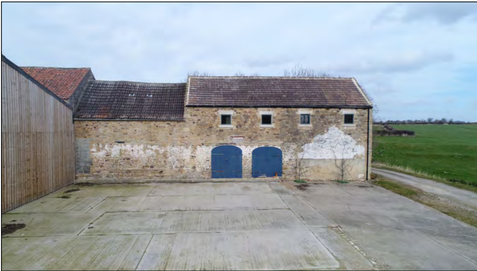
Photo 51. View looking north towards the south wall of the Eastern and Central Buildings in the North Range, with the east gable-end of the former medieval chapel just visible to the left (pantile roof).
