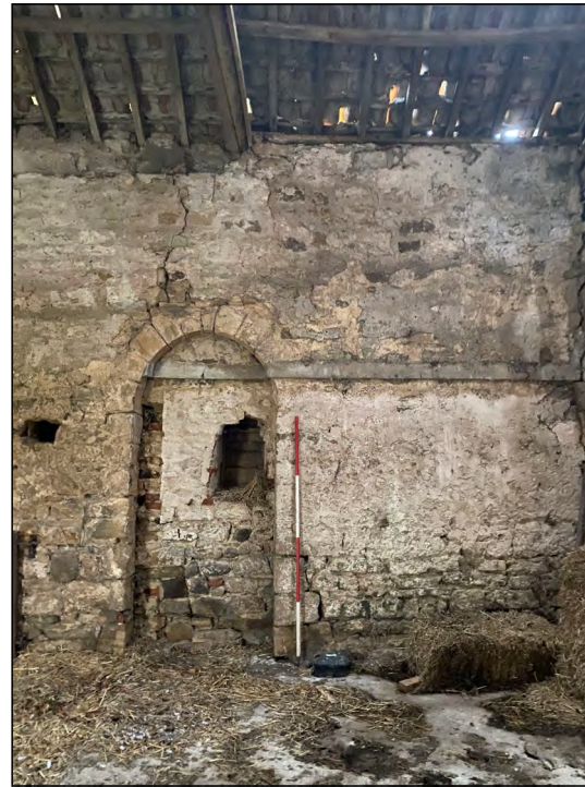
Photo 42. View looking south towards the SW corner of the former medieval chapel, with original doorway (blocked) in the south wall (internal view).
