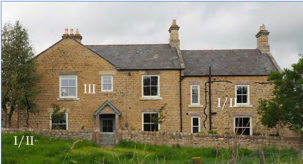
Illus. 35: Annotated photograph of the farmhouse from the south, showing provisional phasing.
