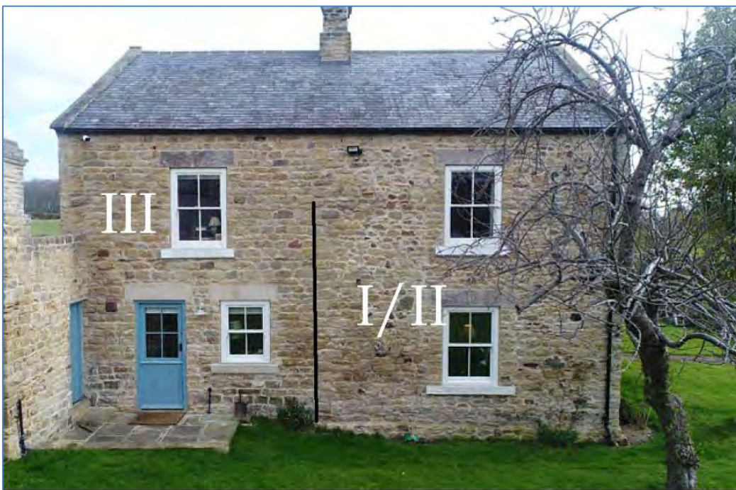
Illus. 36: Annotated photograph of the farmhouse from the west, showing provisional phasing.
