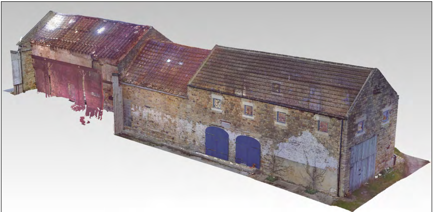
Illus. 25: Digital 3D Scan of the North Range, Walworth North Farm, viewed from the south-east, by Gianluca Foschi, April 2022.
