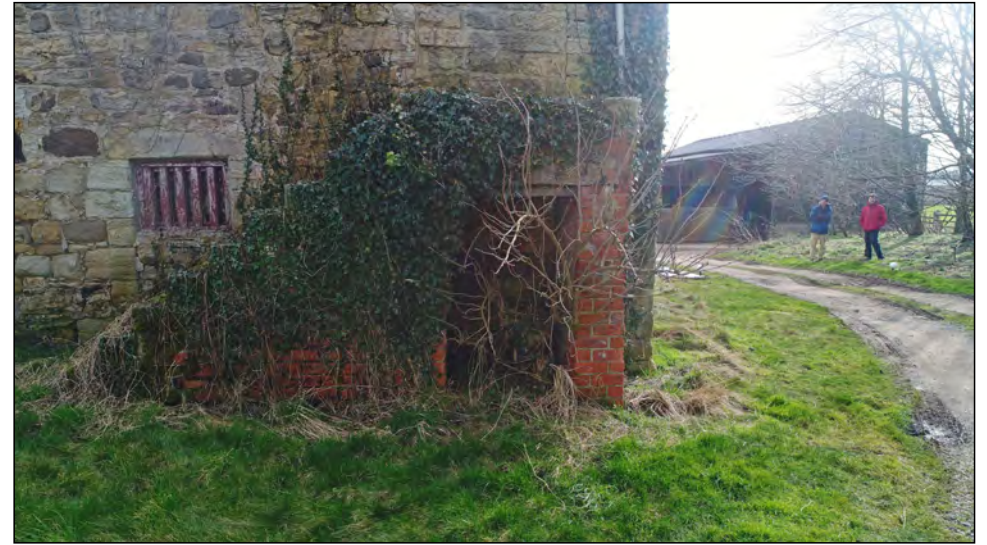
Photo 18. View looking south at an external stair (orange brick with stone steps) located at the west end of the former medieval chapel north wall.
