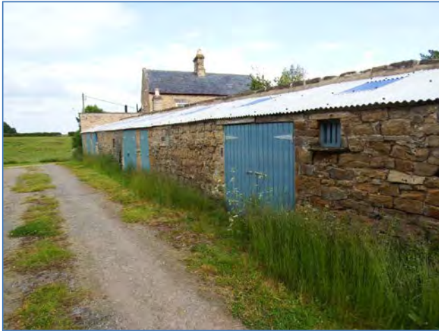
Illus. 39: The outbuilding range looking east, with the farmhouse beyond.
