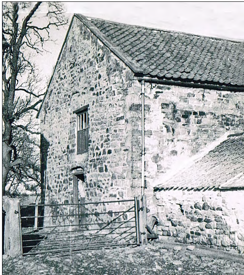
Illus. 09: South-west view of Walworth North Farm Medieval Chapel c.1963, showing the west end before its door and window were replaced by the present cart entrance.
