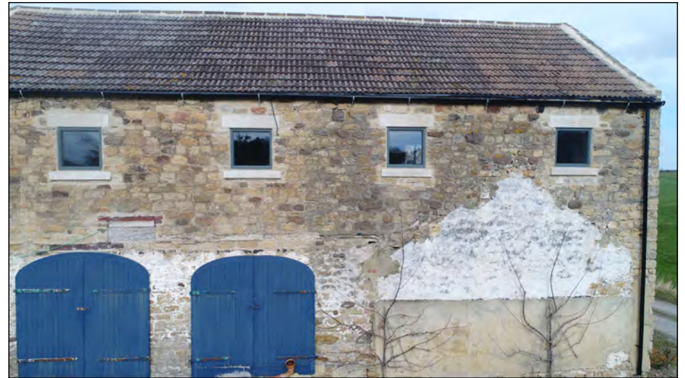
Photo 52. South facing elevation of the Eastern Building of the North Range.
