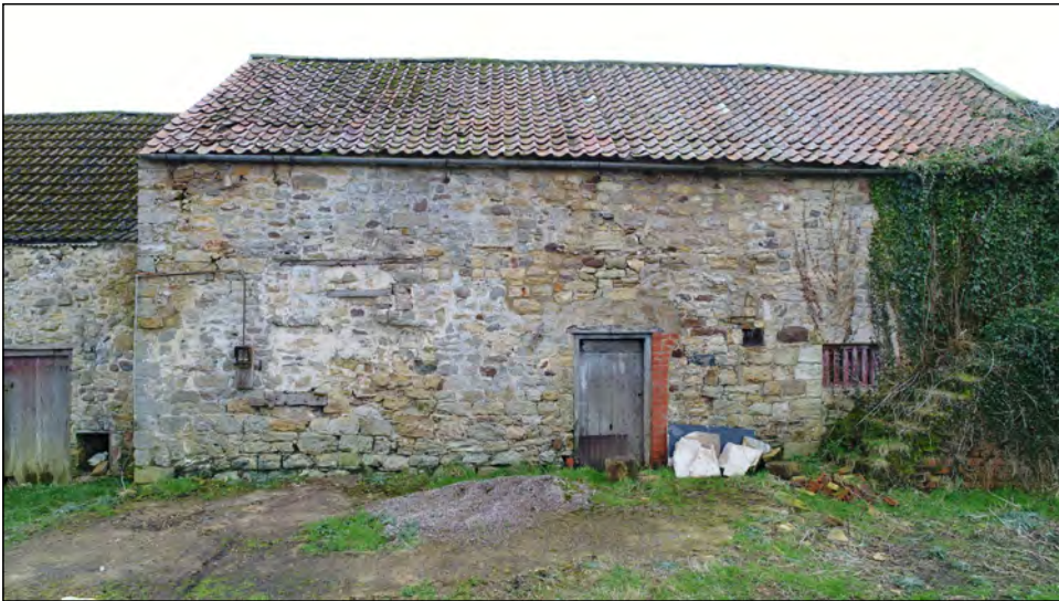
Photo 15. View looking south towards the north elevation of the former medieval chapel in the north range.
