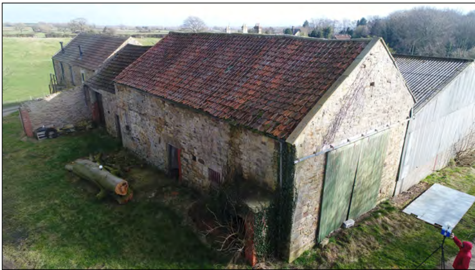
Photo 11. Oblique aerial view, looking south-east across the former medieval chapel.
