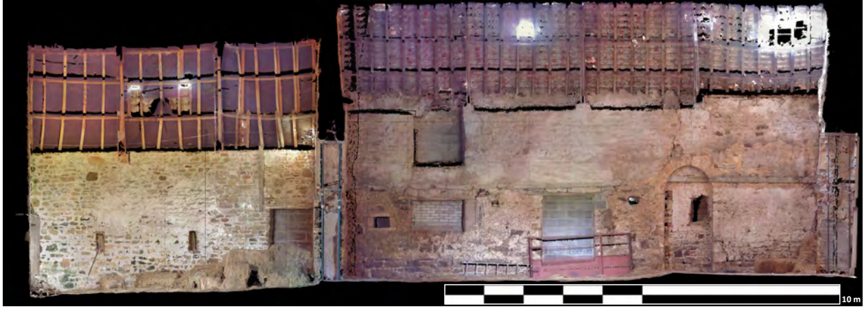
Illus. 15: Digital Scan of the internal south elevation of the Medieval Chapel (right) and Central Barn (left) forming the west side of the North Range, Walworth North Farm, by Gianluca Foschi, April 2022.
