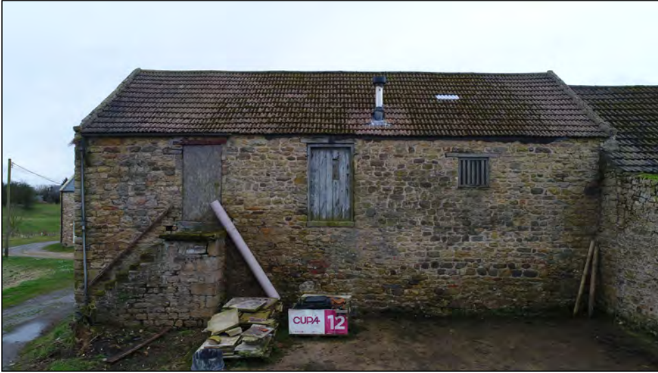
Photo 13. View looking south towards the north elevation of the Eastern Building in the north range.
