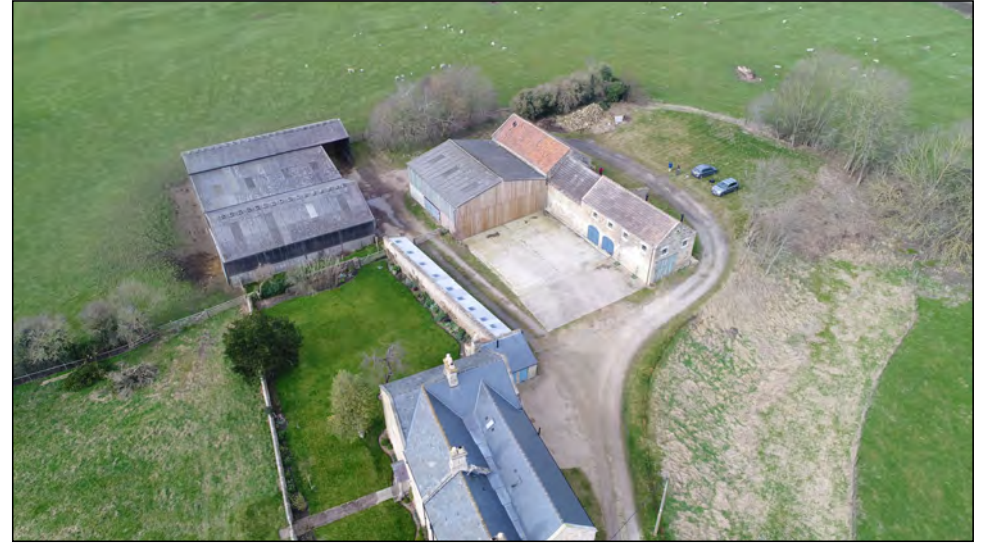
Photo 02. Oblique aerial view, looking north-west across the North Farm complex.
