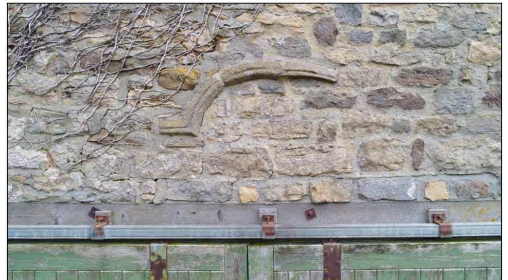
Photo 20. Detail of stones from the hoodmould of a small 12th-century window, visible above the cart-entrance in the west gable of the former medieval chapel.
