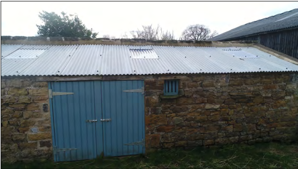
Photo 47. North facing elevation of the west end of the outbuilding range.
