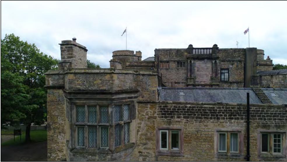
Photo 77. North facing exterior elevation, east end of North Range, upper part of first floor and roof, with Renaissance facade visible in background.
