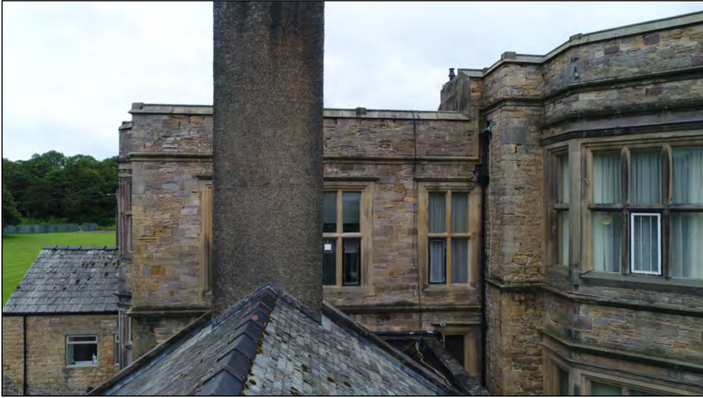
Photo 03. West facing exterior elevation, north end, first floor.
