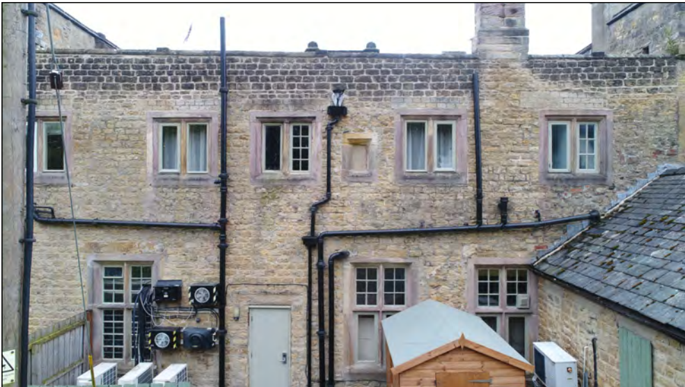
Photo 79. North facing exterior elevation, centre of North Range, first floor.
