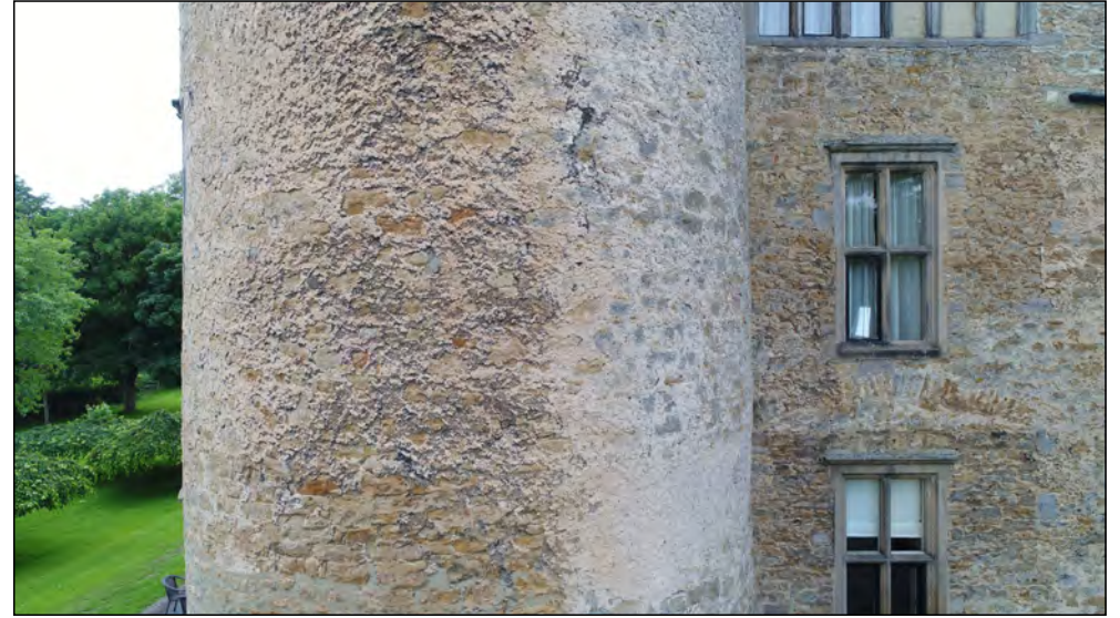
Photo 50. East facing exterior elevation of SE-tower, first floor.
