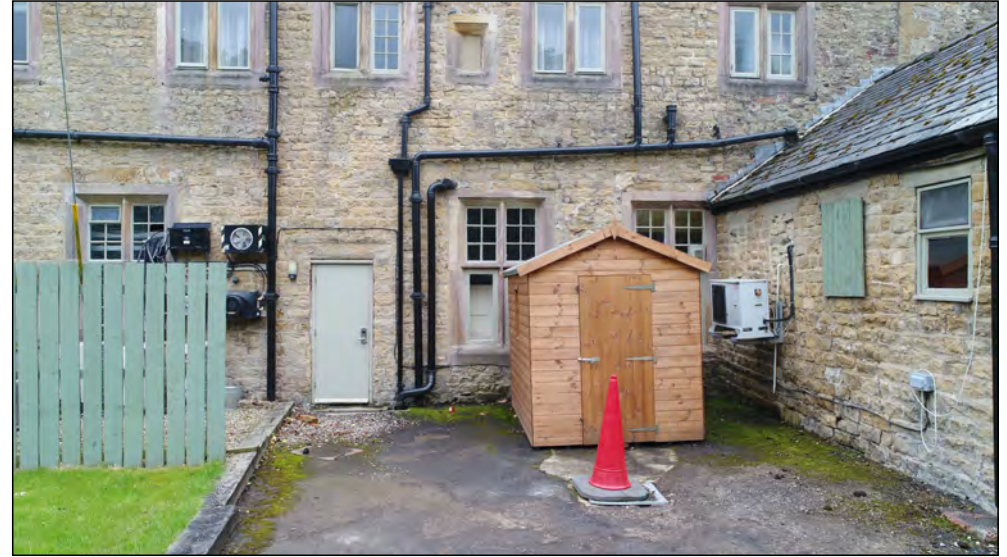
Photo 78. North facing exterior elevation, centre of North Range, ground floor.
