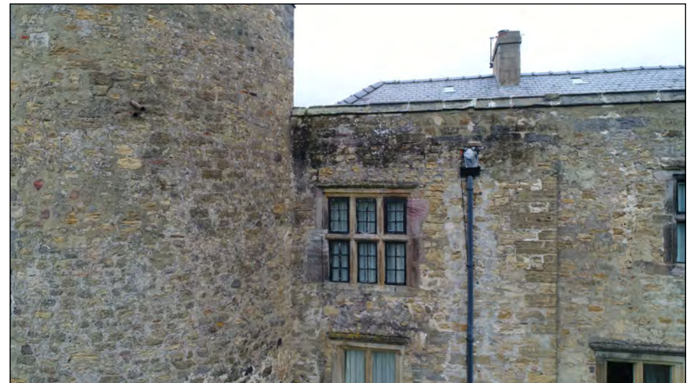
Photo 26. South facing elevation, west end of former manor house, second floor.
