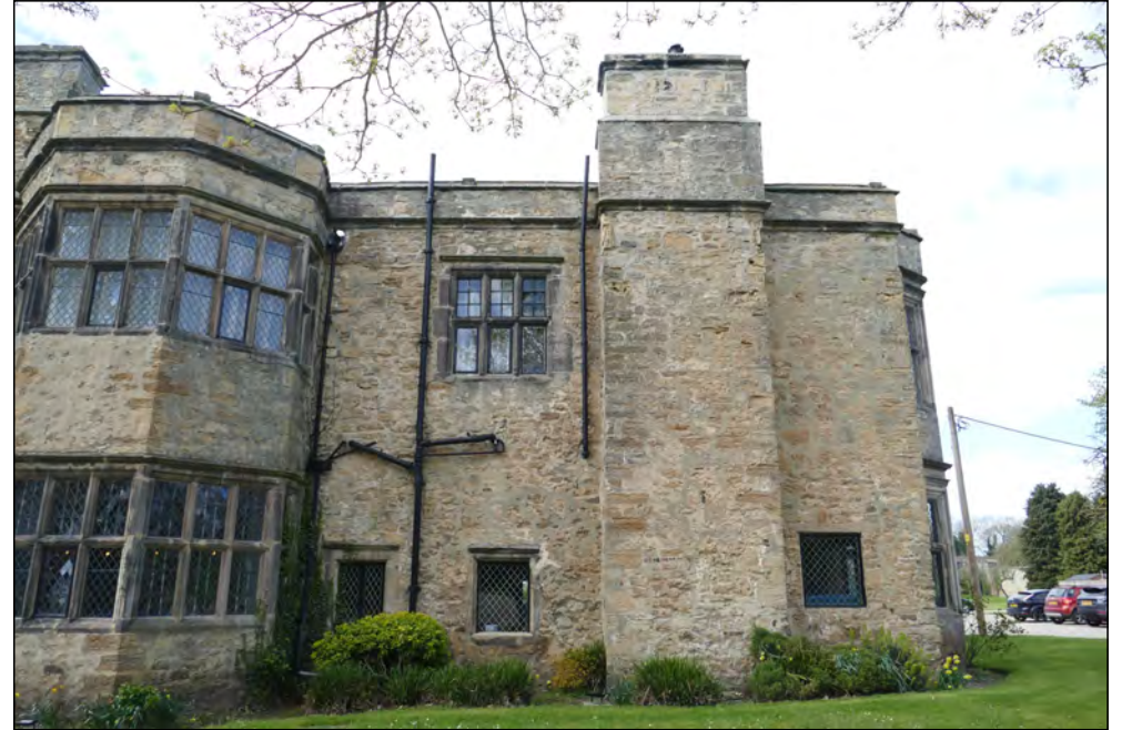
Photo 62. East facing exterior elevation of East Range, north end.
