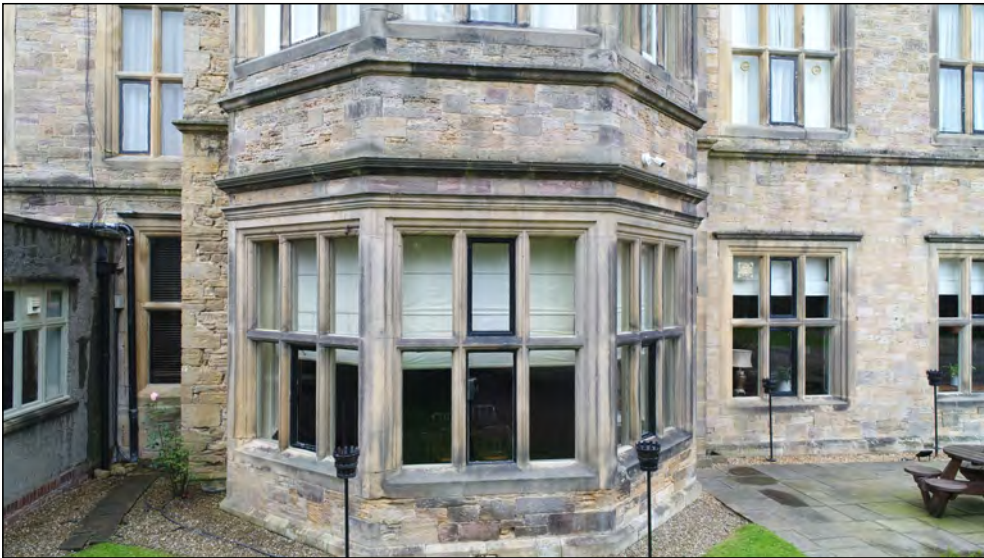
Photo 05. West facing exterior elevation, bay window, ground floor.
