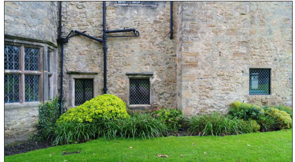
Photo 68. East facing exterior elevation, centre-north of East Range, ground floor.
