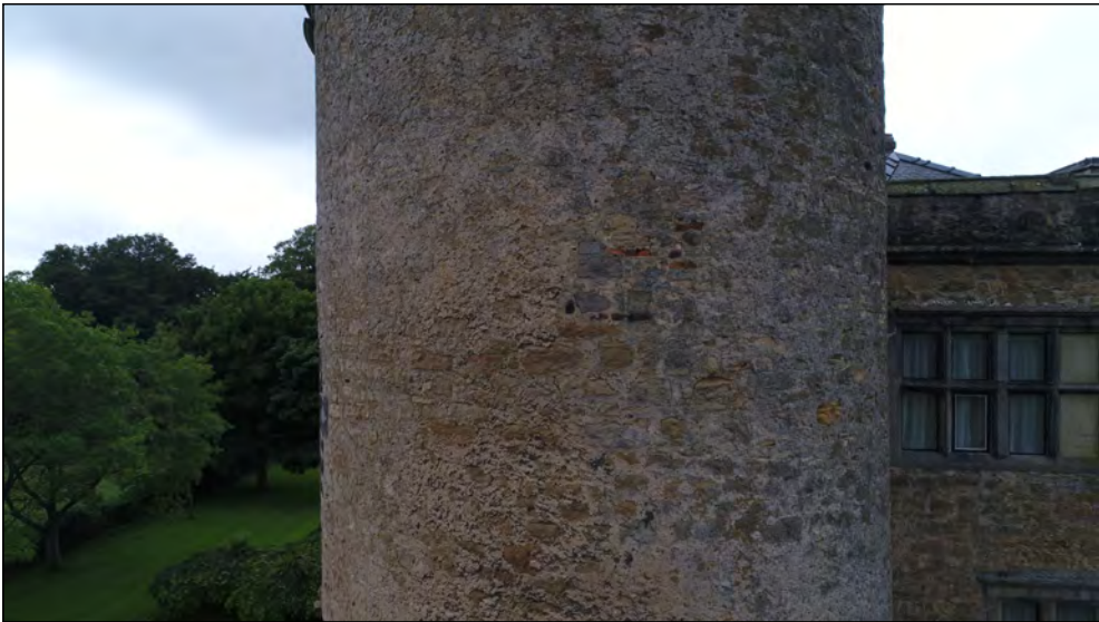
Photo 51. East facing exterior elevation of SE-tower, second floor.
