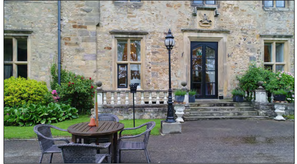
Photo 28. South facing elevation, centre-west part of former manor house, ground floor.
