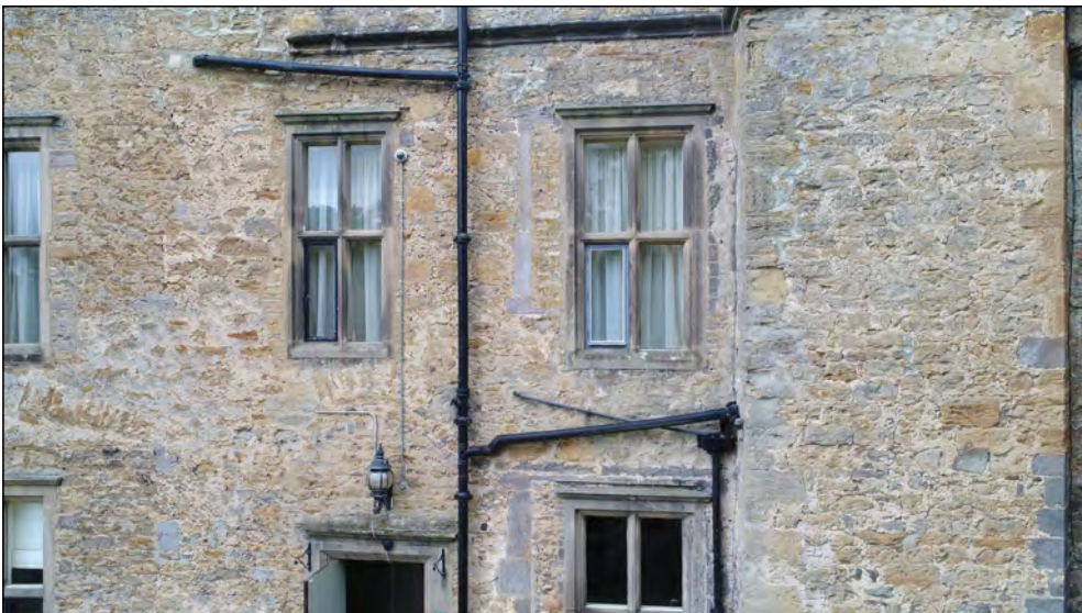
Photo 59. East facing exterior elevation, centre-south of east range, first floor.
