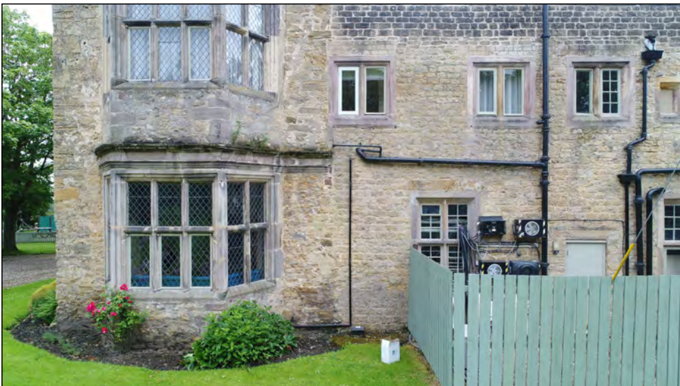
Photo 75. North facing exterior elevation, east end of North Range, ground floor.
