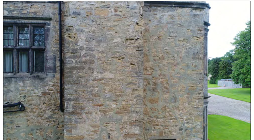
Photo 72. East facing exterior elevation, north end of East Range, first floor.
