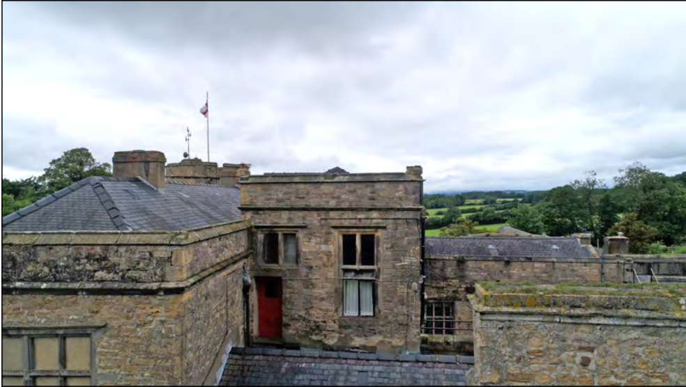
Photo 61. East facing exterior elevation of Renaissance facade second floor.
