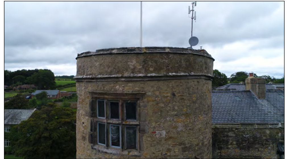
Photo 22. South facing exterior elevation of SW-tower, third floor, with detail of three-light transomed window.
