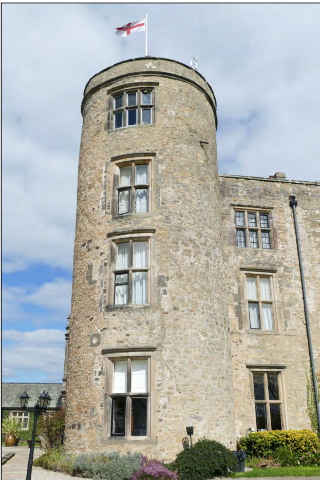
Photo 17. South facing exterior elevation of SW-tower.
