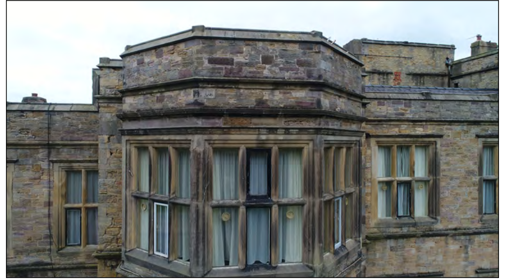
Photo 04. West facing exterior elevation, bay window, first floor.
