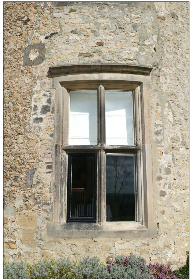
Photo 18. Detail of SW facing, cross window in ground floor of SW-tower.
