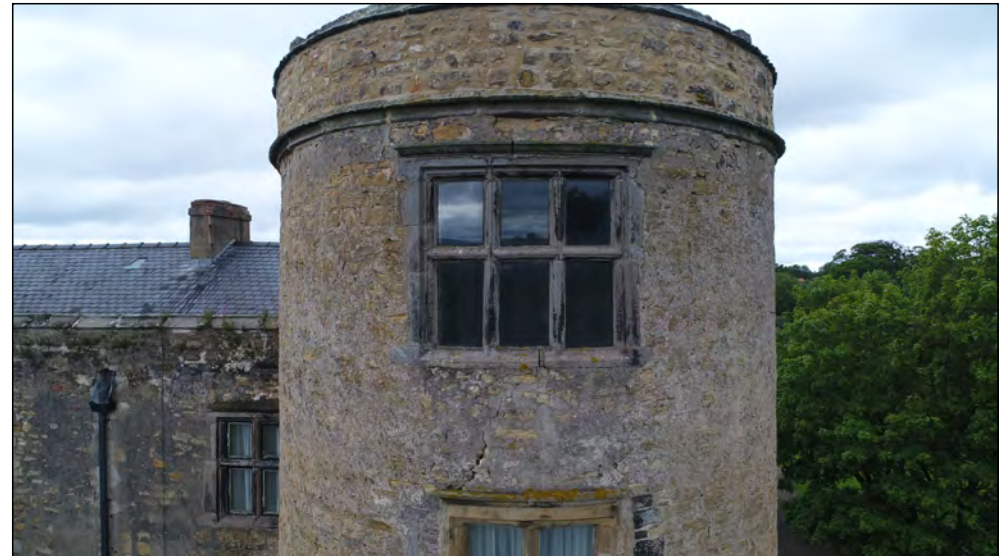
Photo 44. South facing exterior elevation of SE-tower, third floor.
