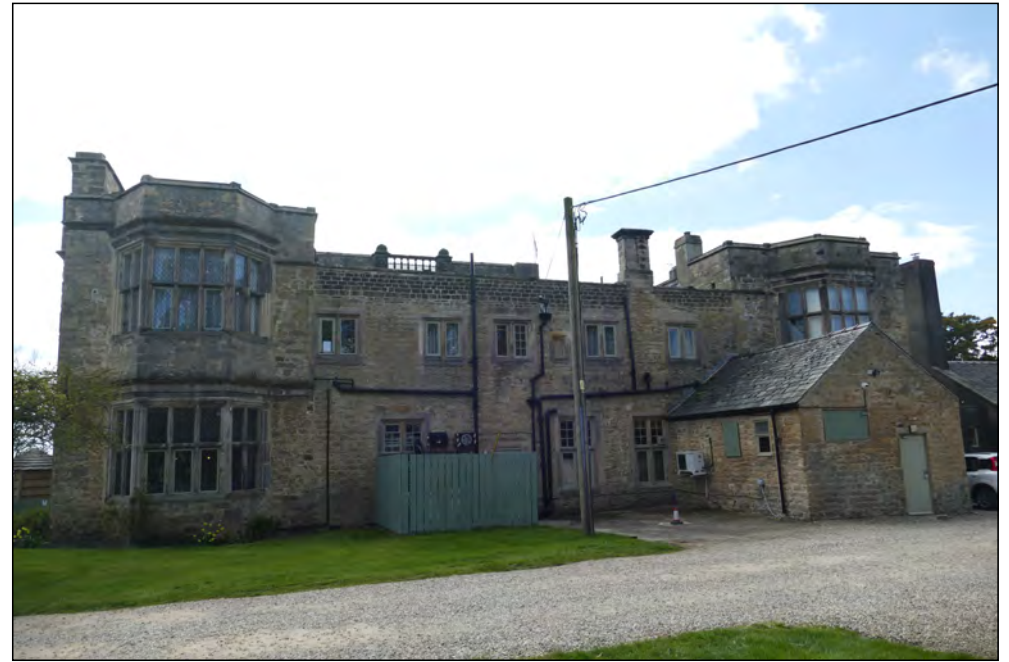
Photo 74. View of Walworth Castle North Range, north facing exterior elevation.
