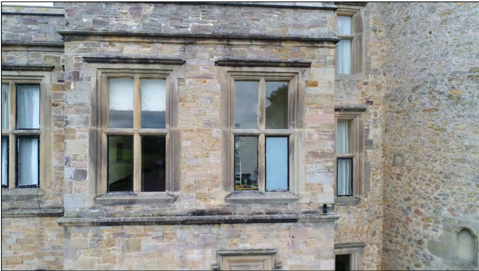
Photo 09. West facing exterior elevation, above reception entrance, first floor.
