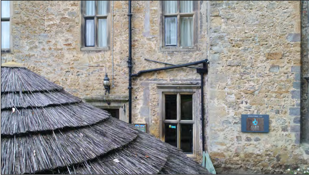
Photo 57. East facing exterior elevation, centre-south of east range, ground floor.
