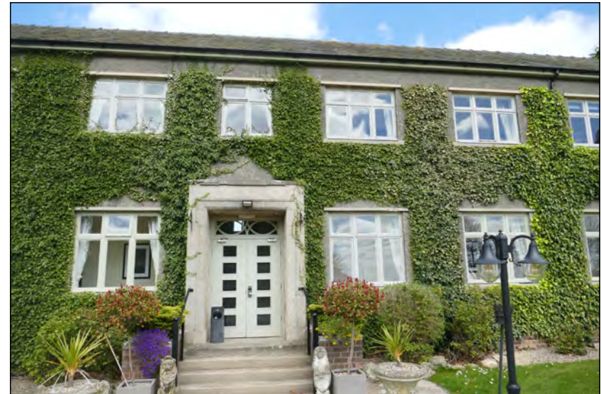
Photo 100. Detail of south facing entrance doorway to modern accommodation wing.
