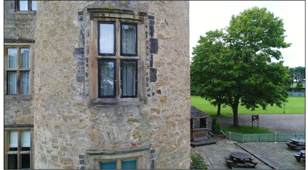
Photo 42. South facing exterior elevation of SE-tower, first floor.
