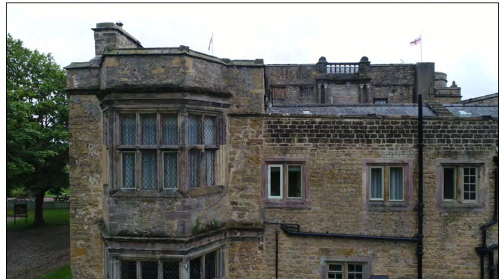
Photo 76. North facing exterior elevation, east end of North Range, first floor.
