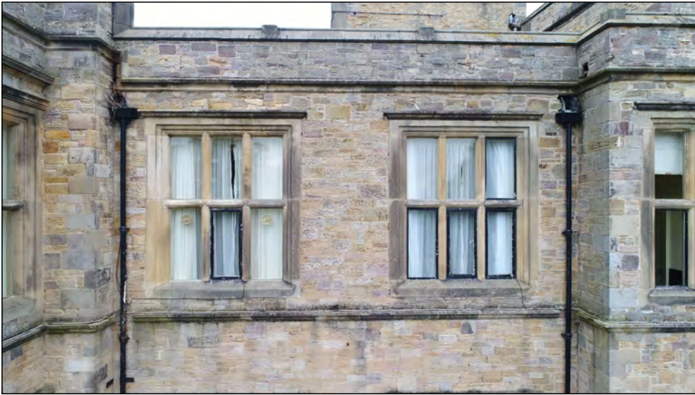
Photo 07. West facing exterior elevation, north of reception entrance, first floor.
