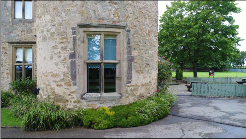
Photo 41. South facing exterior elevation of SE-tower, ground floor.
