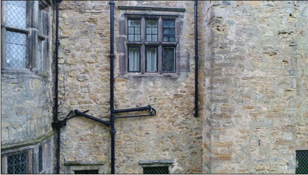
Photo 69. East facing exterior elevation, centre-north of East Range, first floor.
