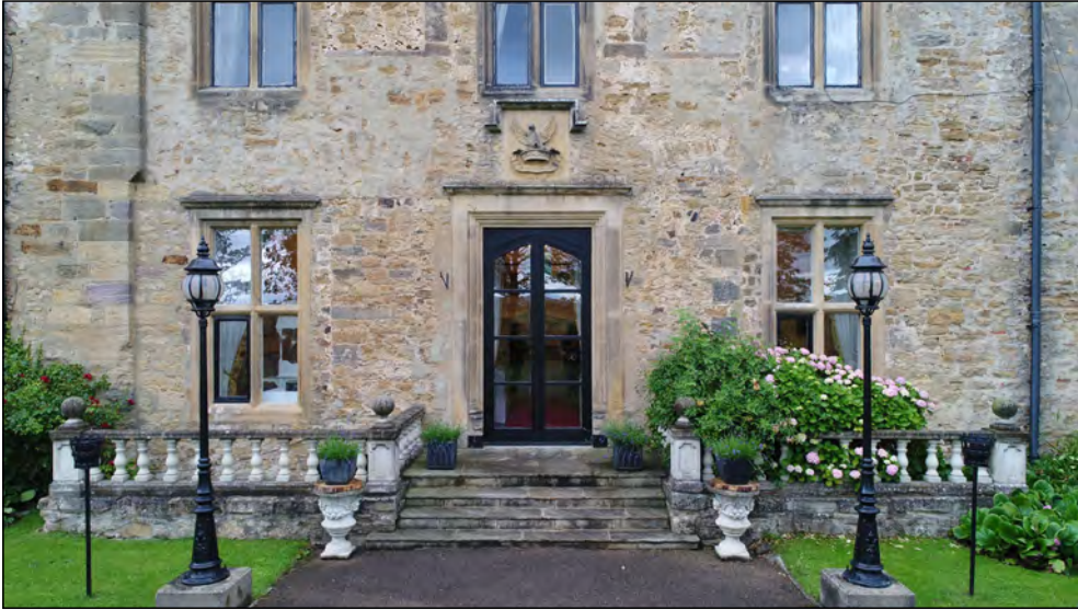
Photo 31. South facing exterior elevation, centre of former manor house, ground floor, showing entrance.
