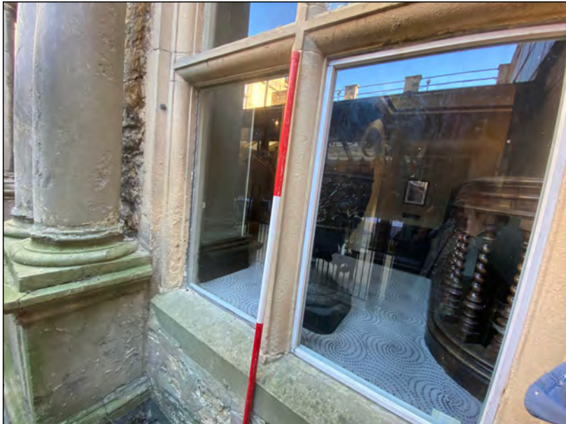
Photo 111. Detail of window on west side of door in Renaissance facade.
