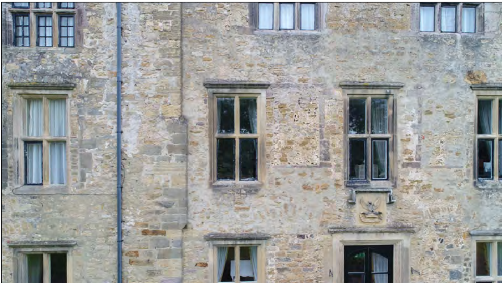
Photo 29. South facing elevation, centre-west part of former manor house, first floor.
