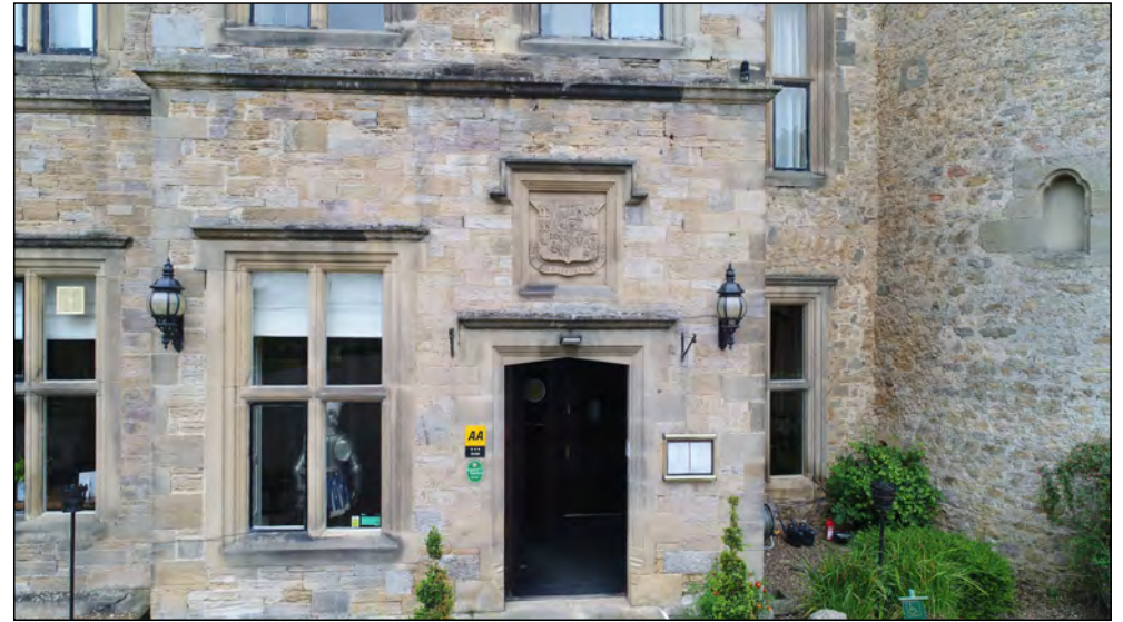
Photo 08. West facing exterior elevation, reception entrance, ground floor.
