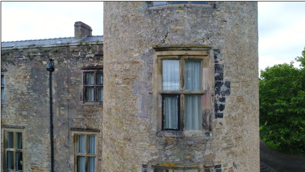
Photo 43. South facing exterior elevation of SE-tower, second floor.
