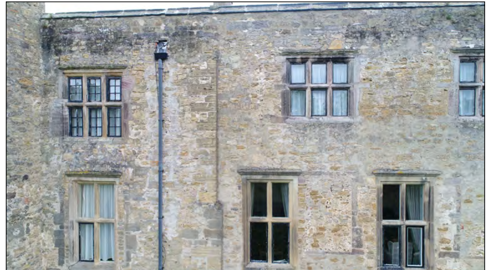
Photo 30. South facing elevation, centre-west part of former manor house, second floor.
