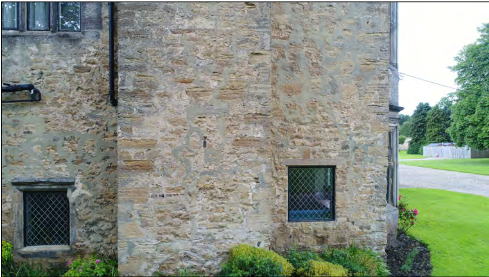
Photo 71. East facing exterior elevation, north end of East Range, ground floor.
