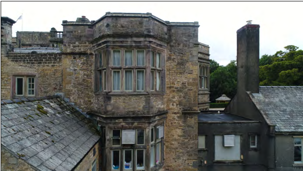
Photo 87. North facing exterior elevation, west end of North Range, ground-first floor.
