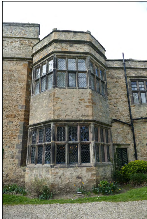
Photo 63. East facing exterior elevation of bay towards centre of East Range.
