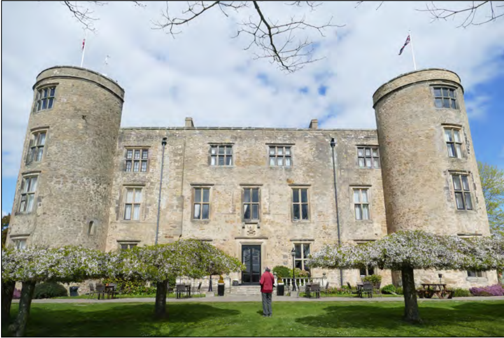
Photo 23. South facing exterior elevation of Walworth Castle.
