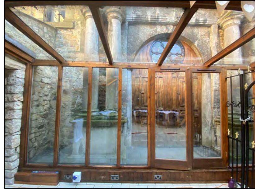
Photo 102. North facing elevation of Renaissance facade, ground floor, from east side of conservatory.
