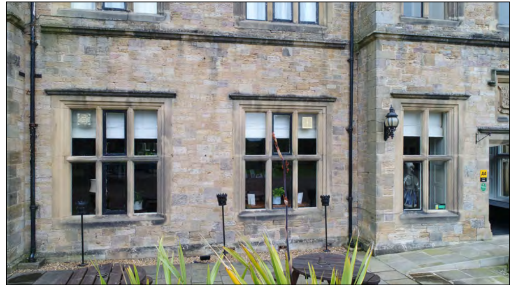
Photo 06. West facing exterior elevation, north of reception entrance, ground floor.
