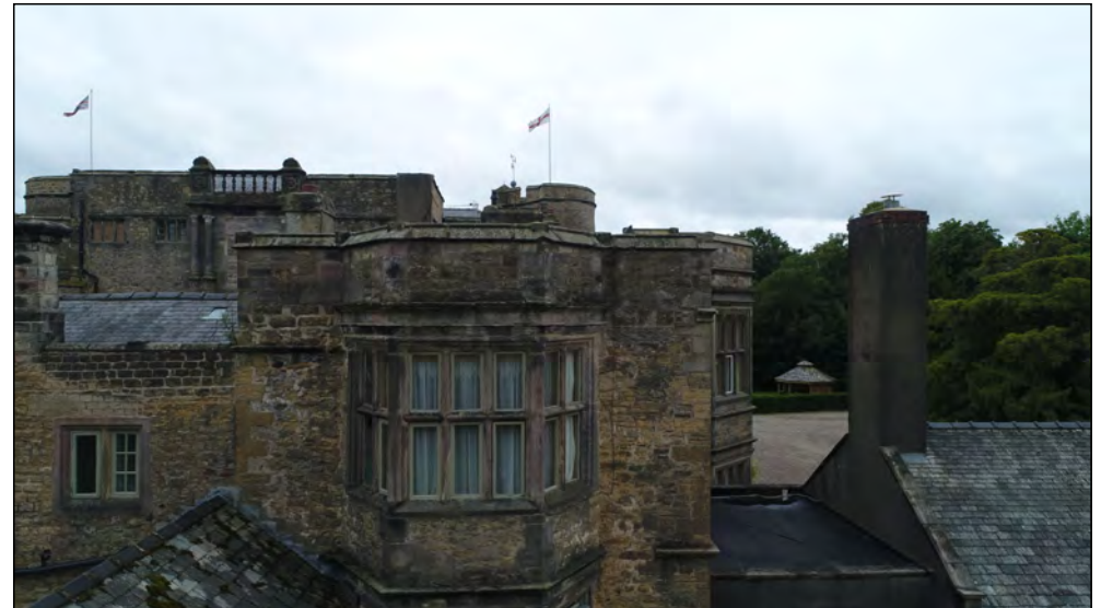
Photo 88. North facing exterior elevation, west end of North Range, first floor.
