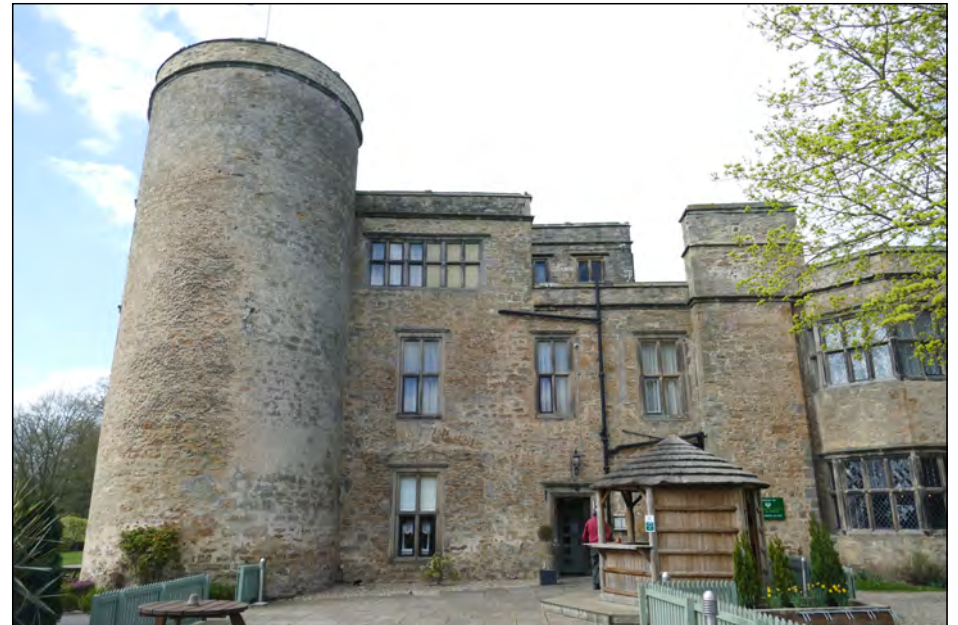
Photo 48. East facing exterior elevation of Walworth Castle south end.
