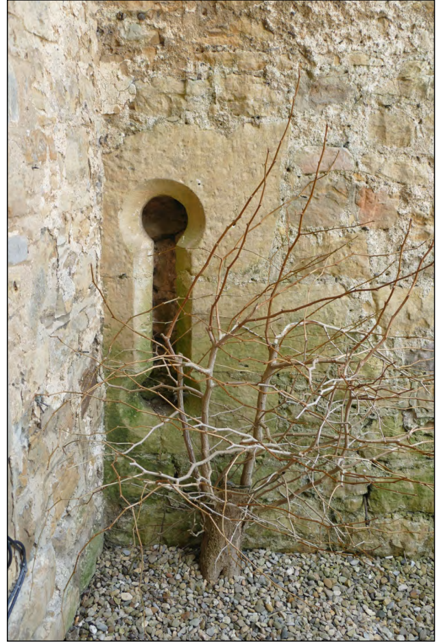
Photo 16. Detail of gunloops in tower, facing north, ground floor.
