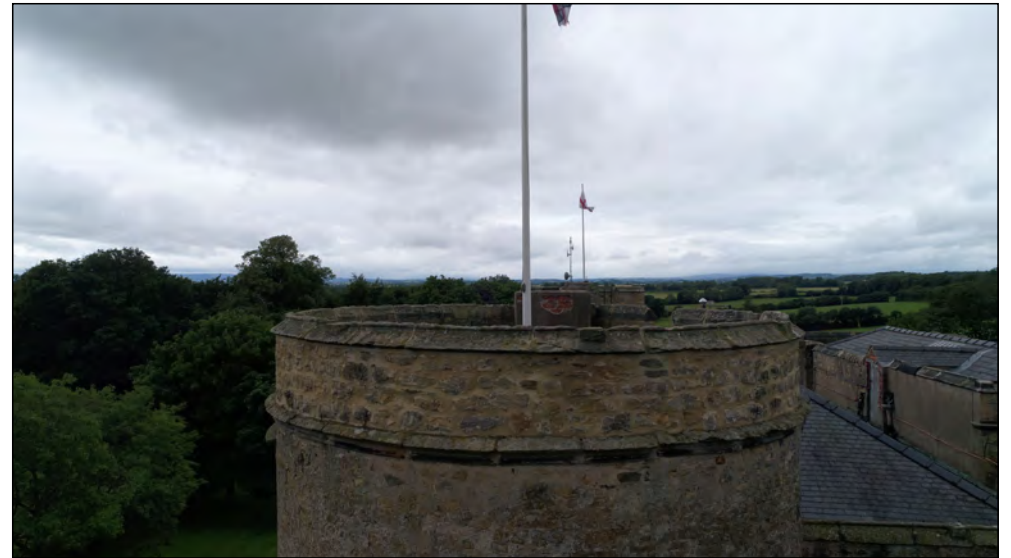
Photo 52. East facing exterior elevation of SE-tower, third floor and roof.
