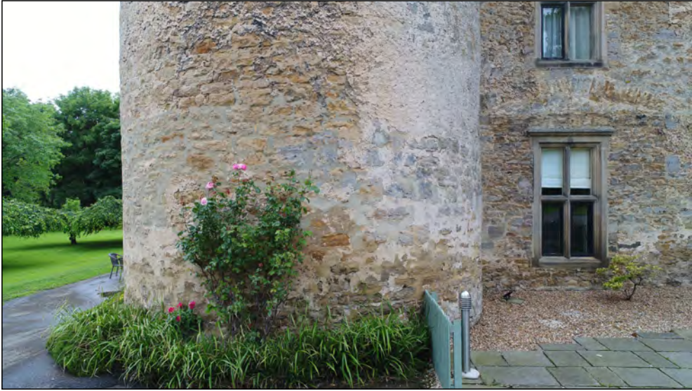
Photo 49. East facing exterior elevation of SE-tower, ground floor.
