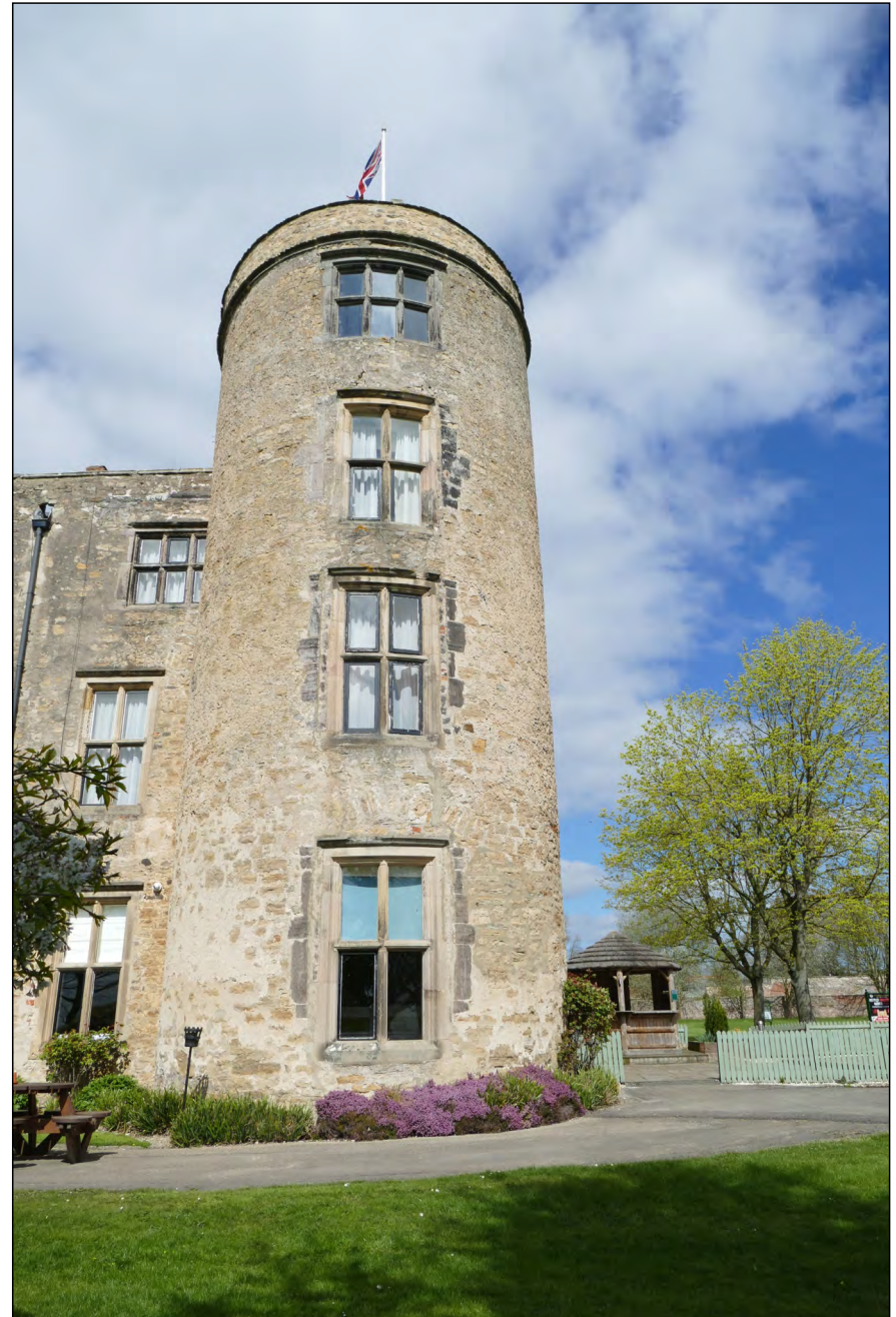
Photo 36. South facing exterior elevation of SE-tower.
