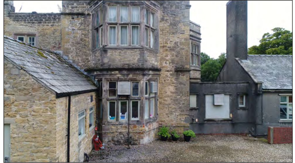
Photo 86. North facing exterior elevation, west end of North Range, ground floor.
