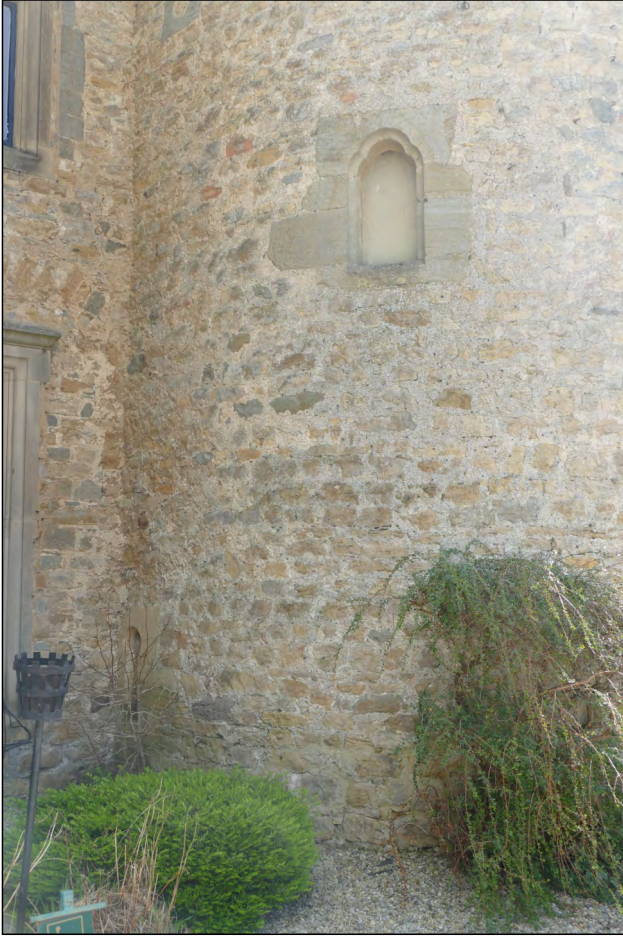
Photo 15. Detail of north facing single window with trefoil head in first floor of tower.
