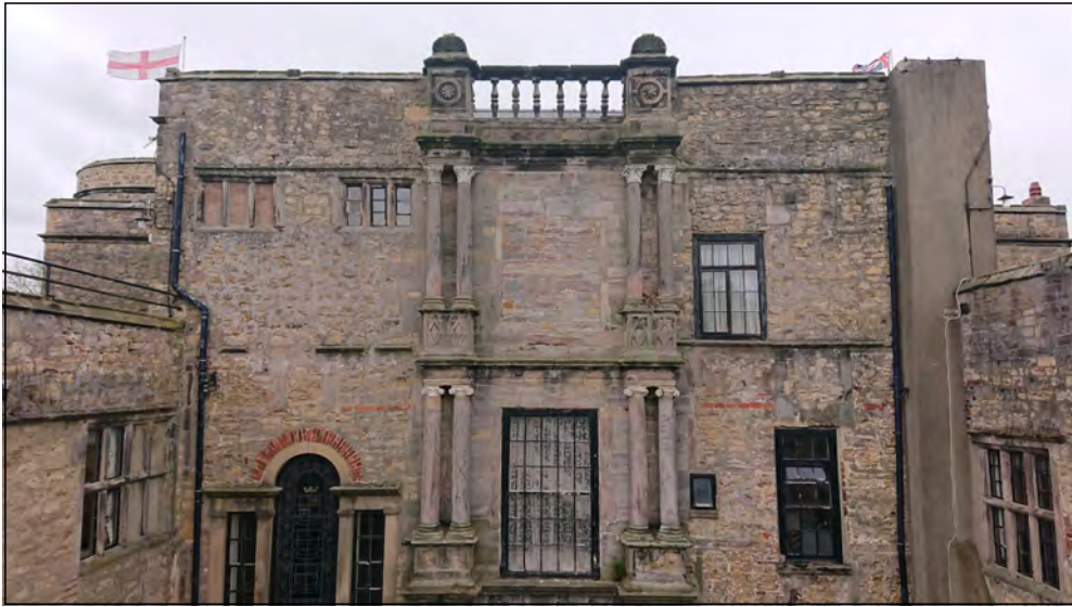
Photo 89. North facing exterior elevation of former manor house, Renaissance facade, first-second floors, taken from roof of North Range.
