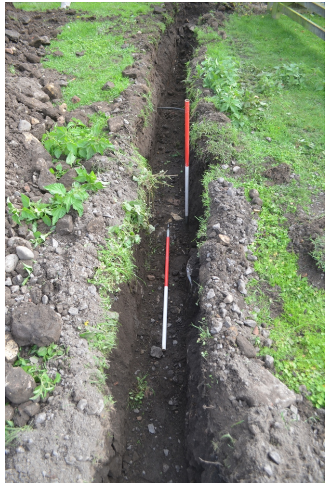
Photo 22. View looking west at pipe trench.
