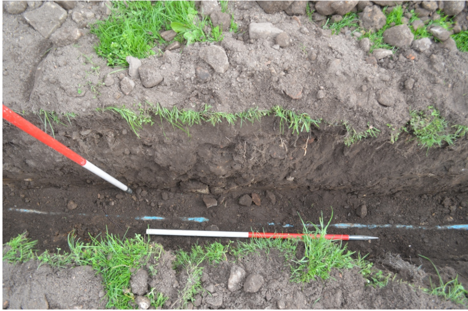
Photo 17. View of the west-facing section of the pipe trench.
