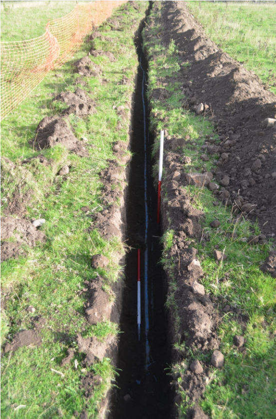
Photo 04. View of pipe trench looking north.
