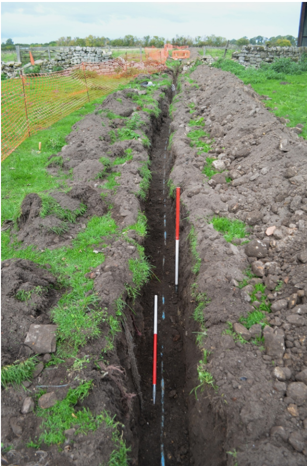
Photo 18. View looking north of pipe trench.
