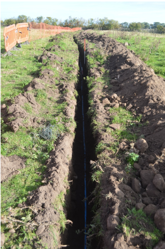
Photo 12. View of pipe trench looking north.
