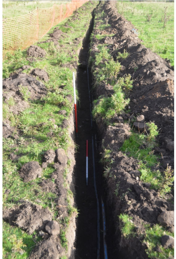
Photo 05. View of pipe trench looking north.
