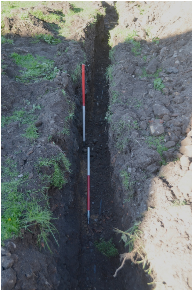
Photo 21. View looking east of pipe trench.
