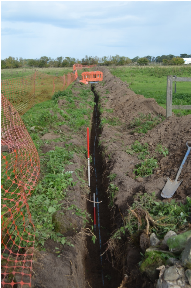
Photo 15. View looking north of pipe trench.
