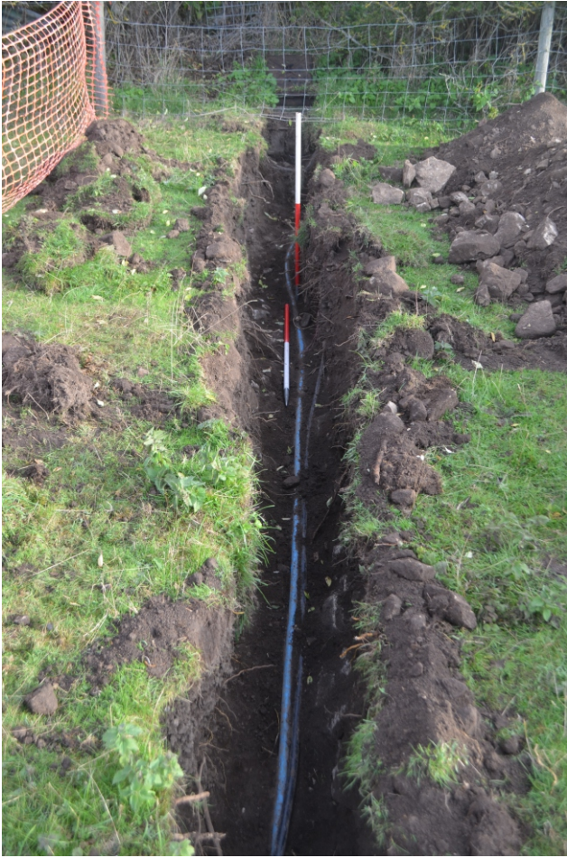
Photo 01. View looking north of pipe trench.
