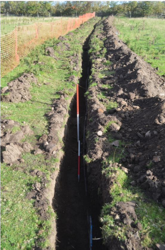
Photo 06. View of pipe trench looking north.
