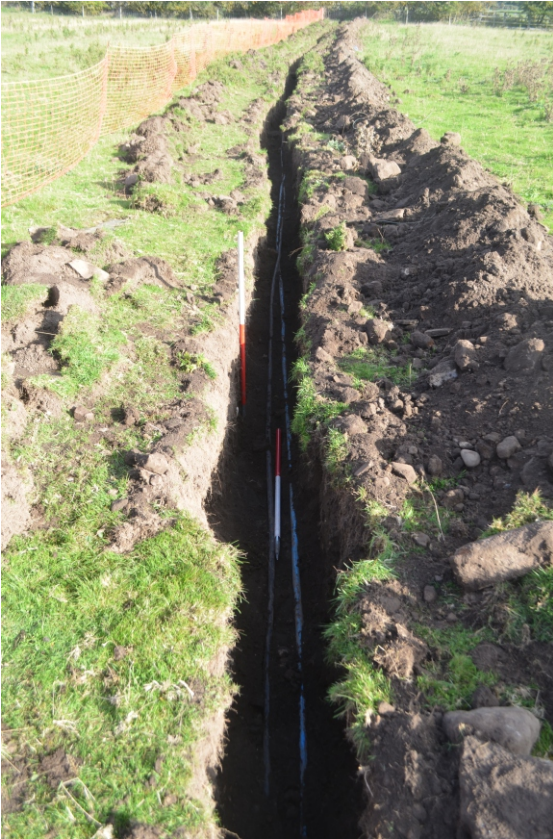
Photo 10. View of pipe trench looking north.
