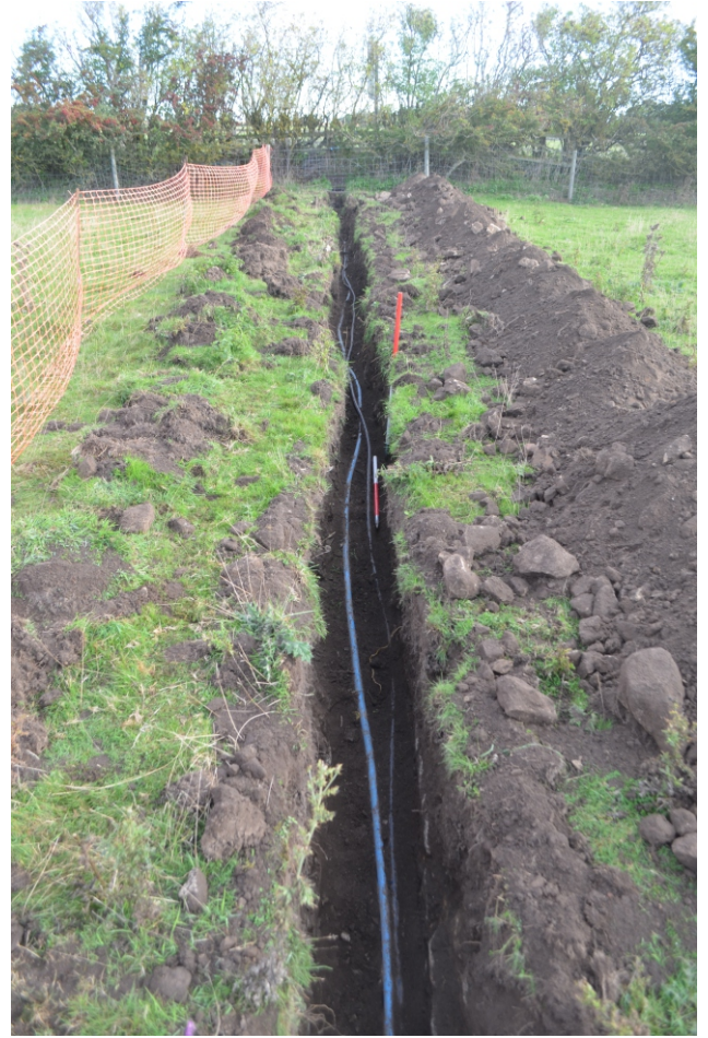
Photo 02. View looking north at pipe trench.
