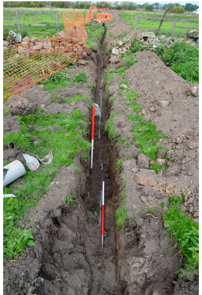
Photo 16. View looking north at pipe trench.
