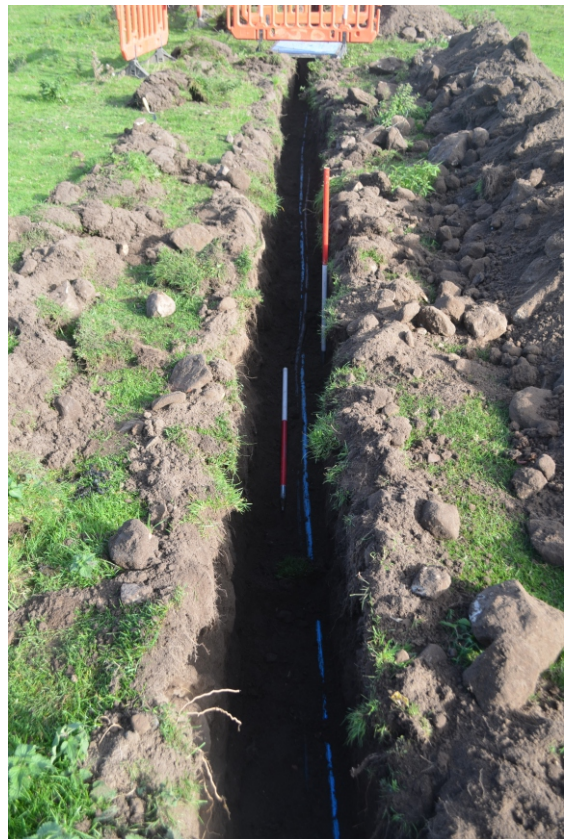
Photo 13. View of pipe trench looking north.
