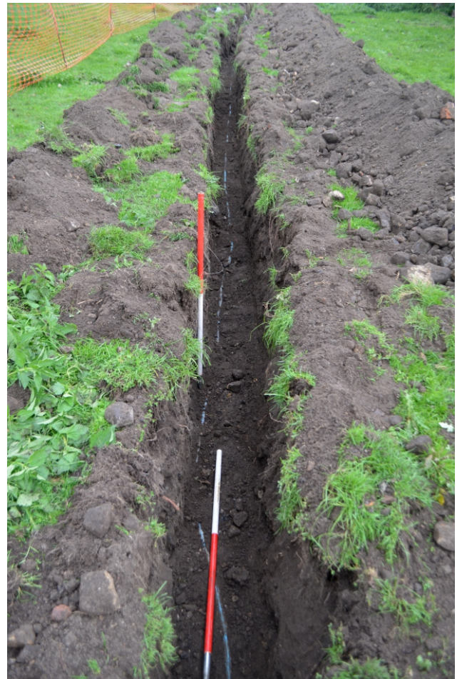
Photo 19. View looking north at pipe trench.
