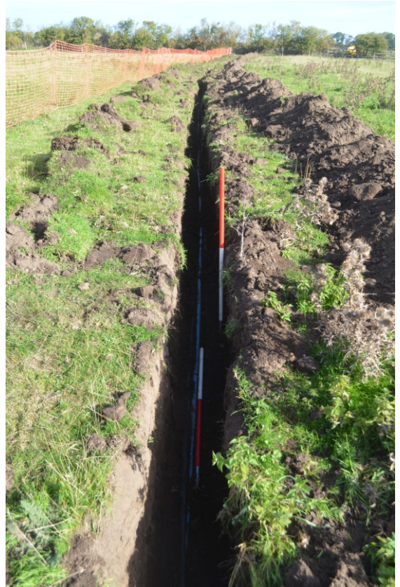
Photo 11. View of pipe trench looking north.
