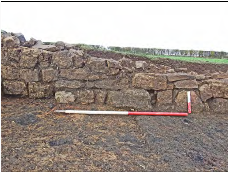
Photo 11. Trench 1 (West), south facing elevation of central part of Building 1 north wall [5113].
