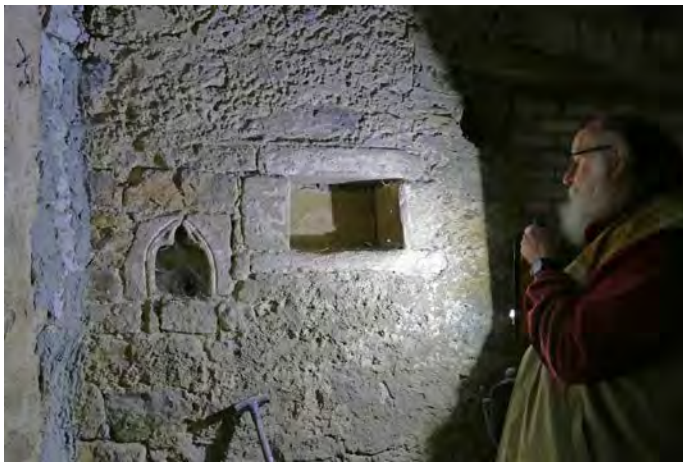
Illus. 08: Piscina and niche at the east end of the internal south wall of the former chapel
