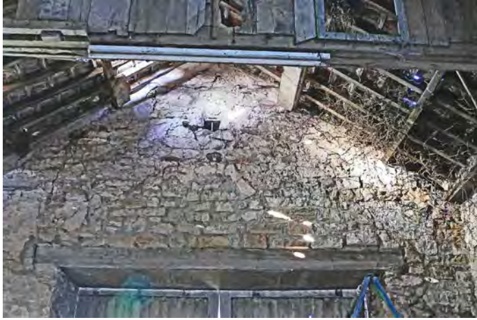
Illus. 07: The internal west gable elevation of the former chapel
