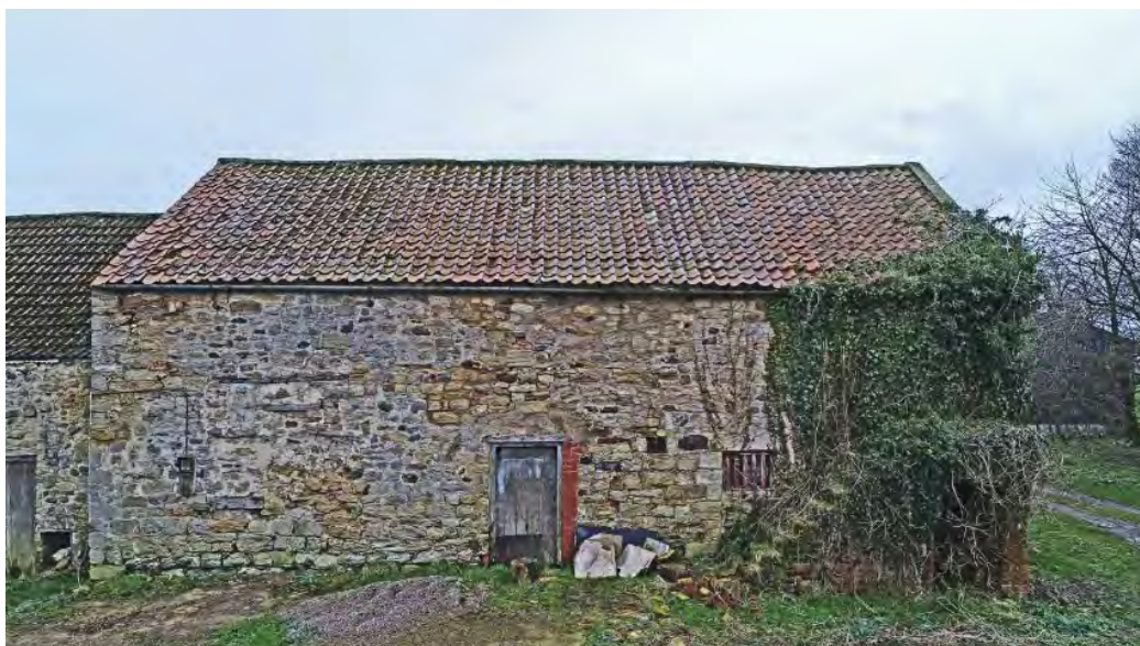
Illus. 06: The external north elevation of the former chapel
