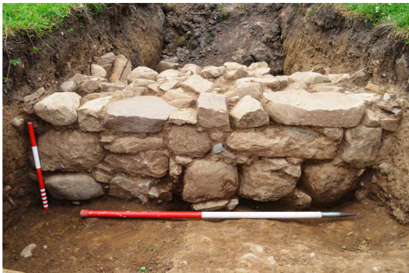
Photo 30: Wall [508], west view.
