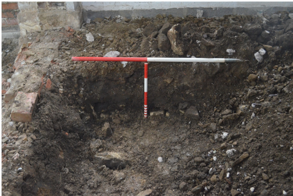
Photo 03. View looking west at excavations into made ground after concrete removal.
