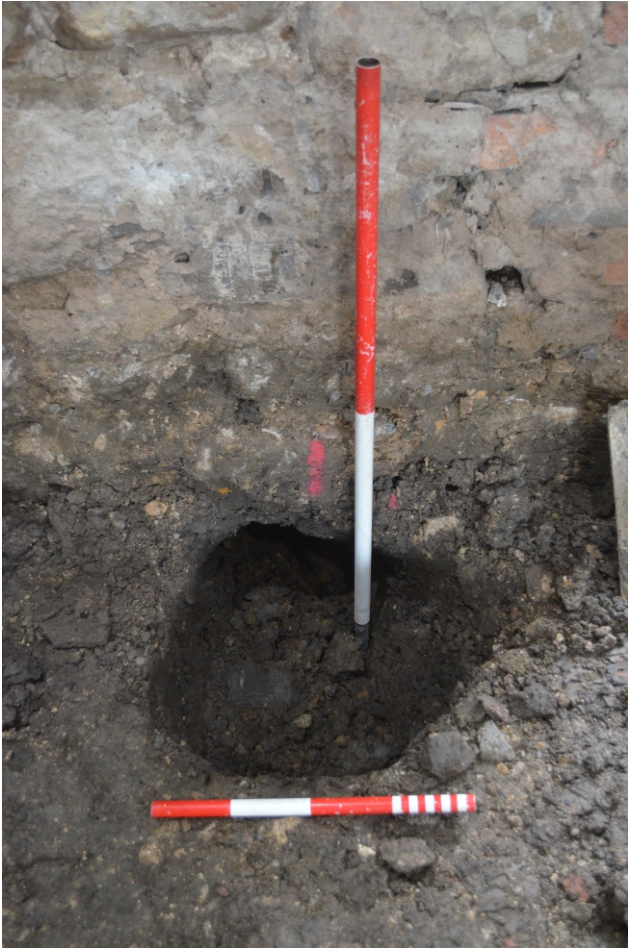
Photo 01. View looking north at pit excavated for drainage against the north wall of the building.
