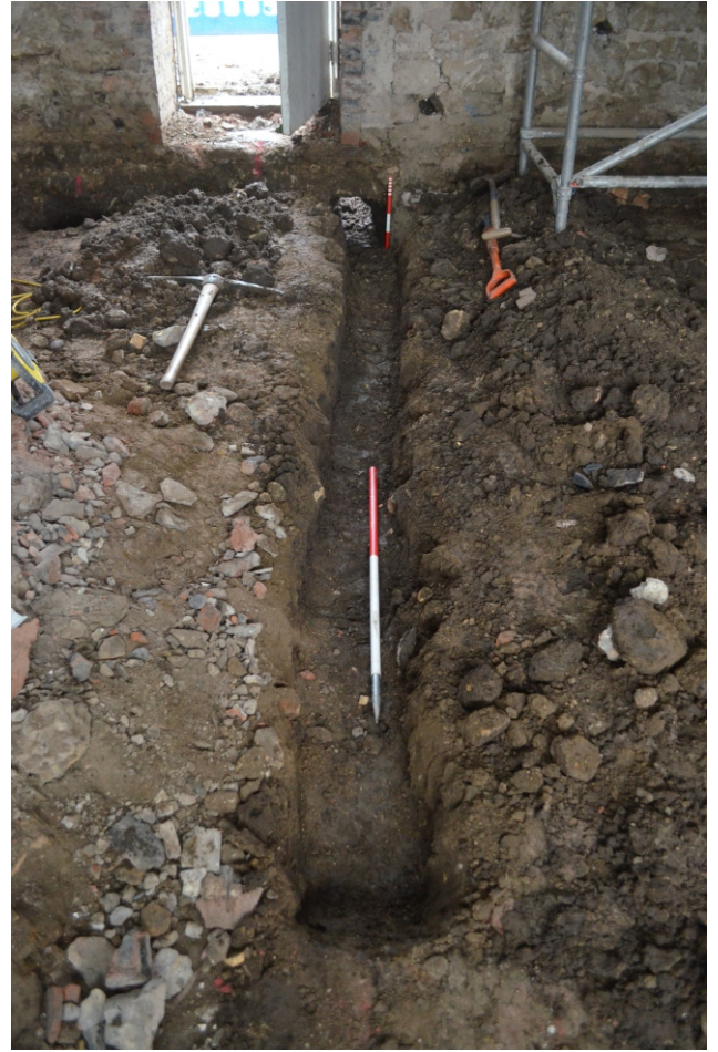
Photo 02. View looking north at excavated trench for drainage.
