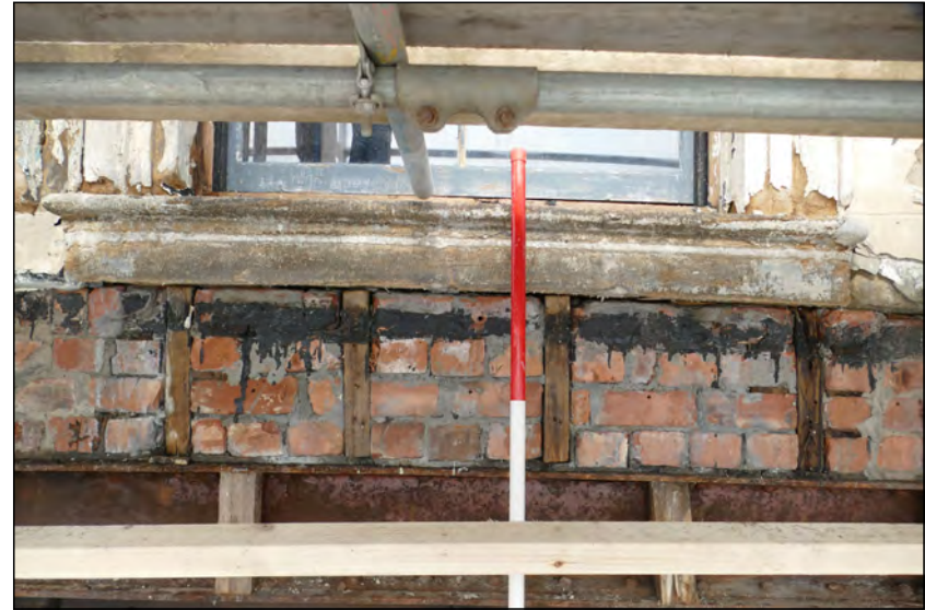
Photo 12. Interface between ground and first floors, view looking NNW at lower part of crumbling window architrave and lintel in the south wall, centre-west window of High Street West No. 1.
