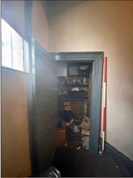
Photo 93. Door to storage cupboard on mid-stair landing (see Pic. 97).
