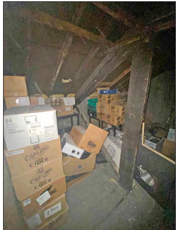
Photo 110. View looking NE across the attic, NW room.
