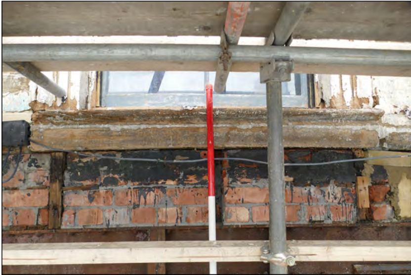
Photo 11. Interface between ground and first floors, view looking NNW at lower part of crumbling window architrave and lintel in the south wall, centre-east window of High Street West No. 1.
