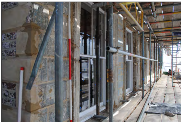
Photo 26. Exterior first floor, view looking ENE from the SW corner.
