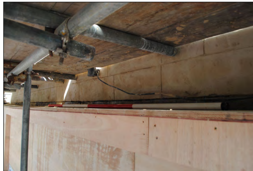
Photo 38. Interface between first and ground floors, exterior, south wall, view looking WNW at repointed stonework.
