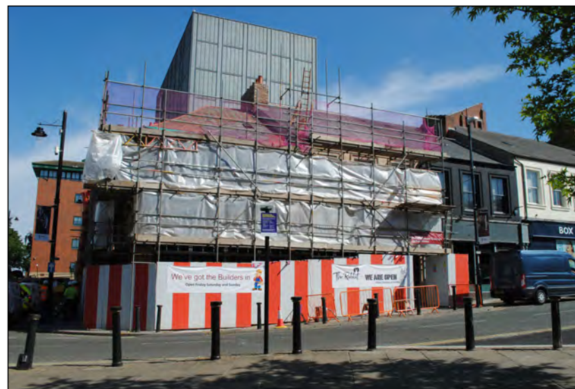
Photo 40. Broad view looking North at 'The Rabbit', whilst undergoing renovation work.
