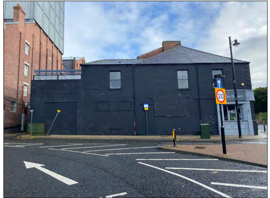
Photo 02. West elevation, prior to renovation works.
