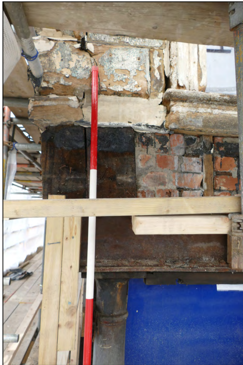
Photo 11. Interface between ground and first floors, view looking NNW at lower part of crumbling window architrave and lintel in the south wall, centre-east window of High Street West No. 1.
