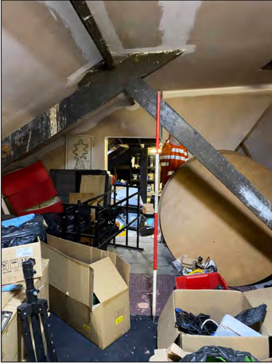
Photo 99. View looking WSW along central part of attic space.
