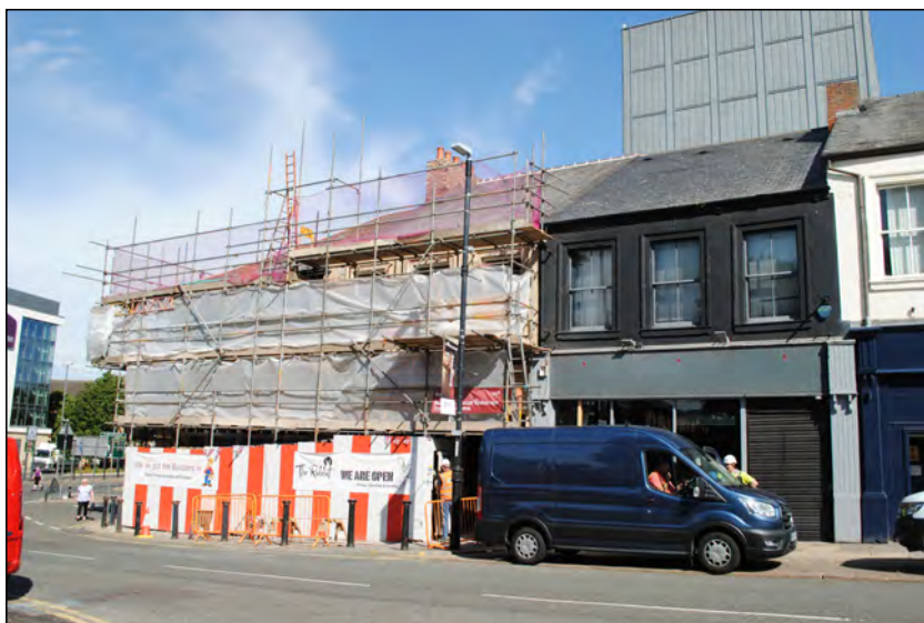
Photo 39. Broad view looking NW at 'The Rabbit', whilst undergoing renovation work.
