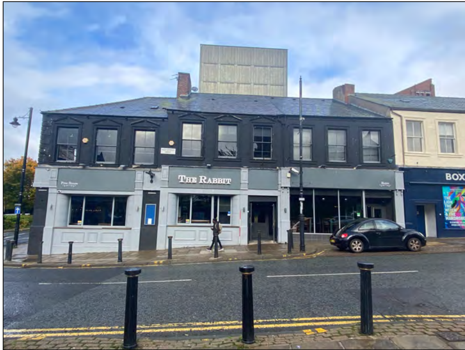
Photo 01. South elevation, prior to renovation works.
