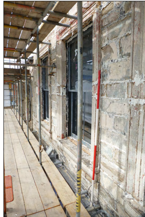
Photo 12. Interface between ground and first floors, view looking NNW at lower part of crumbling window architrave and lintel in the south wall, centre-west window of High Street West No. 1.
