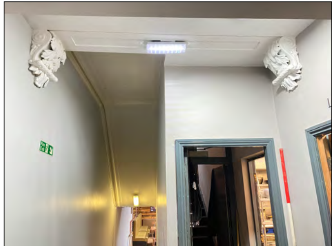
Photo 90. A metre or so south of 89, with detail of scrolled brackets with leaf design, located at the top of the stairs.
