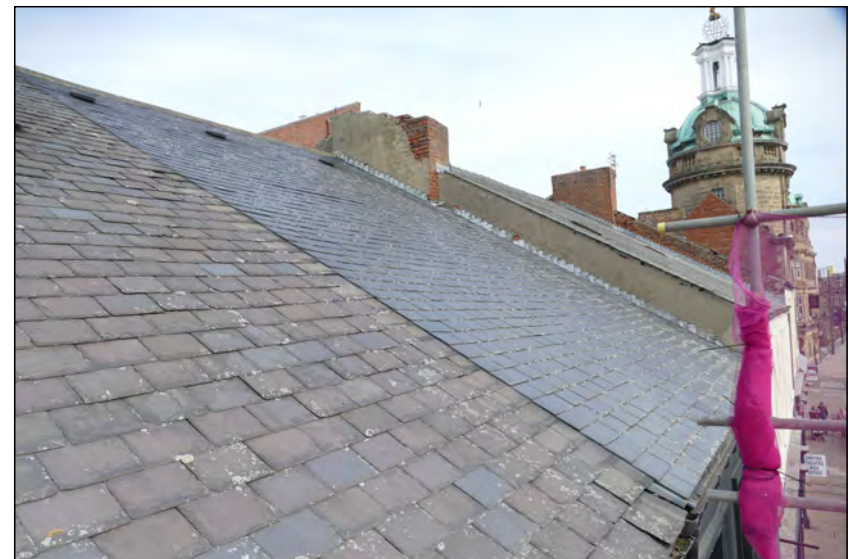
Photo 18. External roof of High Street West Nos. 2-3, view looking ENE.
