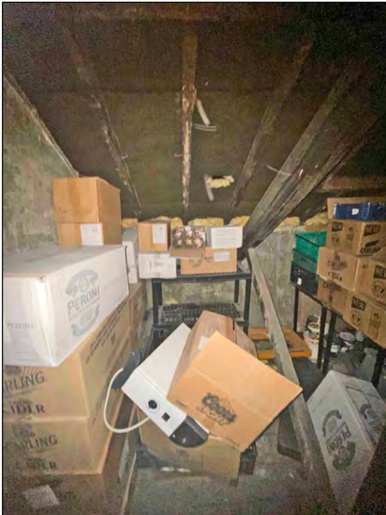
Photo 111. View looking NNW at NW room in attic space.
