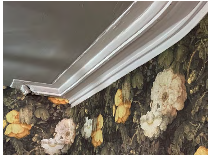
Photo 98. Interior ground floor, west wall, view looking SSW at regency cornice.
