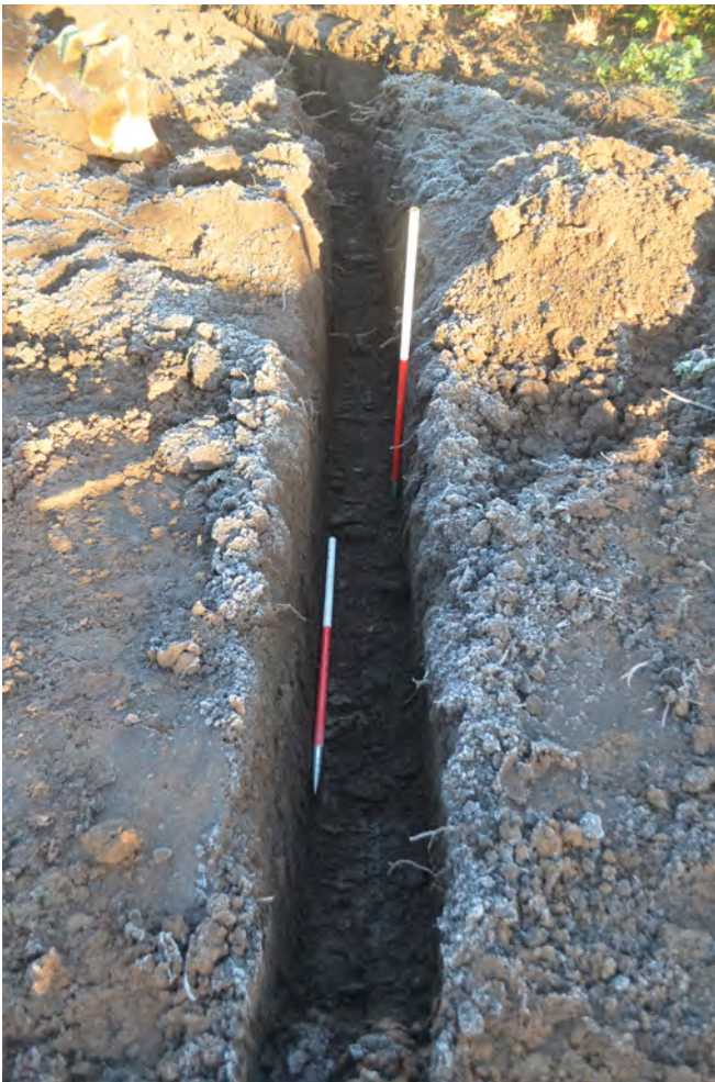
Photo 05. The NE-SW pipe trench. NE view.
