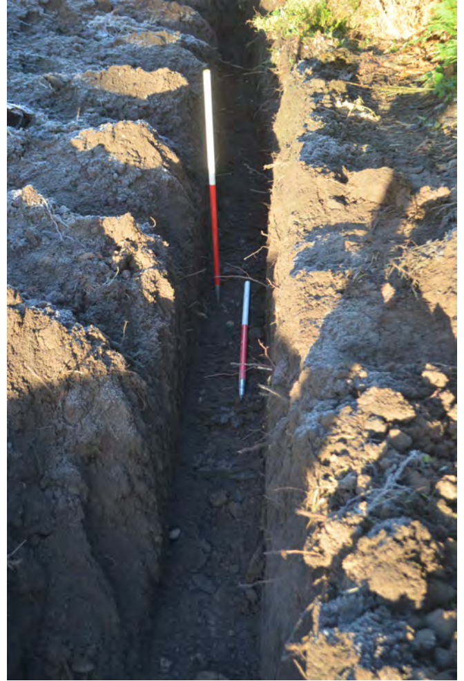
Photo 08. The north end of the N-S pipe trench. N view.
