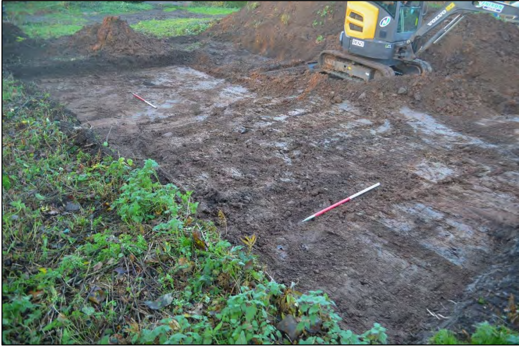
Frontispiece: Stripping of topsoil at Land West of Braeside, Branxton, Northumberland.
