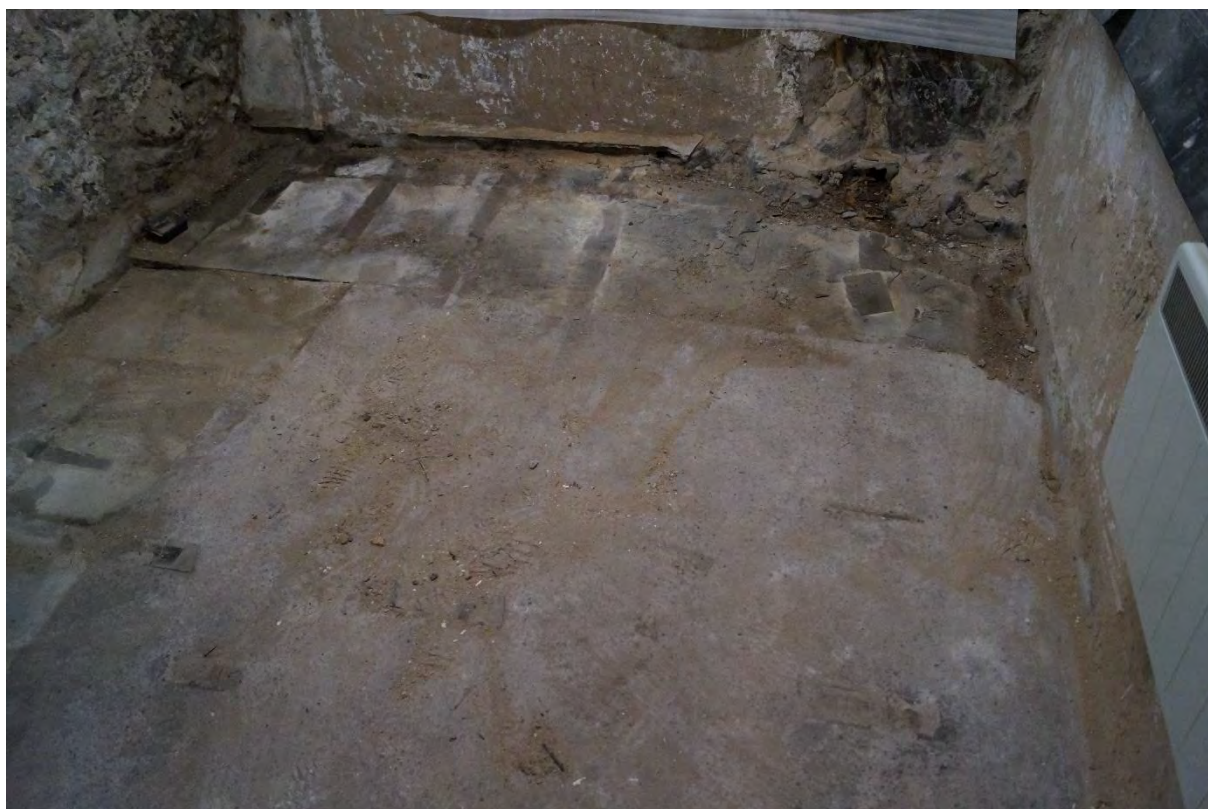
Concrete floor, Butler's Pantry, looking west
