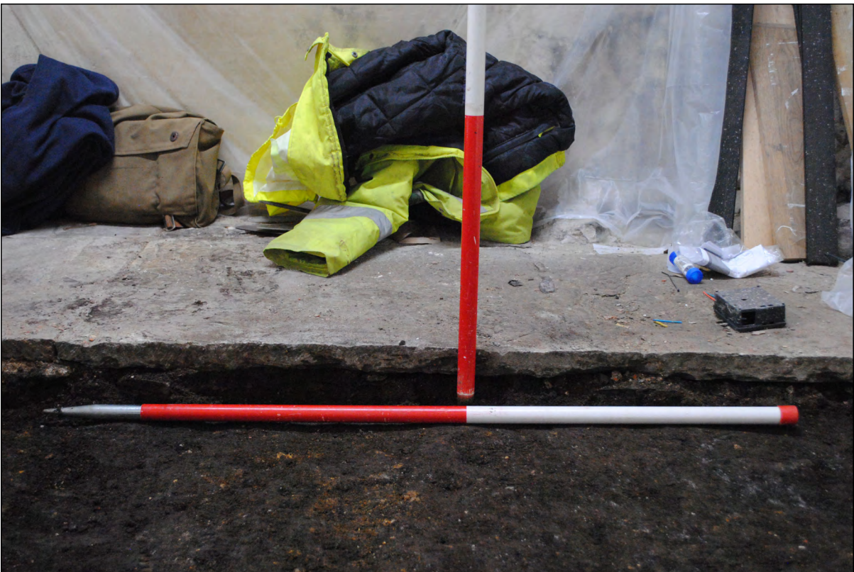
Photo 8. East facing section of the Butler's Pantry floor, following excavation of concrete debris and rubble layers.
