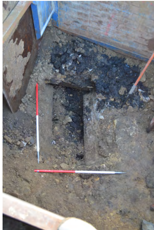
Photo 25. The culvert [115], as exposed in a trial pit in the eastern end of site. SE view.
