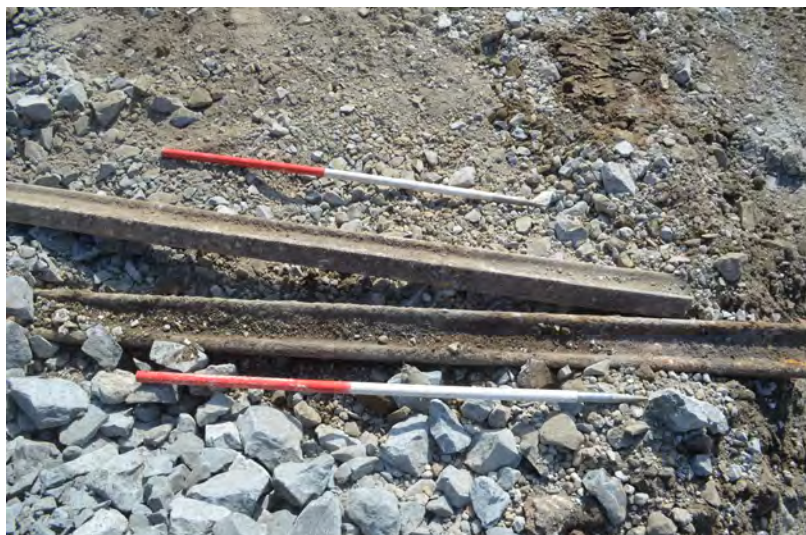
Photo 52. The rails observed on the top of concrete structure [125].
