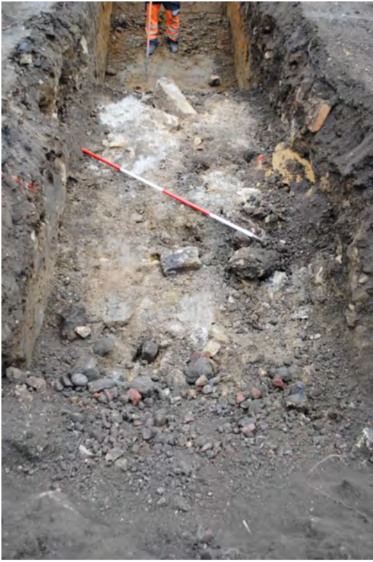
Photo 07. The culvert in area 2, before the removal of capping stone, SW view.
