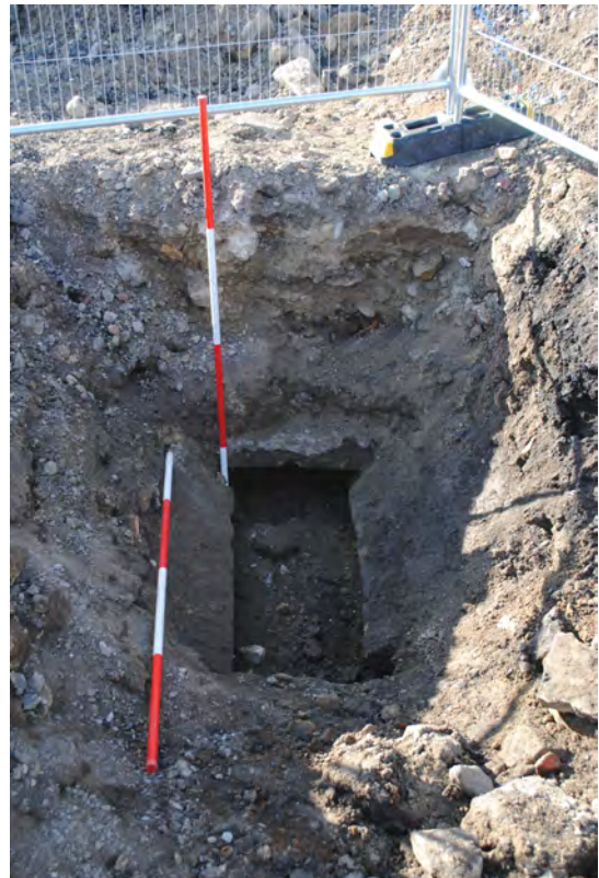
Photo 16. Area 3, the culvert with capping stones removed, SSE view.
