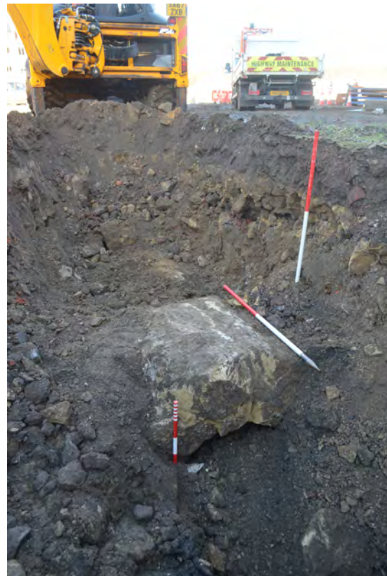
Photo 28. Detail shot of the vaulted capping stones of the culvert, N view.
