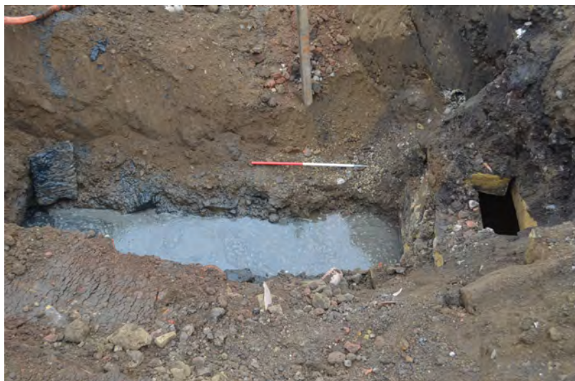
Photo 34. The culvert's NW-SE leg at the point of feeding into chamber [116]. The NE-SW leg joins where the wooden stake has been embedded in the spoil.
