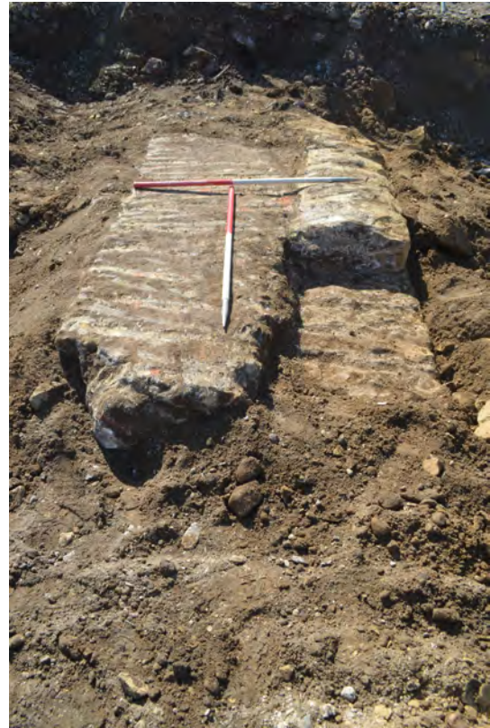
Photo 51. The concrete structure [125] encountered during excavation of the roadway. SW view.
