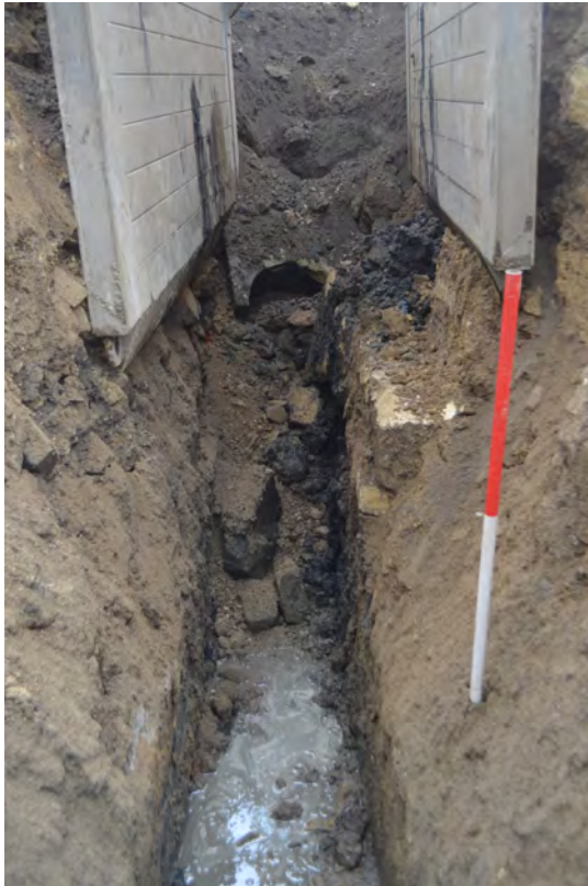
Photo 44. The NW-SE culvert, showing a section of reinforced wall and one half of a latrine chute course amongst the demolition debris. SE view.
