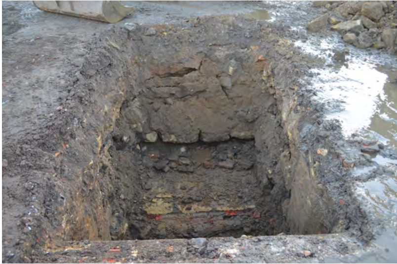
Photo 23. E view, showing the culvert as exposed in a trial pit.
