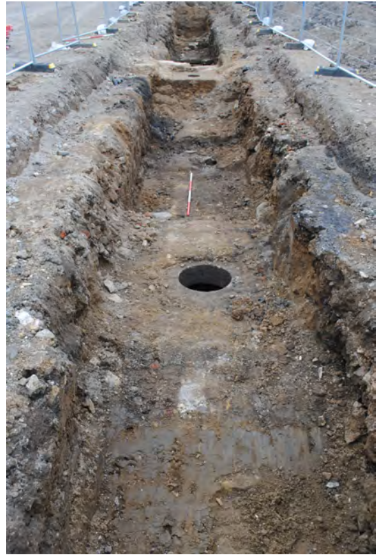
Photo 08. Area 1, stripped down to the culvert surface and showing chute [107]. NE view.
