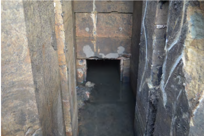
Photo 38. The inside of the chamber. NW view.
