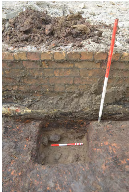
Photo 64. A small trial hole showing the depth of layer (132) below the school front wall foundations and overlying probable natural (135). NW view.
