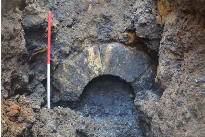
Photo 41. S view, showing a small area of vaulted capping on the NW-SE leg of the culvert.
