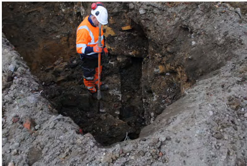
Photo 09. The culvert [115] in area 2, with capping stones removed and the small channel feeding it revealed. Working shot, W view.
