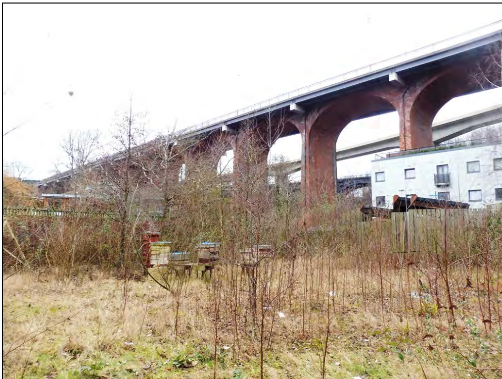
Frontispiece: A view of the interior of the Kelly's Yard site, looking north-west, towards Byker Bridge, the Metro bridge and the Ouseburn railway viaduct.
