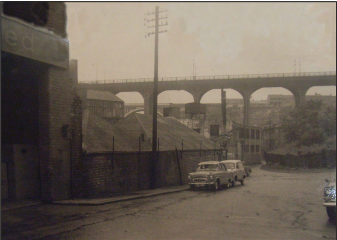
Figure 12: View of Foundry Lane looking north towards Kelly's Yard, 1963 (NL Acc.63084)
