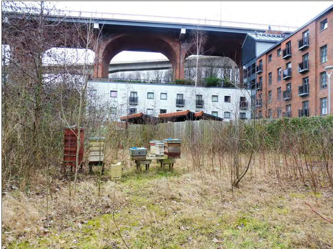
Photo 1: View of the interior of the Kelly's Yard site, looking north, with the new Farm View apartment blocks, Byker Bridge and the Metro Bridge beyond.
