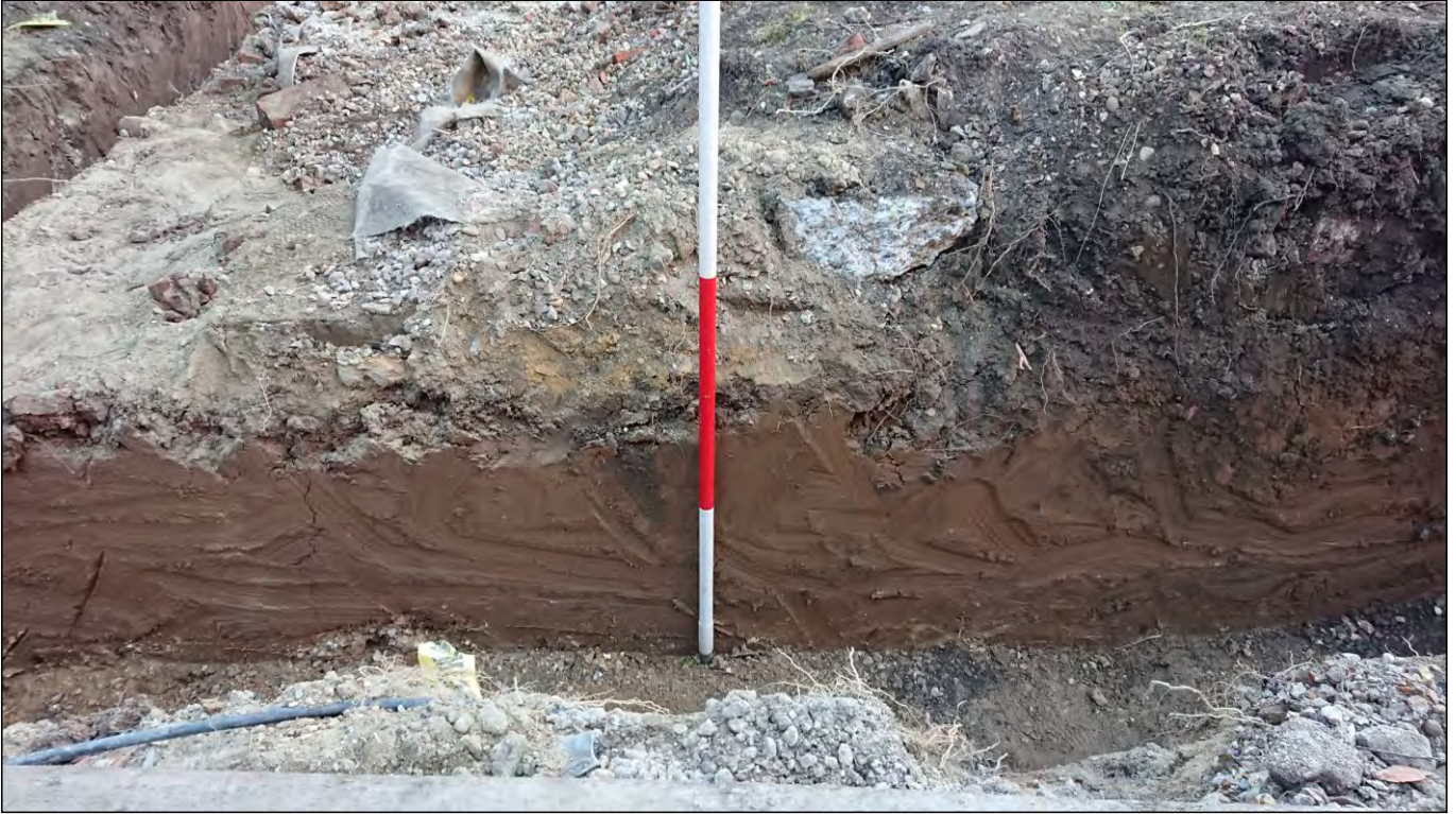
Photo 05. Foundation trench B-E, north facing section.
