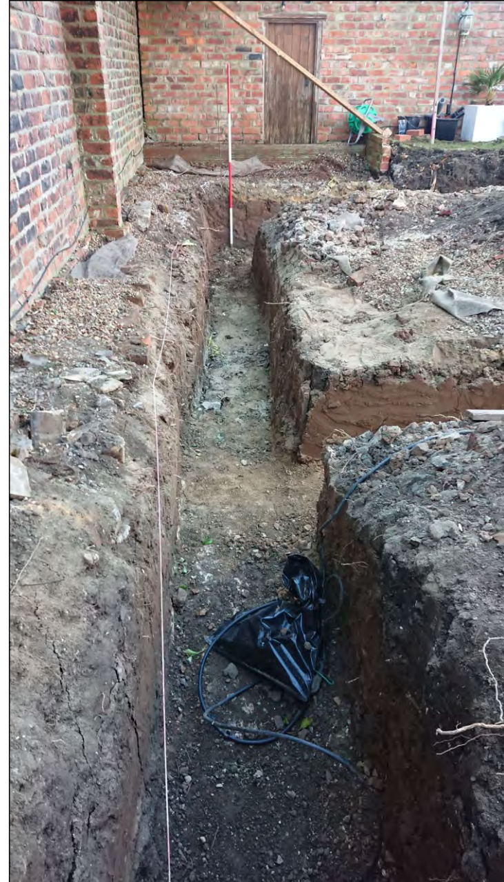
Photo 14. Foundation trench G-D, view looking south.
