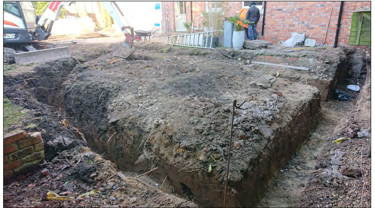
Photo 16. Broad view across site following foundation trench excavations, looking north-west from G.
