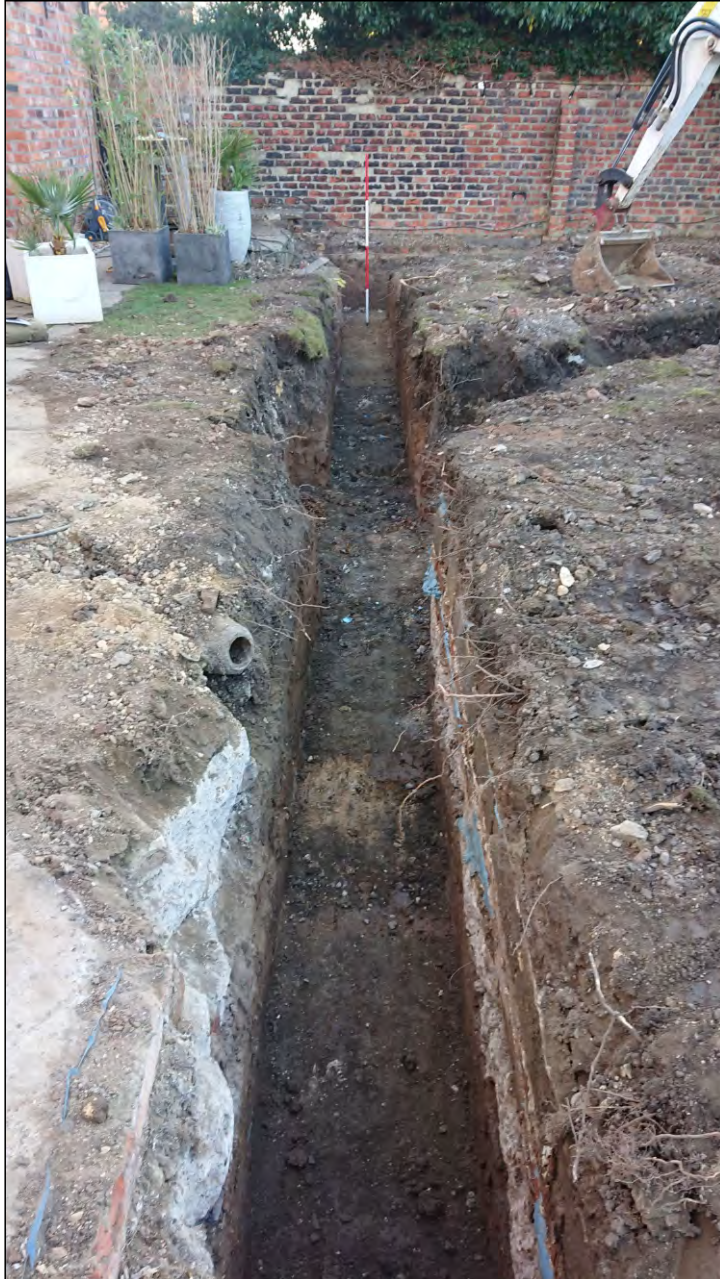
Photo 03. Foundation trench A-B, view looking east.
