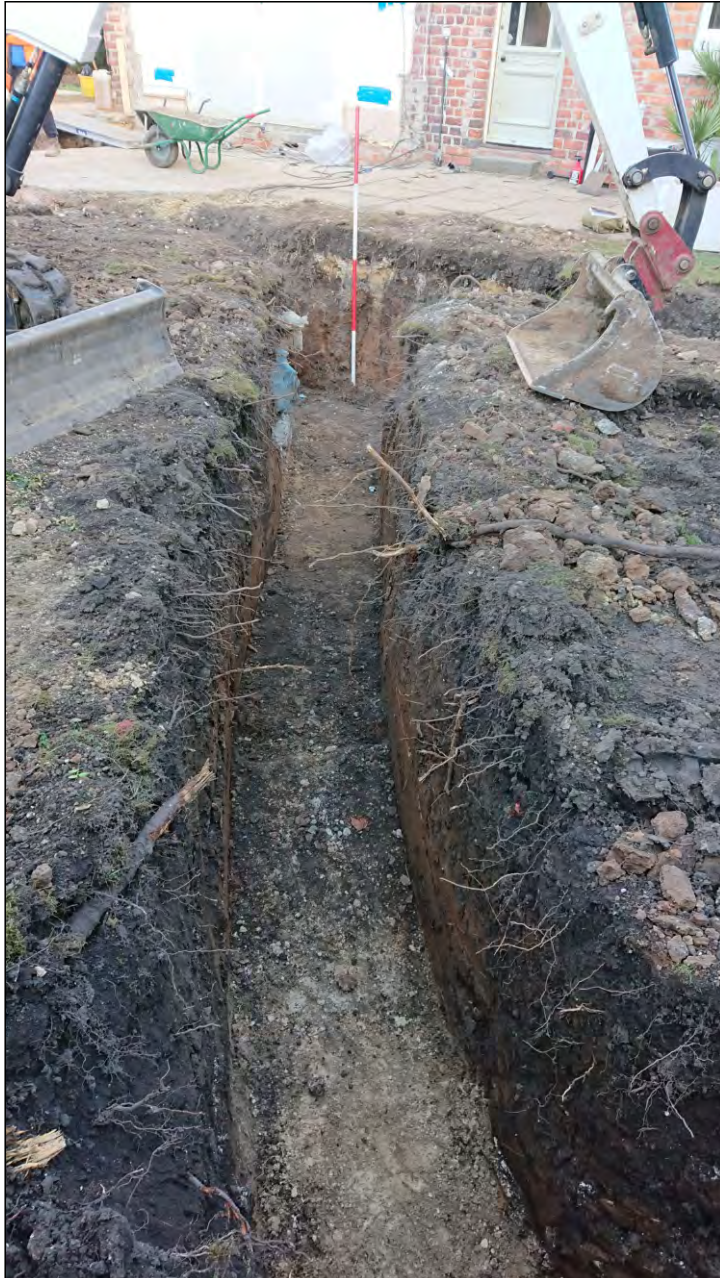
Photo 11. Foundation trench F-E, view looking north-west.
