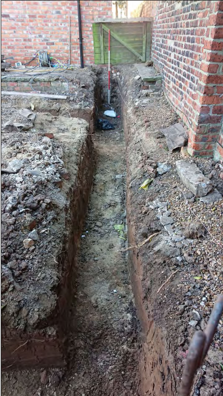
Photo 13. Foundation trench G-D, view looking north.
