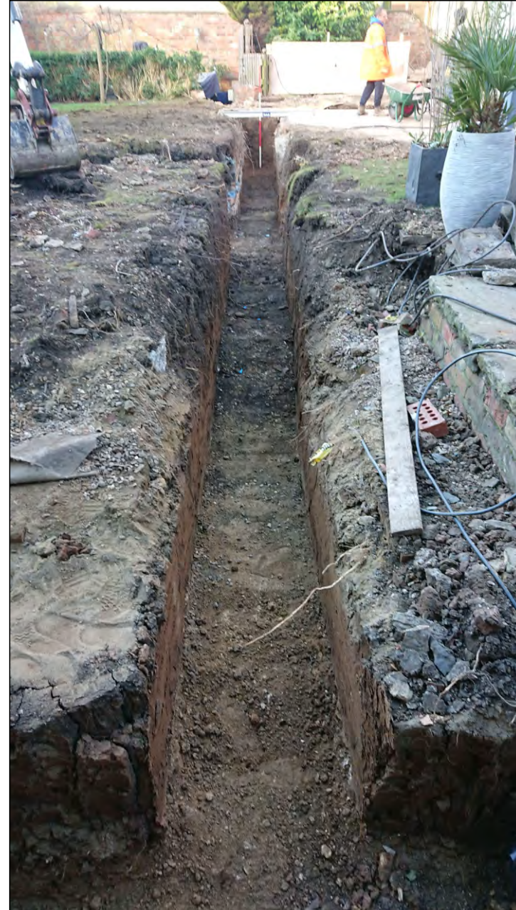
Photo 04. Foundation trench B-A, view looking west.
