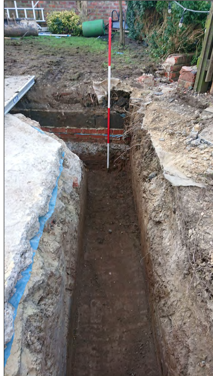
Photo 10. Foundation trench C-A, view looking south.
