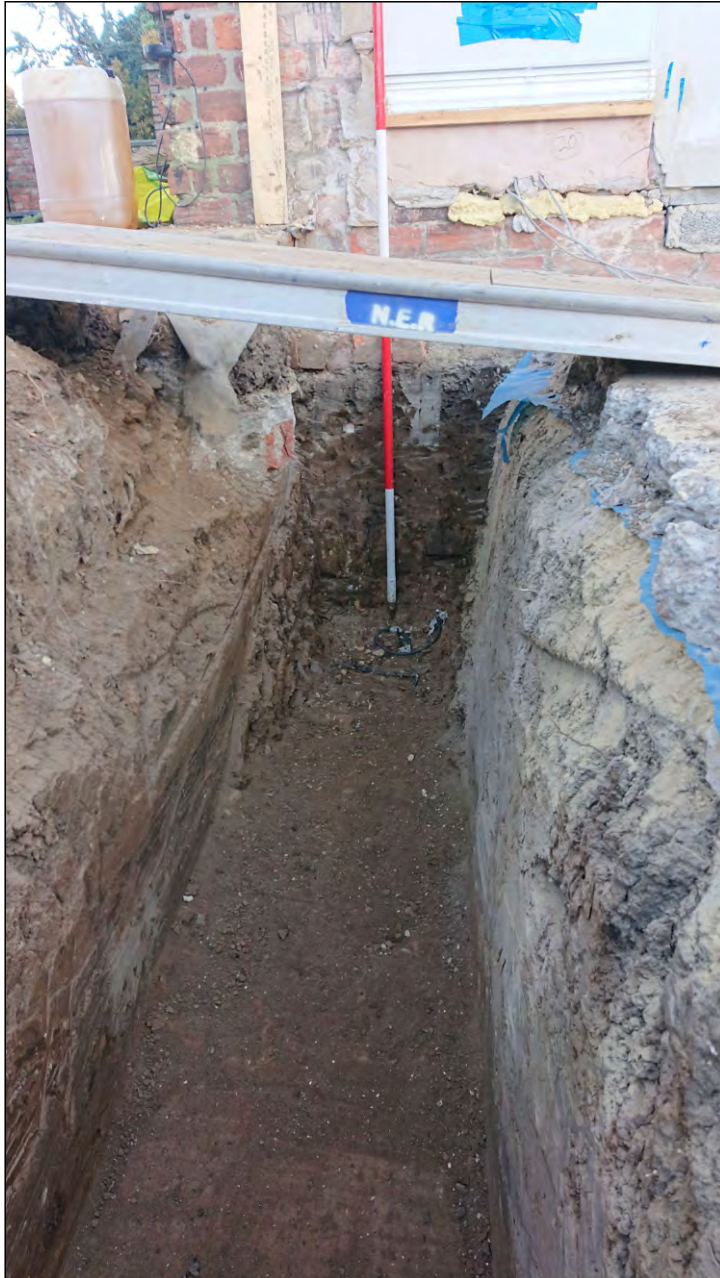
Photo 09. Foundation trench A-C, view looking north.
