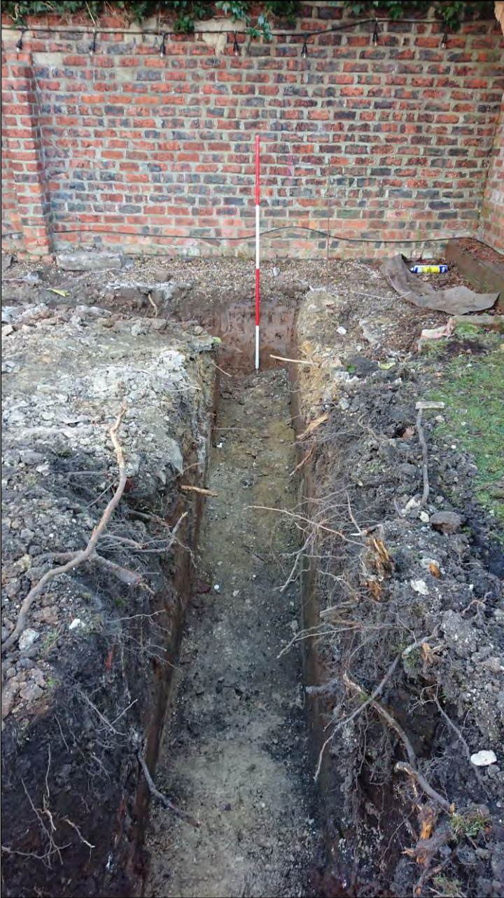
Photo 15. Foundation trench F-G, view looking east.
