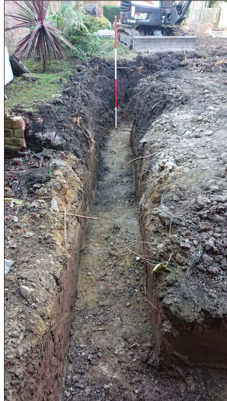
Photo 12. Foundation trench G-F, view looking west.
