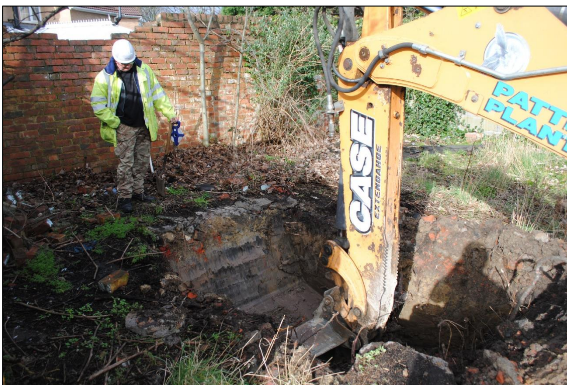
Frontispiece: Working shot of Trench 2 being excavated.
