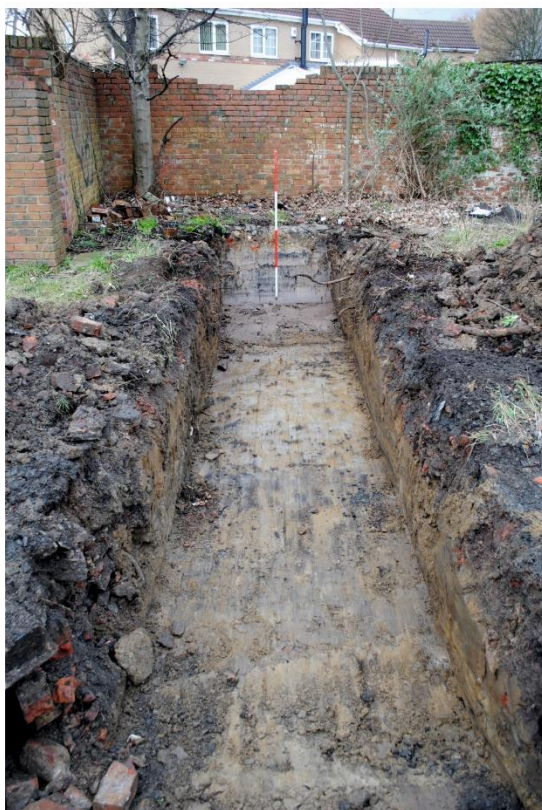
Photo 05. Trench 2 looking west
