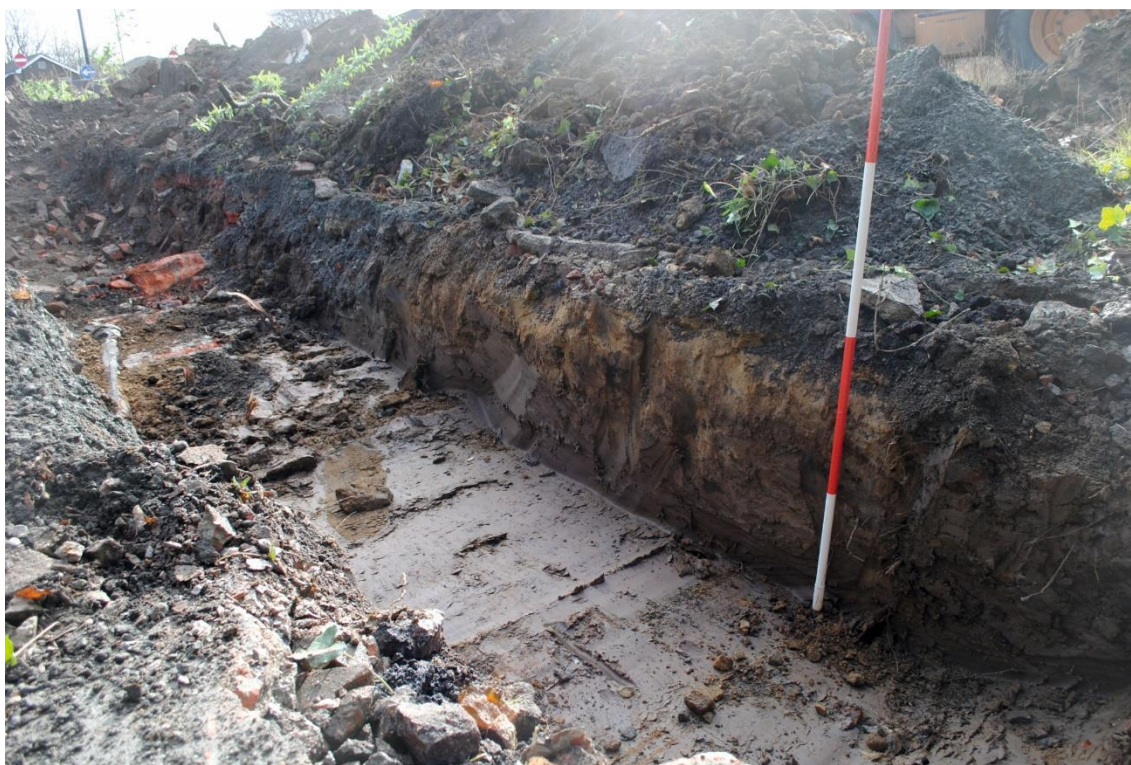
Photo 04. Trench 1 north-facing section, looking south-west, showing disturbance caused by Carville Hotel building and services towards eastern end of trench
