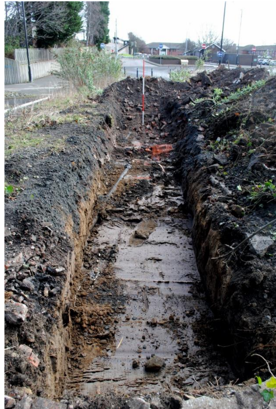
Photo 02. Trench 1 looking east
