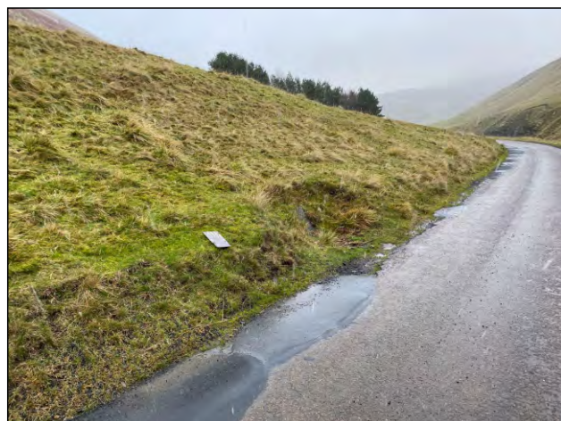
Photo 175. U4c. South end looking south
