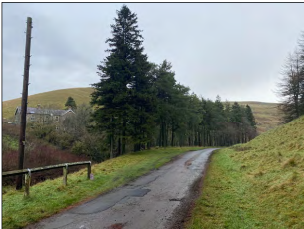
Photo 166. U2a. HV - looking NE
