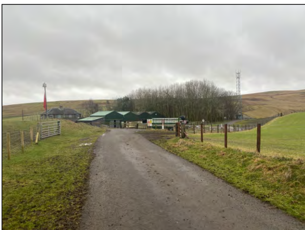
Photo 204. U13. Quickening Cote Mast
