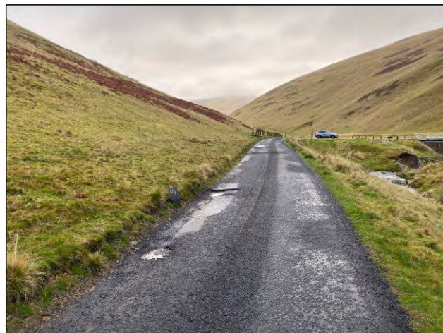
Photo 173. U4a. North end looking SSE
