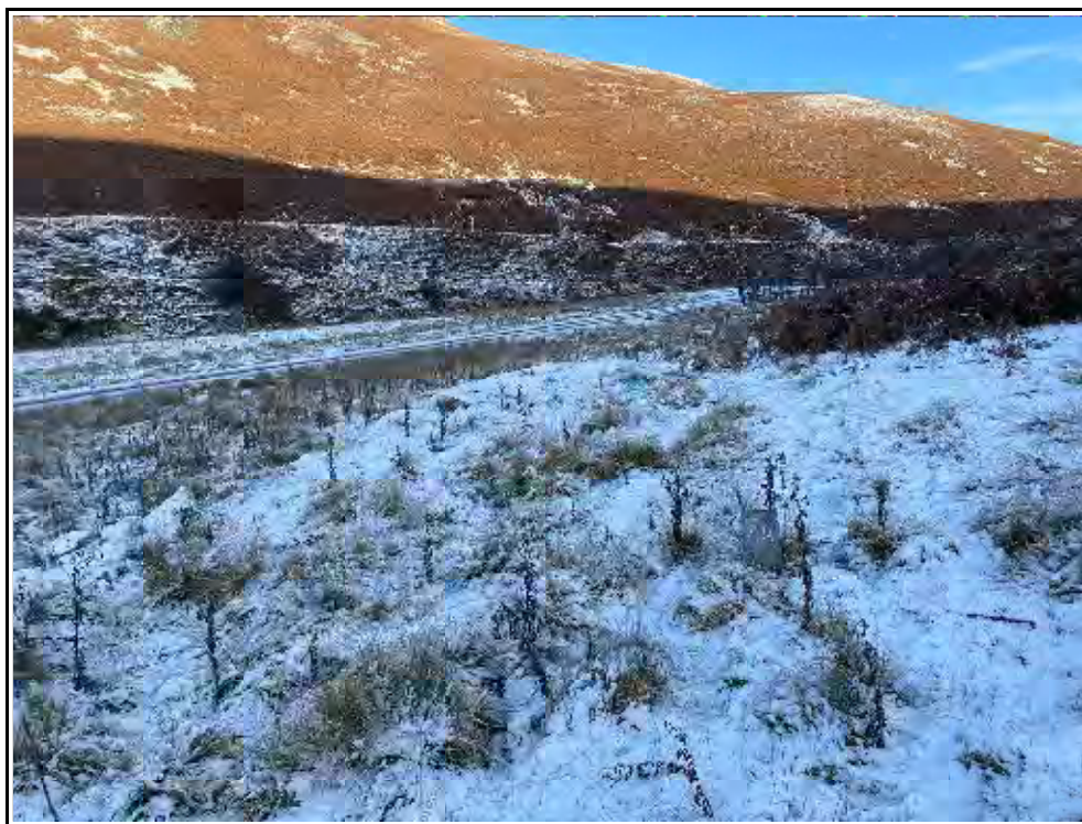
Frontispiece: Earthworks adjacent to Pole Site 74 below Bygate Hall.
