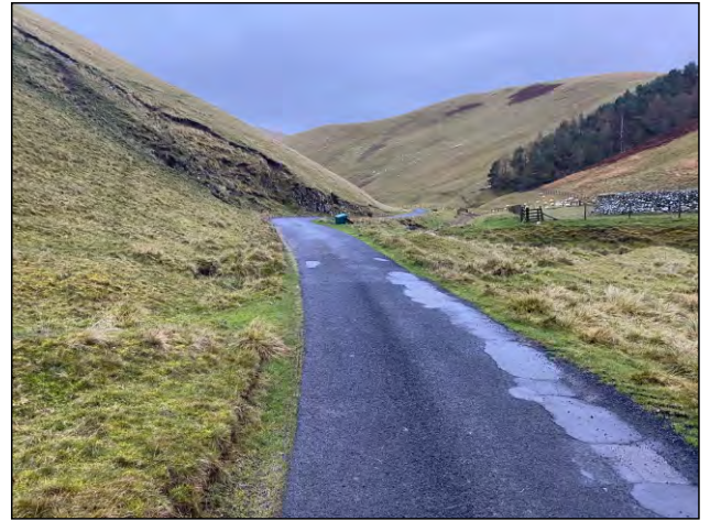
Photo 189. U9b. View looking south
