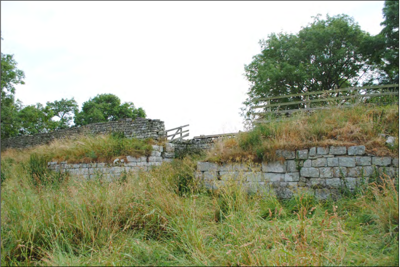
Photo 1. View looking WNW towards the west gate of Bremenium Roman Fort, prior to excavations for an interpretation panel.
