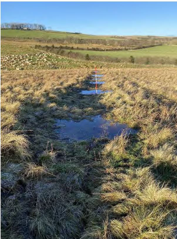
Photo. 10: Ground-level view of groundworks on N-S grips to create dams and small ponds across a grip in the west part of the site.
