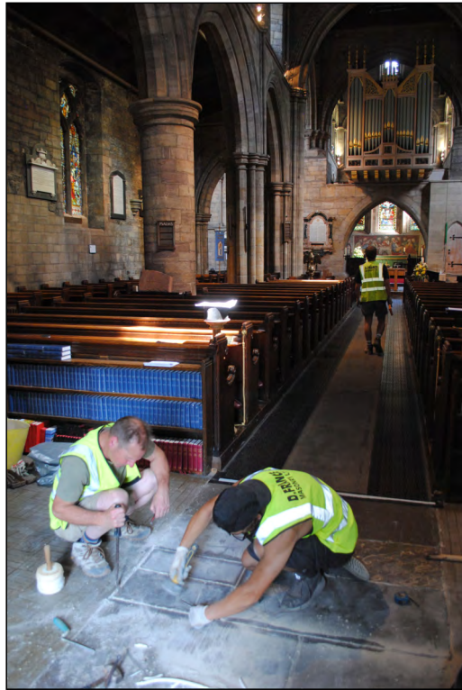
Photo 09. Test Pit 2, view looking east during removal of flags.
