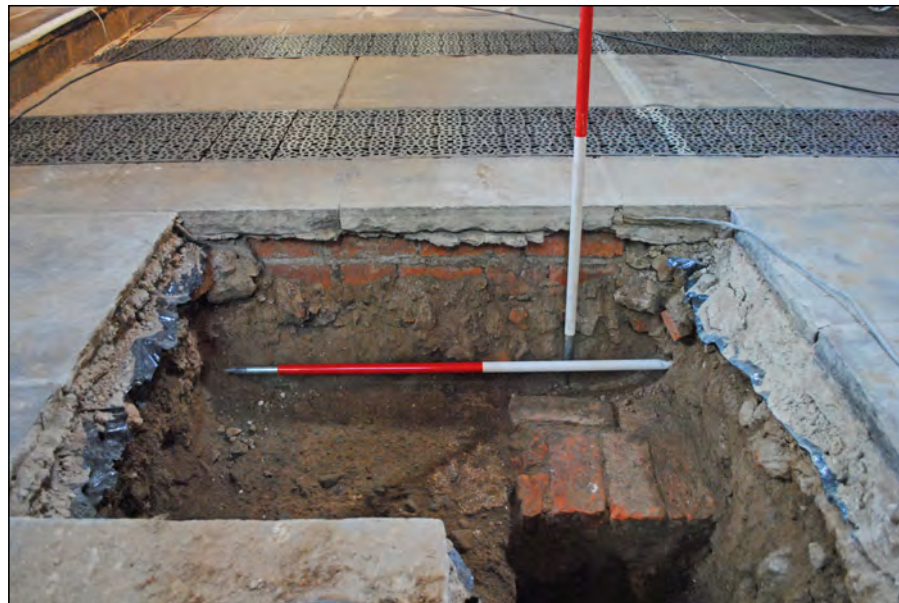
Photo 07. Test Pit 1, south view, showing north-facing section and partially truncated C18/19 brickwork and concrete below the floor.
