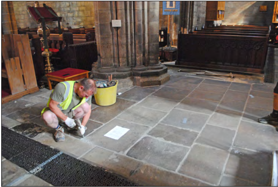
Photo 01. Test Pit 1, view looking north-west during the removal of flags in the crossing.
