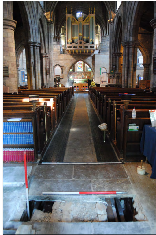
Photo 10. Test Pit 2, broad view looking east down the central aisle after removal of flags.
