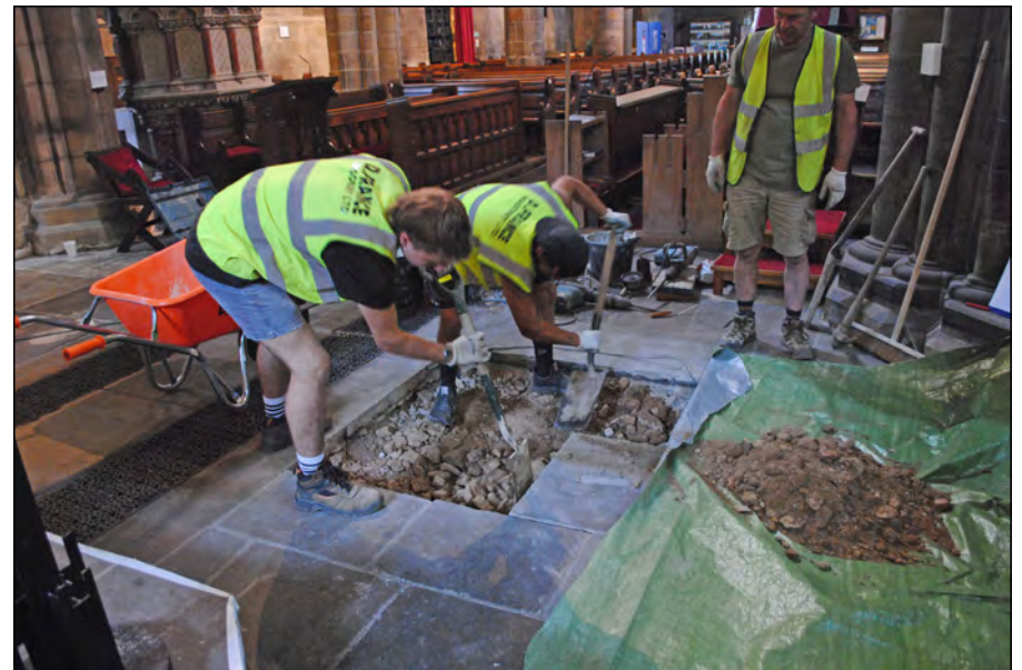
Photo 04. Test Pit 1, south view, removal of concrete after breaking.
