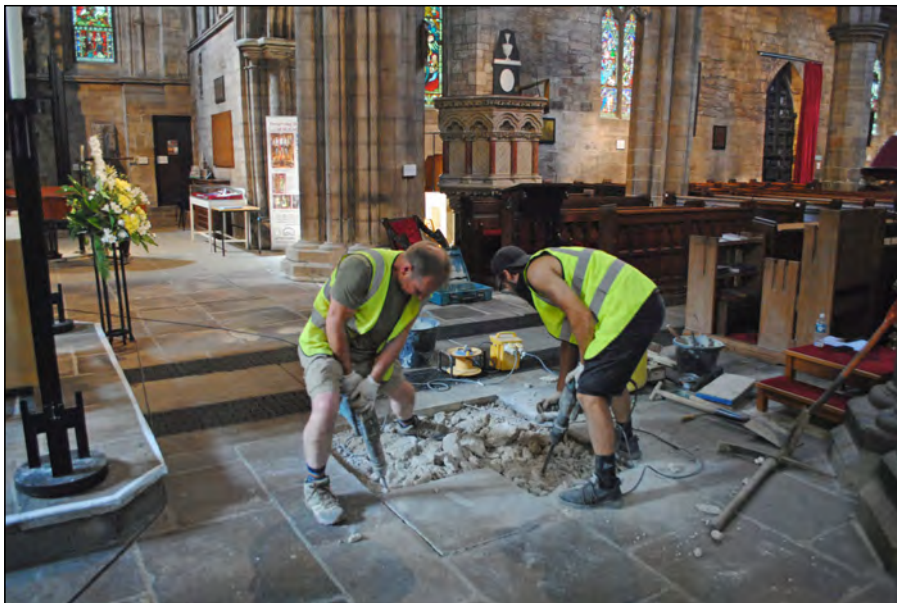
Photo 03. Test Pit 1, south-west view during concrete breaking.
