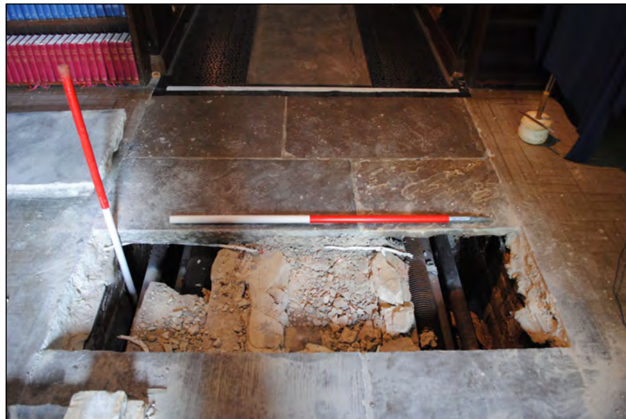
Photo 11. Test Pit 2, detailed view looking east at exposed pipework, revealed after removal of flags.
