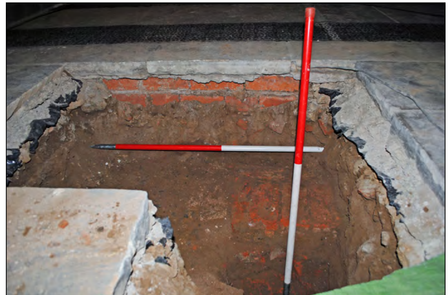
Photo 08. Test Pit 1, south view (with flash), showing depth of truncation in C18/19 brickwork and concrete below the floor.
