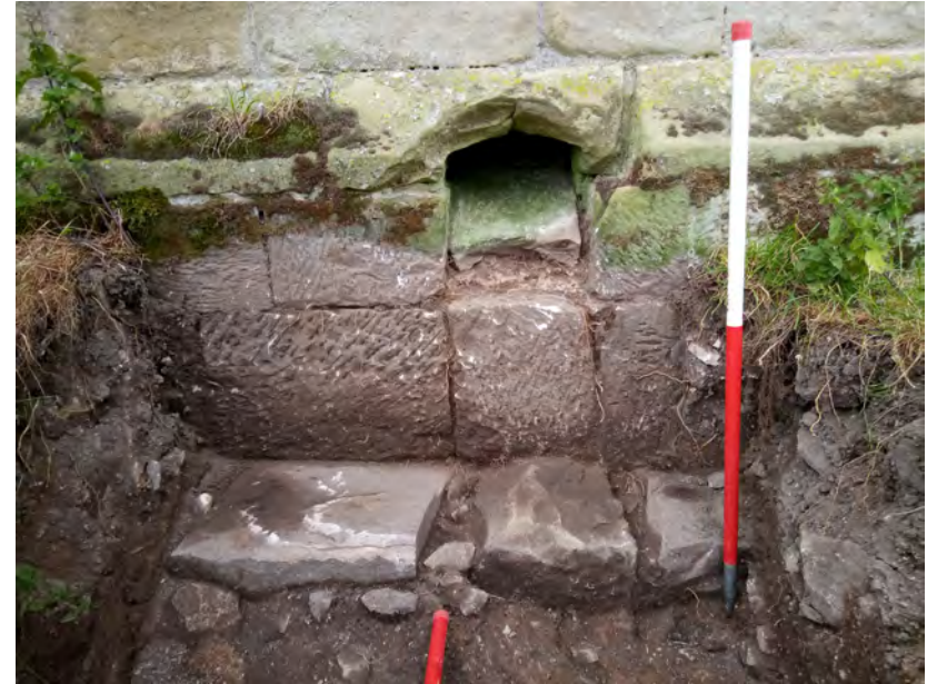
Illus. 13b: Trench L looking S showing offset wall foundation
