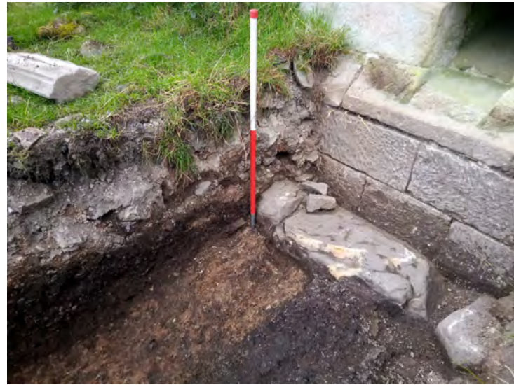
Illus. 14b: Trench L looking SE showing offset foundation
