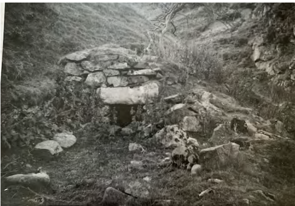
A malting kiln used in the production of whiskey at Rory's Still, Upper Coquetdale (unpublished photo. Taken in 1956 by Captn. Walton, used courtesy of BrightWater volunteer, Barbara McCabe)
