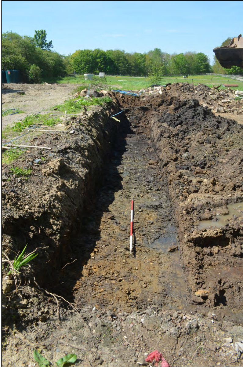
Photo 05. View looking west along south trench, following excavation to finished depth.
