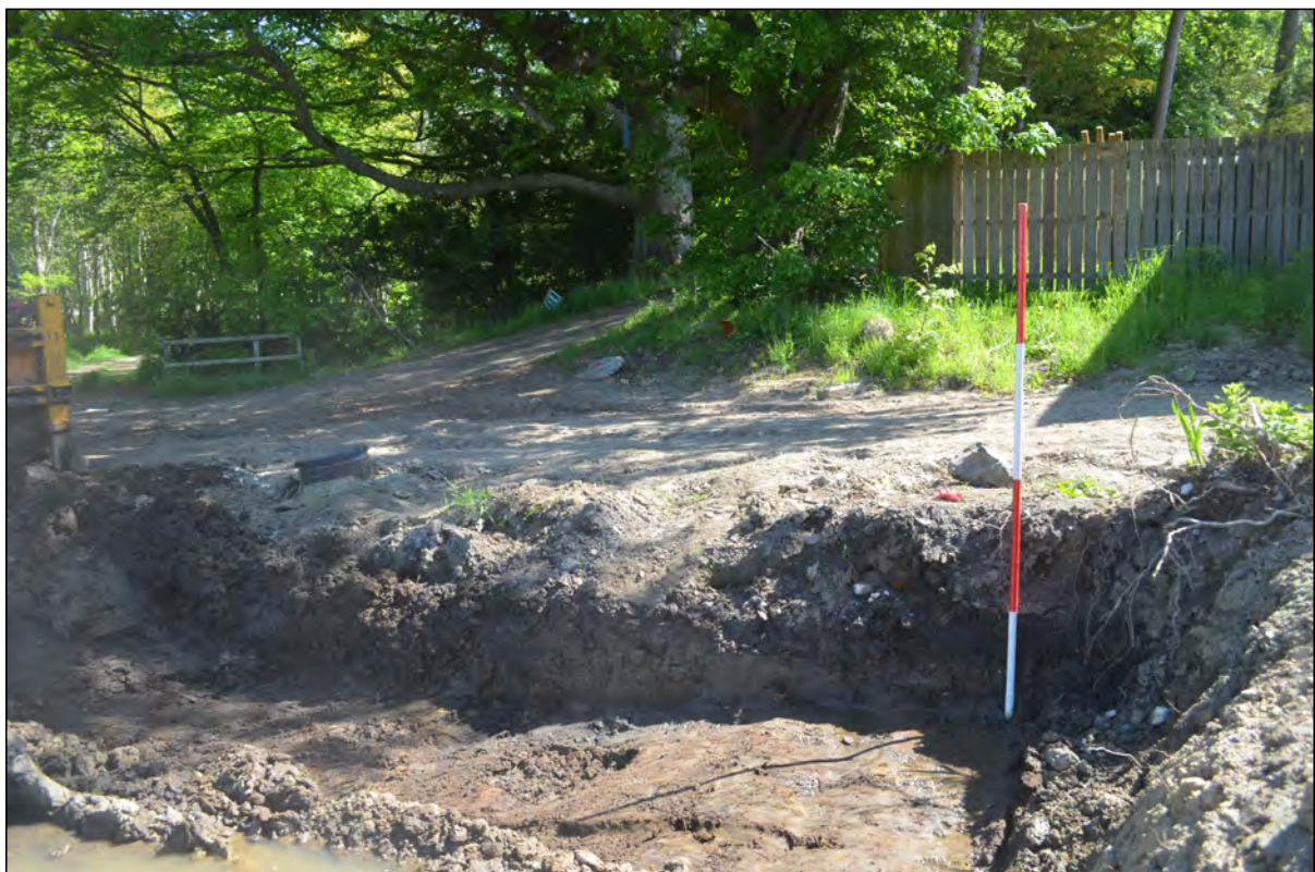
Photo 04. West facing section of east trench, following excavation.
