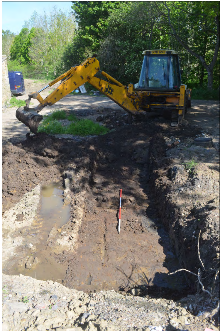
Photo 03. View looking north along the east trench, following excavation.
