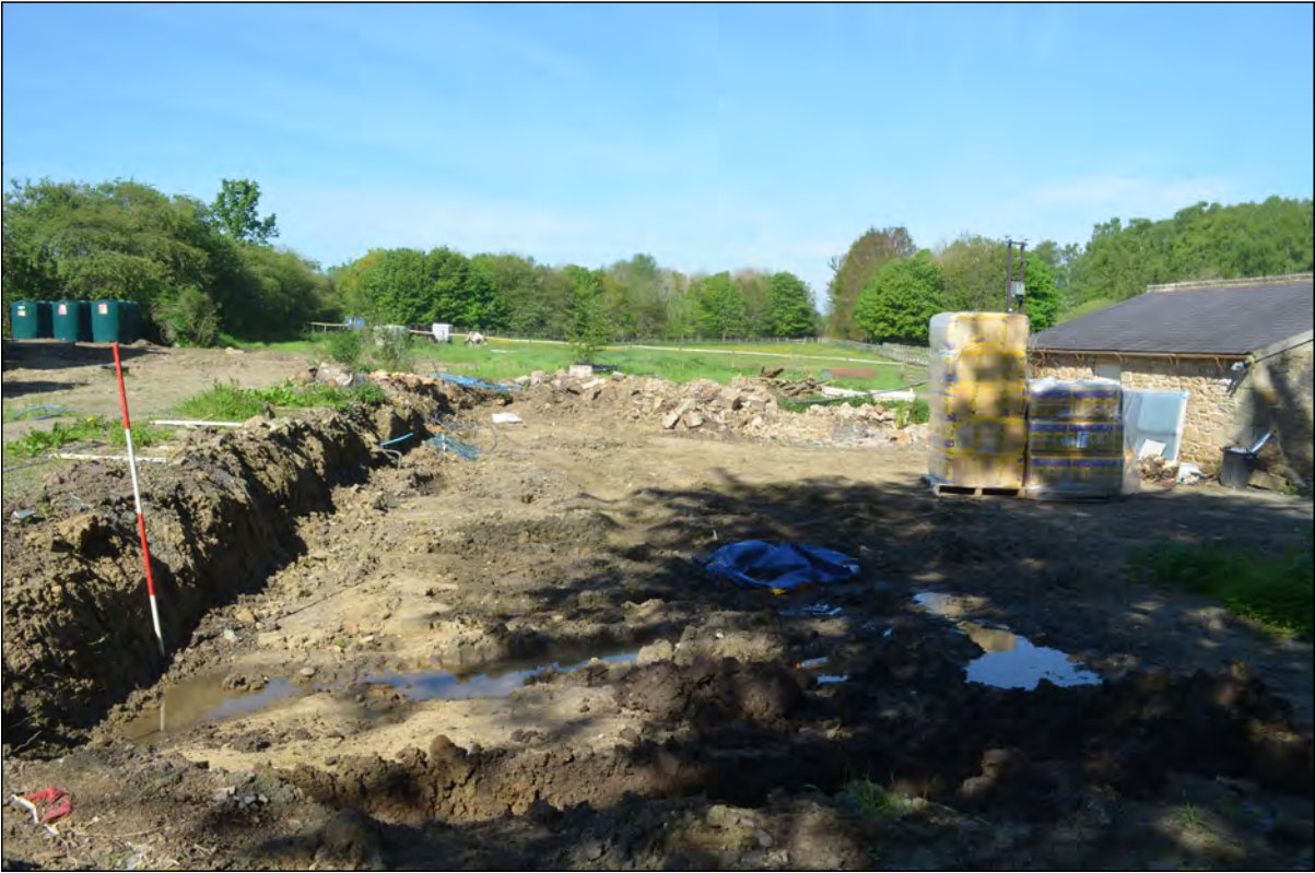
Photo 01. Pre-excitation shot. View looking west following demolition of the Pole Barn.
