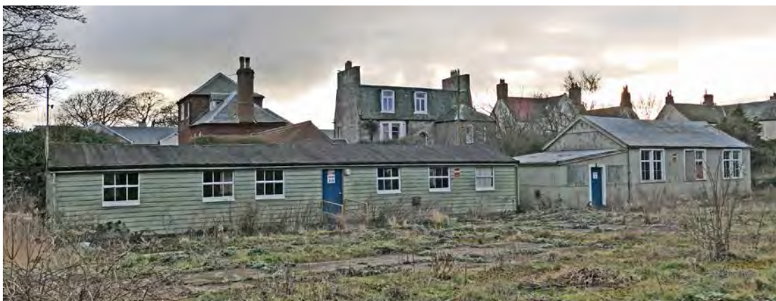
Illus. 13: View from the east of the detached classroom buildings in the rear yard.
