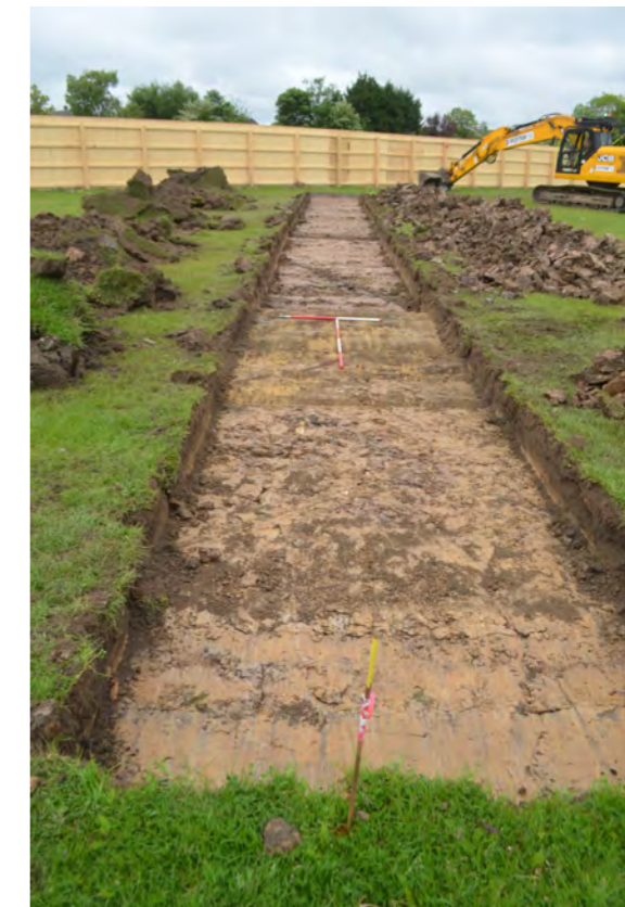
Overview shot of T21, looking SW.
