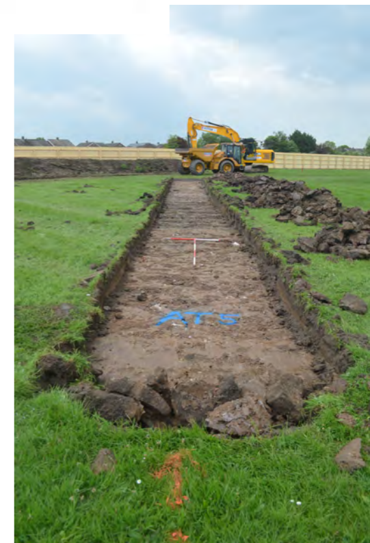
Overview shot of T16, looking SW.
