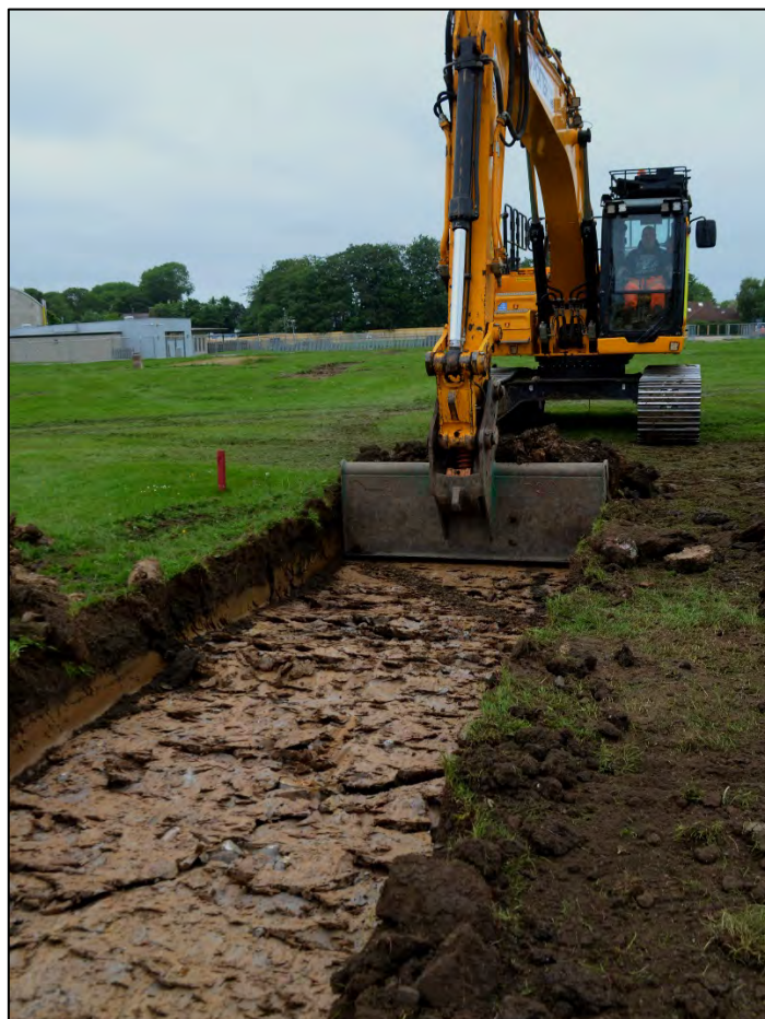
Frontispiece: North view, working shot, Trench 22.
