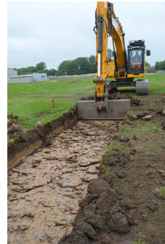
Working shot showing the excavation of T22.
