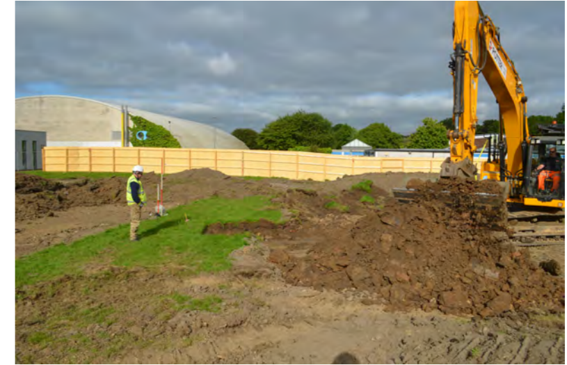
Working shot of the excavation of T3.
