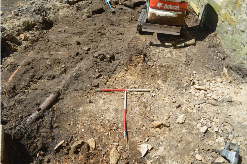
Photo 03. View looking west showing the area of ground reduction.
