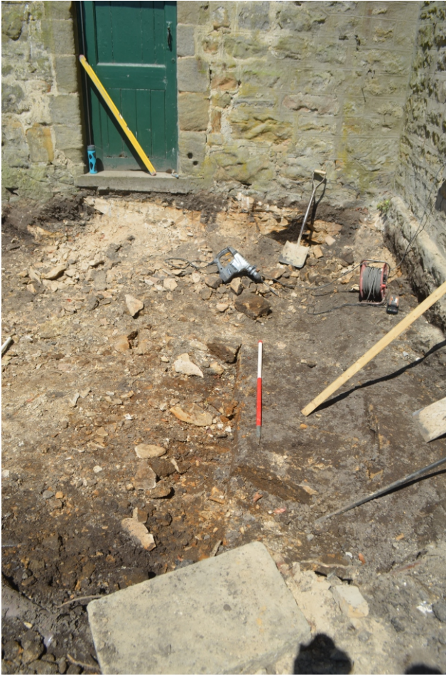
Photo 05. View looking north of the east end of the ground reduction.
