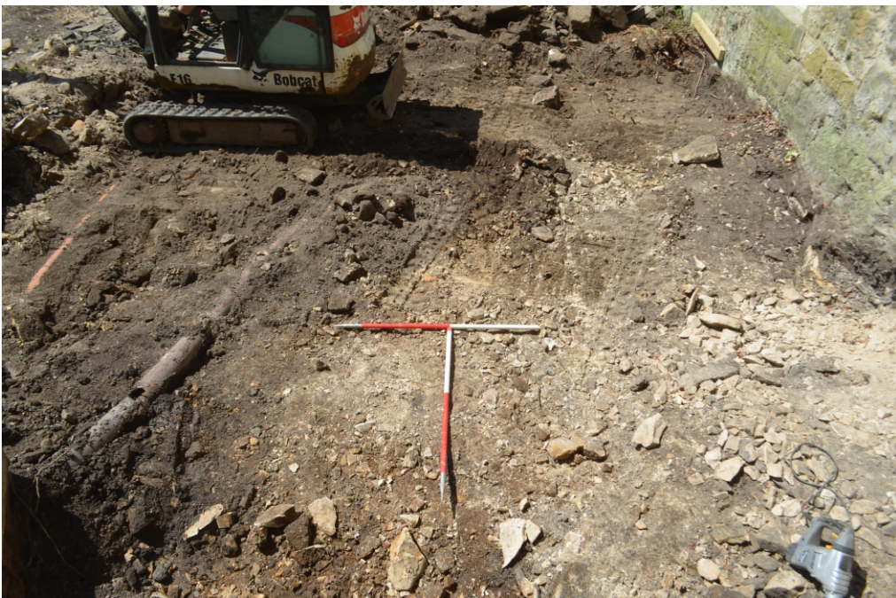
Photo 04. View looking west showing the area of ground reduction.
