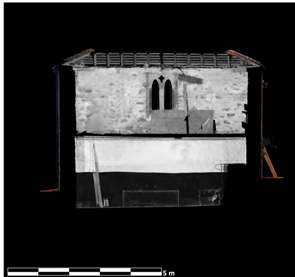
Illus. 23: Digital Scan of the north-facing internal face of the south end wall of the West Range, Shield Hall, processed by Gianluca Foschi, April 2022.
