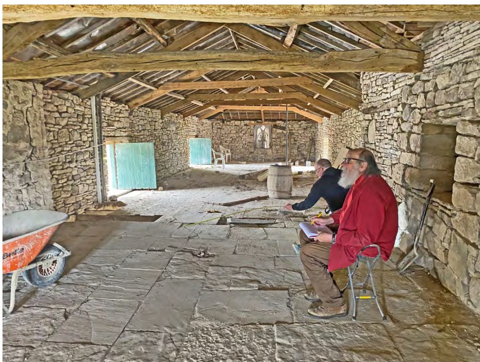
Illus. 11: Recording the upper floor and internal walls of the cross-wing prior to consolidation works.
