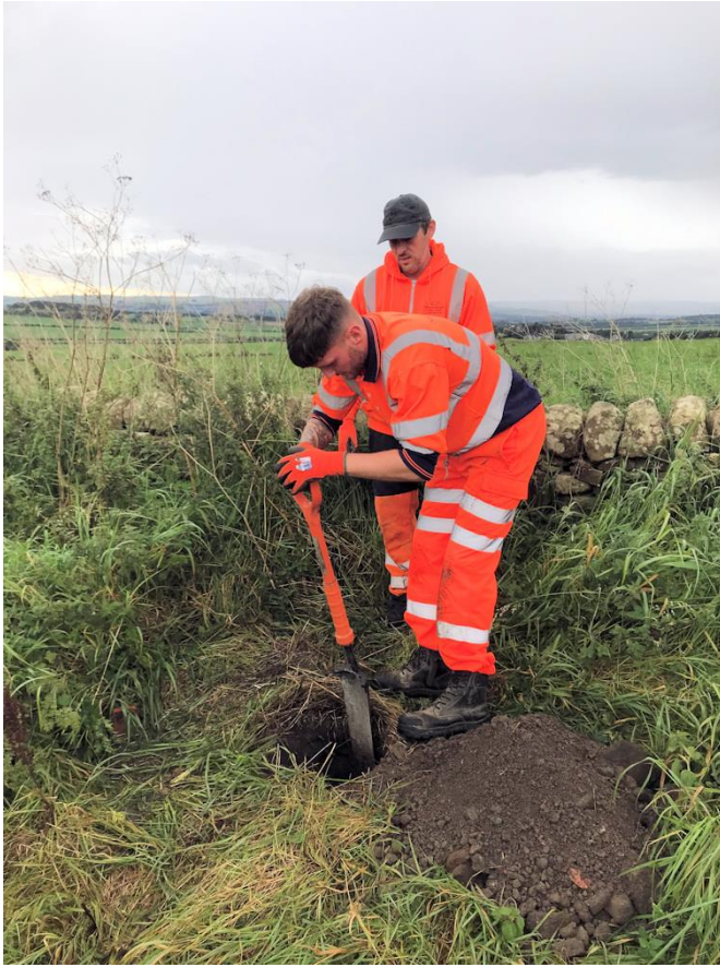
◀ Photo. 03: Hand excavating foundation pit in progress, looking southwest.
