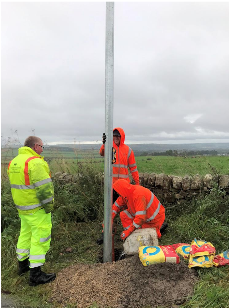
◀ Photo. 08: Installation of signpost in progress, looking southwest
