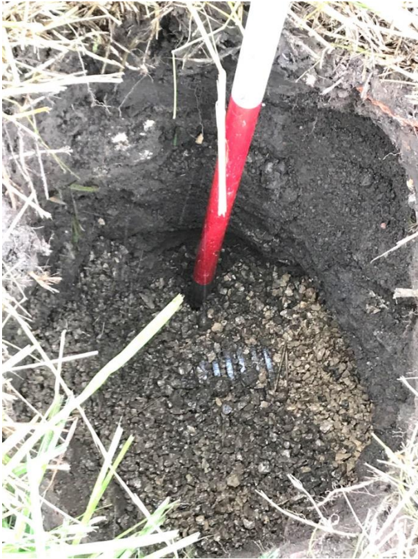
◀ Photo. 05: Top of plastic utility pipe [04], packed with gravel [03], looking southwest.
