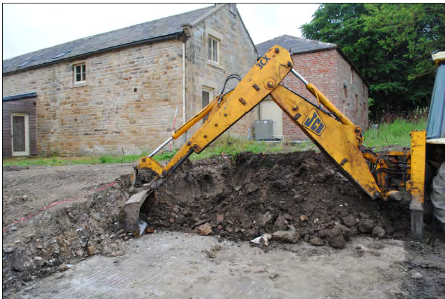
Photo 03. View looking south-east during landscaping works.
