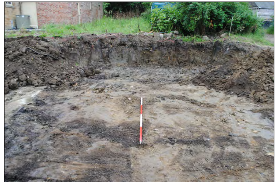
Photo 07. View looking south at landscaping works (2 metre scale at centre).
