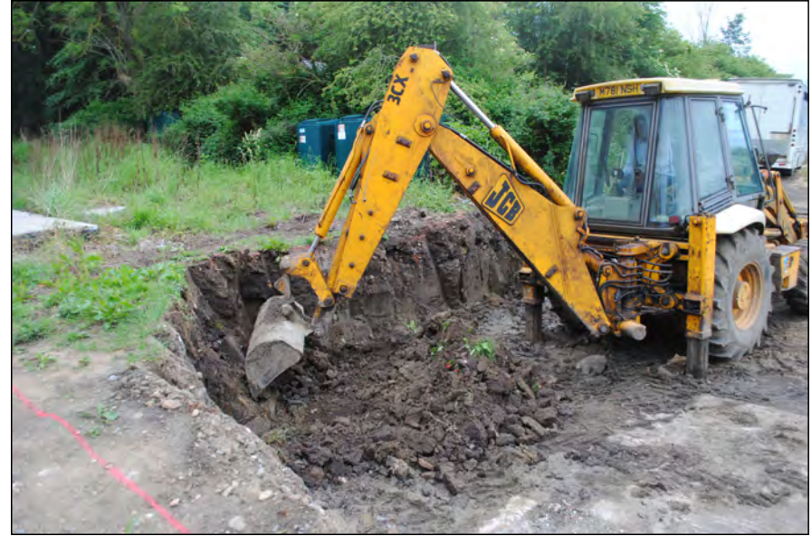
Photo 02. View looking south-west during landscaping works.
