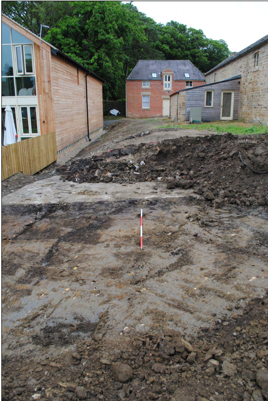
Photo 05. View looking east at landscaping works (2 metre scale at centre).
