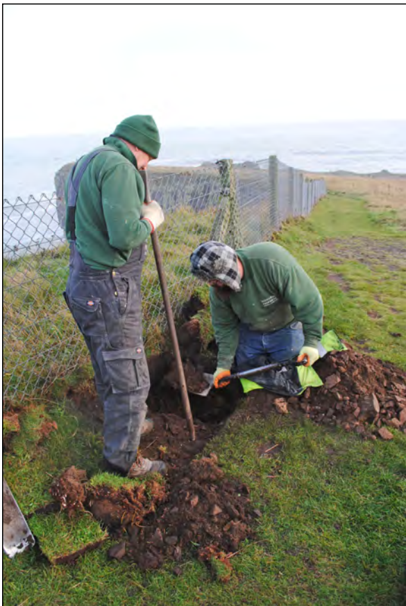
Photo 13. View looking northeast during final stages of excavation for Test Pit 1.
