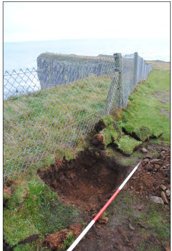
Photo 14. View looking northeast at completed excavation for Test Pit 1.
