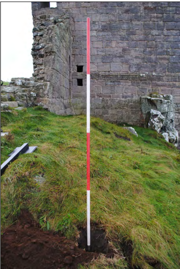
Photo 6. View looking SSW at completed excavation on the north side of Lilburn Tower.
