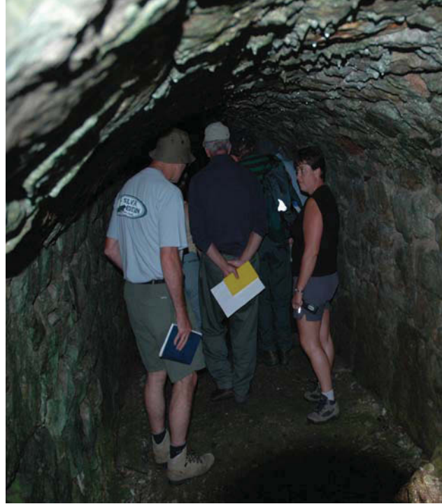
Plate 5: detail of tunnel shown in Plate 4
