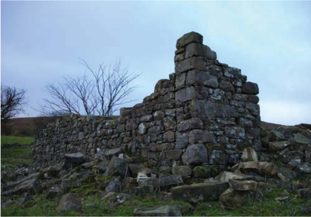
Plate 45: NE corner of farmhouse
