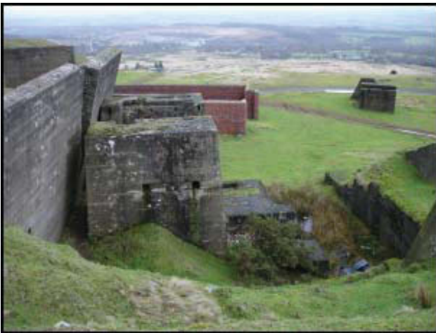
Plates 218-223: The building complex at the ropeway terminal. The substantial stone and concrete pylons in the top images were the supports for the crushing plant. Other structures relate to the secondary ropeway which carried stone from the quarry to the main ropeway loading head. The purpose of the brick building in the middle images is uncertain. It is at present being used as a winter feeding station for sheep with some resultant poaching of the areas around the buildings.
