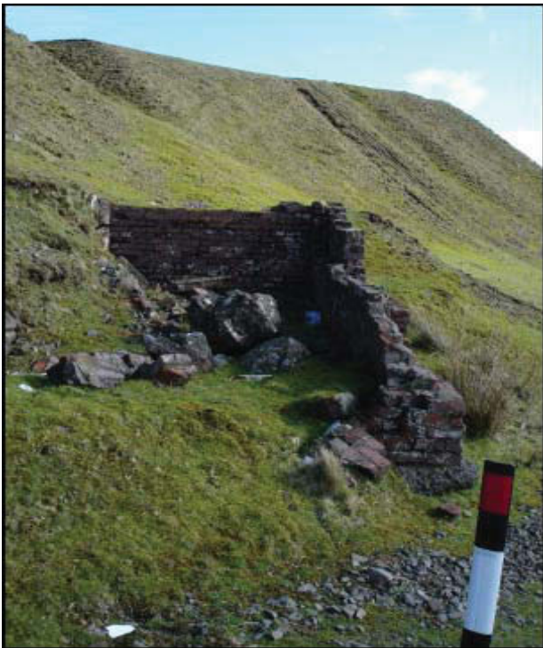
Plates 39-41: Two buildings centred at SO 5947 7759 at the head of Dhustone Lane Quarry approach. The lower is built of brick, the higher of dressed stone
