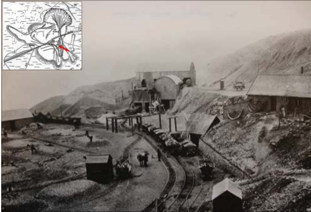
Plate 11: Sidings at the top of the main incline c.1903, seen from the SE
