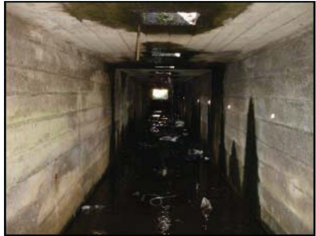
Plates 48-49: Tunnel running from cutting in the east at SO 5933 7741 to SO 5928 7743 in west. The concrete capped tunnel is probably designed to protect a tub line from the spoil field above
