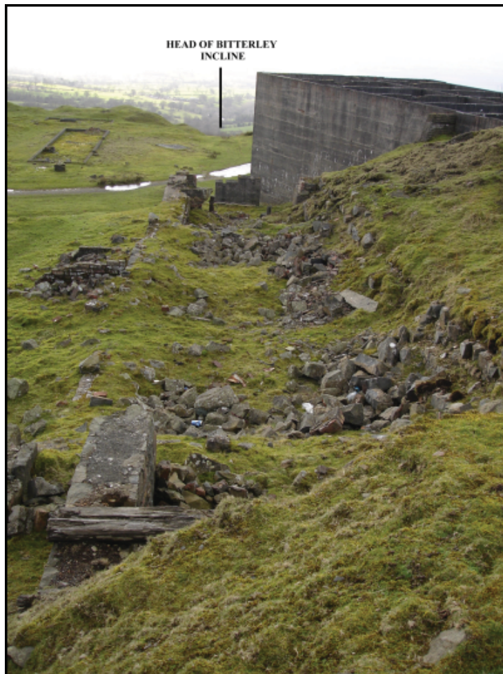
Plate 1: Looking along the line of the 1884 building towards the incline head
