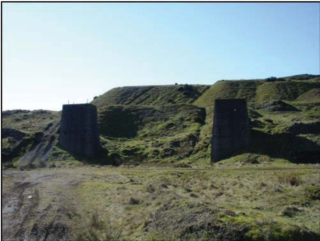
Plate 183: The site today, the two pylons survive intact, the central building is a foundation only Located at SO 6146 7752
