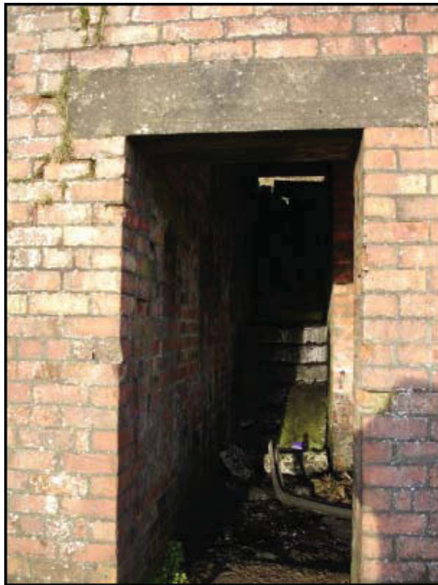
Plates 144-149: Brick chamber built beneath upper rail line at SO 5891 7605. Top right shows concrete and RSJ roof structure. Bottom shows stairs linking to open inspection chamber in top of rail embankment. Doorway now blocked with bricks.
