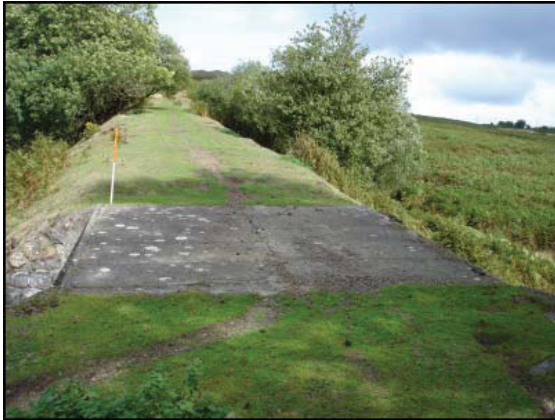
Plates 84 and 85: Left the concrete crossing plinth and right the stone abutments
