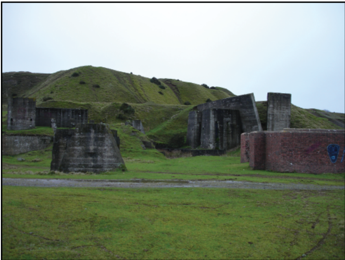
Plate 187: The secondary ropeway complex as it survives today
