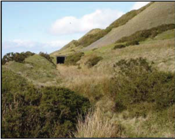
Plates 48-49: Tunnel running from cutting in the east at SO 5933 7741 to SO 5928 7743 in west. The concrete capped tunnel is probably designed to protect a tub line from the spoil field above
