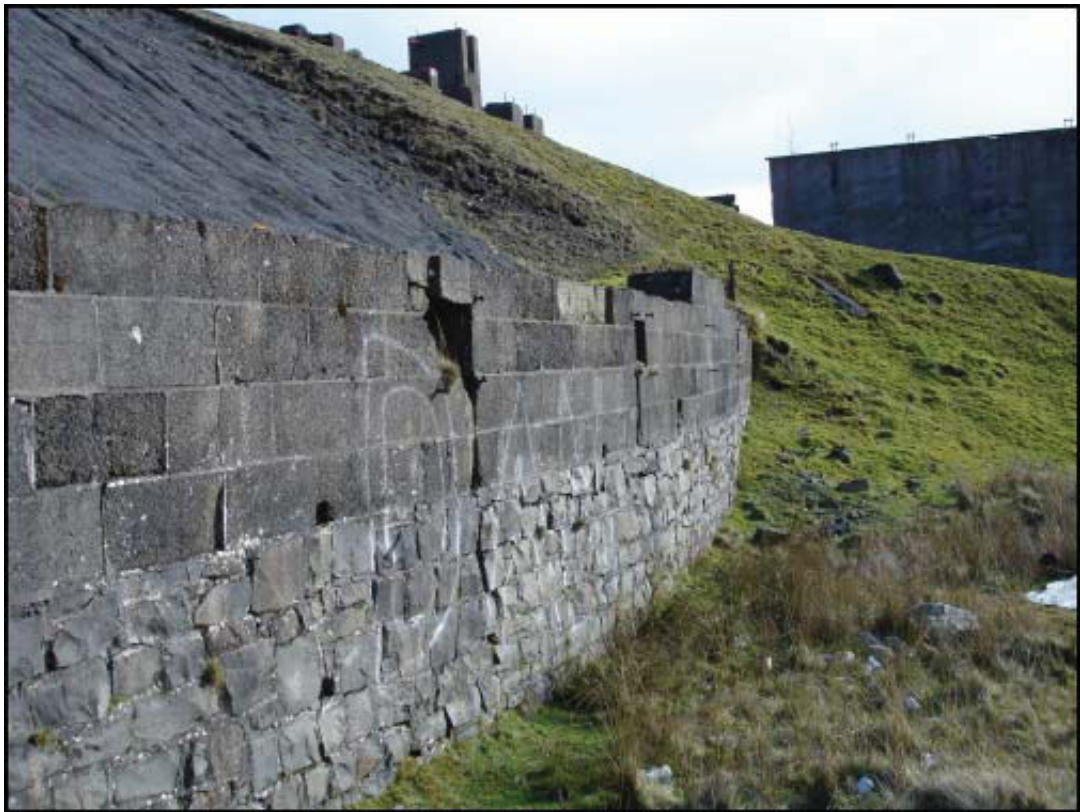
Plate 9: Stone revetments at the bottom and top of slope survive today
