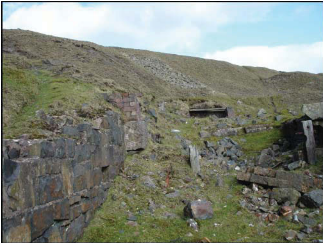
Plate 4: The north side of the building, built into the hill slope
