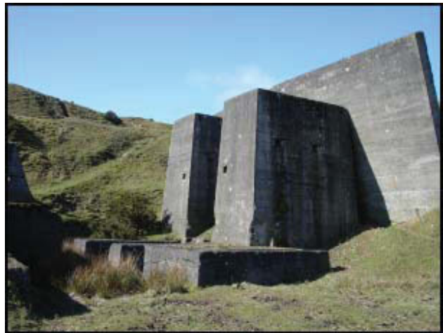
Plates 218-223: The building complex at the ropeway terminal. The substantial stone and concrete pylons in the top images were the supports for the crushing plant. Other structures relate to the secondary ropeway which carried stone from the quarry to the main ropeway loading head. The purpose of the brick building in the middle images is uncertain. It is at present being used as a winter feeding station for sheep with some resultant poaching of the areas around the buildings.
