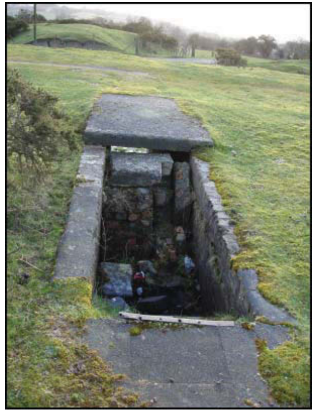
Plates 144-149: Brick chamber built beneath upper rail line at SO 5891 7605. Top right shows concrete and RSJ roof structure. Bottom shows stairs linking to open inspection chamber in top of rail embankment. Doorway now blocked with bricks.
