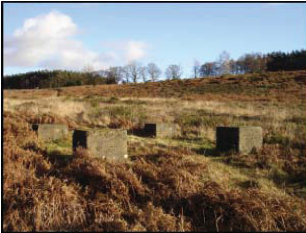
Plates 224-228: The top image shows the approximate line of the ropeway from its terminal on Magpie hill running out across Catherton Common. The middle left image shows the very substantial base of a terminal pylon at SO 6155 7745. The other images show examples of the concrete pylon bases that survive along the course of the ropeway.
