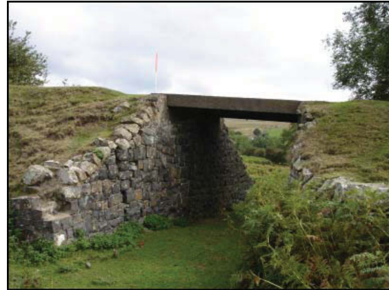
Plates 84 and 85: Left the concrete crossing plinth and right the stone abutments
