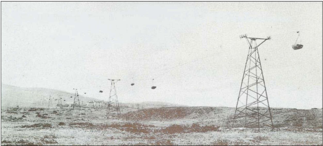
Plate 180: Aerial ropeway in operation running across Catherton Common, Magpie Hill in the distance (Photo courtesy of A Jenkins)
