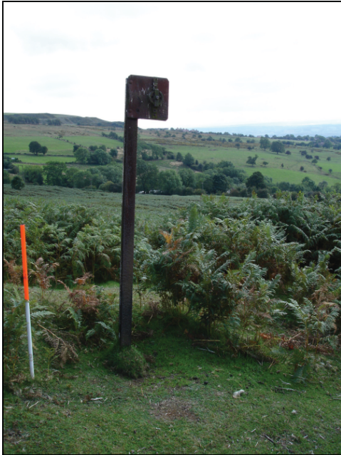
Plate 79: SO 59018 77506 length of rail supporting pulley
