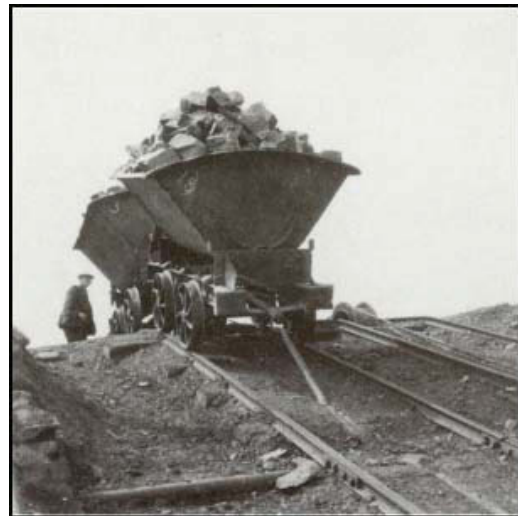
Plates 102-103: Tubs climbing the Dhustone Quarry incline; stone setts at the head of the incline
