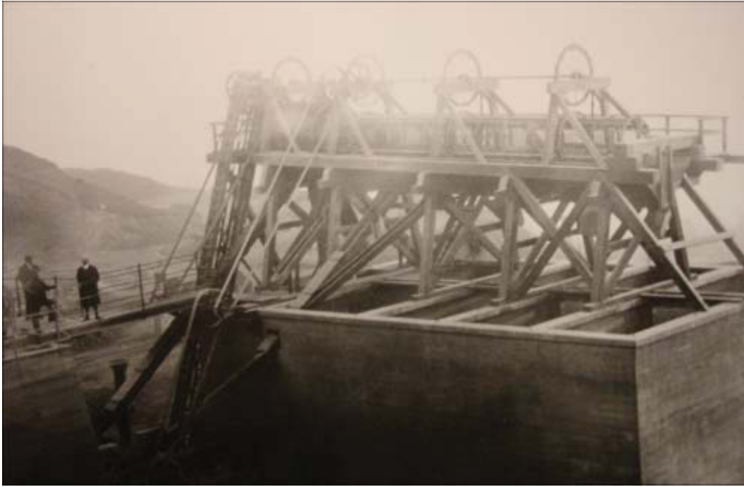
Plate 20: Early stone crusher, showing the exposed superstructure
