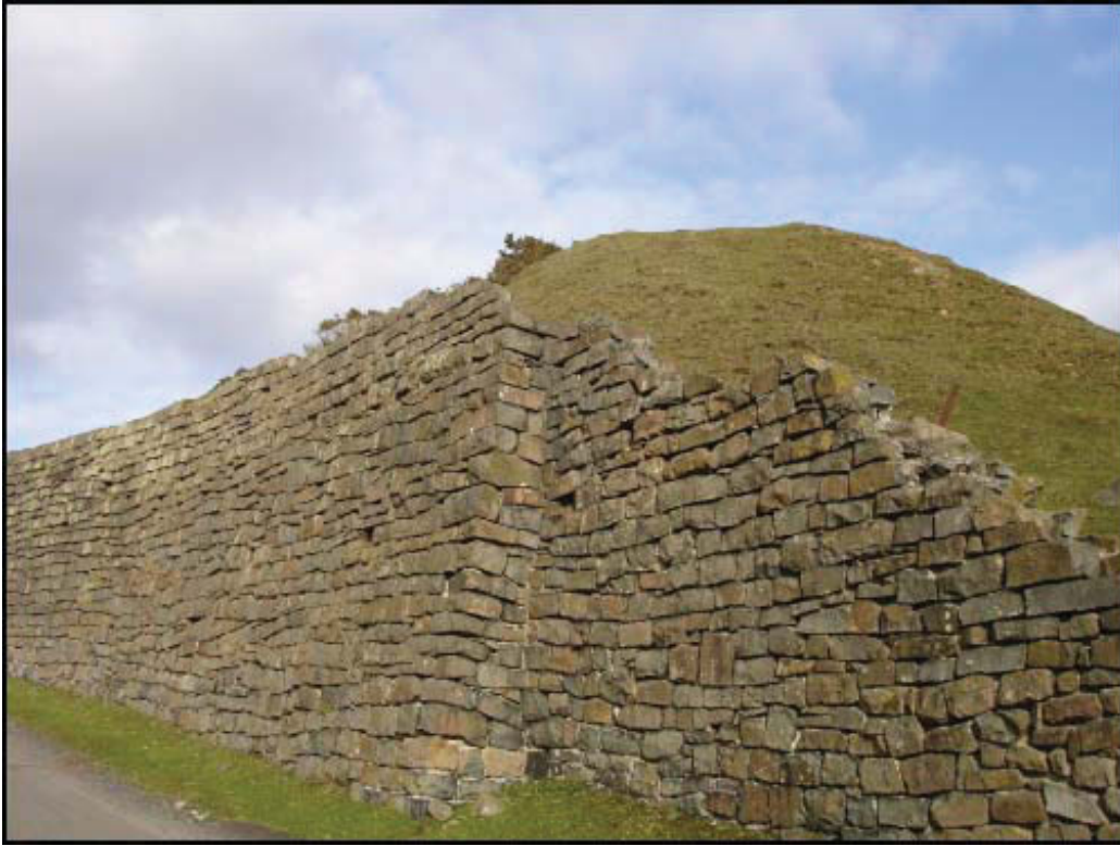
Plate 172: Stone built revetment wall below incline head located at SO 5953 7556
