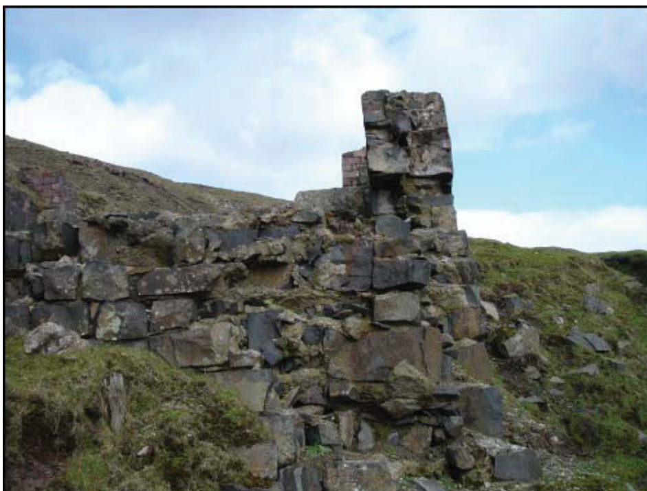
Plate 3: The south end of the building, showing exposed wall structure
