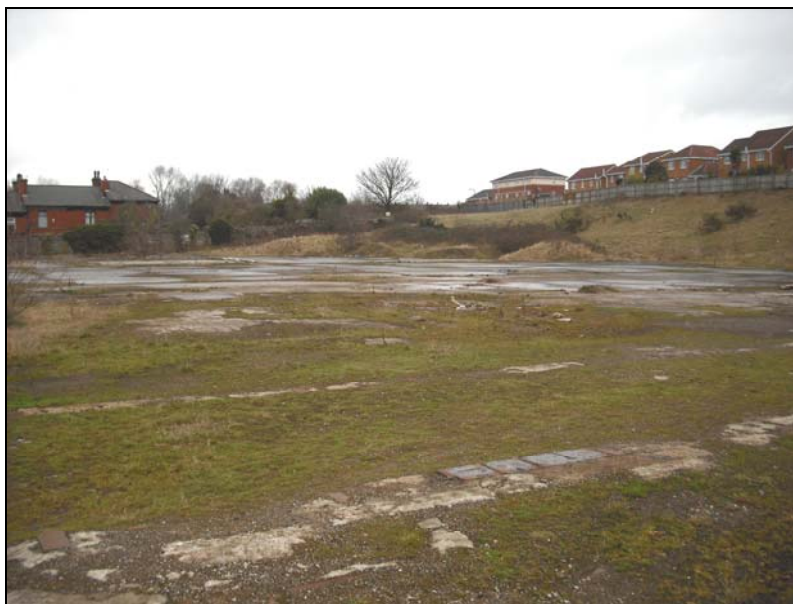
Plate 5 (10): the western area of the PDA with the building platform, from the west southwest
