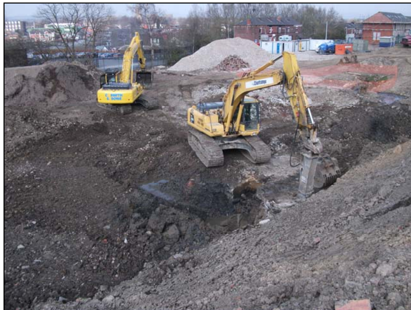
Plate 2, 5: general view of the excavations, looking north
