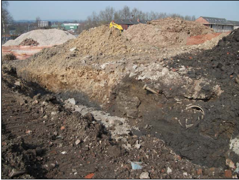
Plate 3, 11: Oblique view of the section through the dam, looking north
