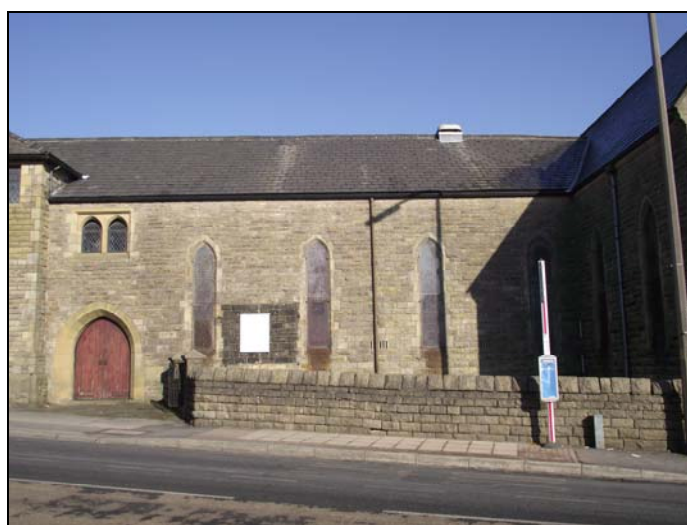
Plate 3, 22: view of the Nave's south elevation, from the south
