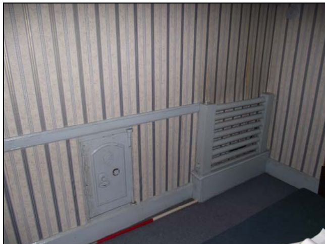
Plate 18, 153: Room 2, view of the safe and radiator to the west wall
