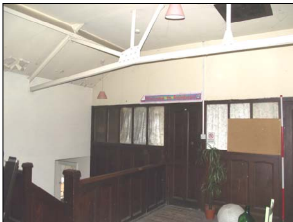
Plate 43, 112: View of the landing and staircase (Rm. 18) with exposed roof truss and half glazed timber partition, from the northwest
