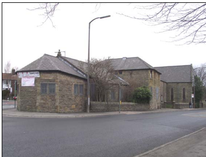
Plate 1, 15: general view of the church's west elevation, from the west southwest
