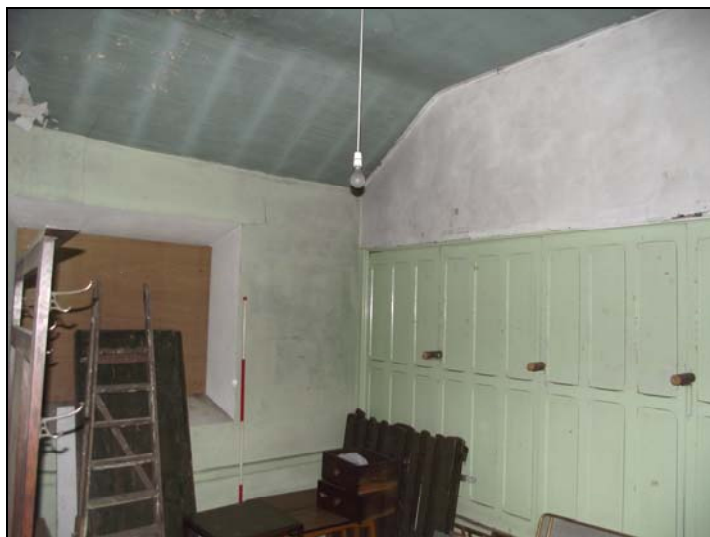
Plate 49, 124: General view with the balcony shutters closed (Rm. 26), from the southwest
