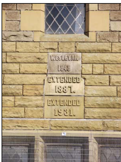
Plate 5, 17a: date stones to the south elevation, from the south
