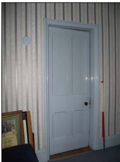
Plate 14, 155: room 2, detail of the 4 panelled doorway with stop chamfered decoration (c. 1870), from the south southwest
