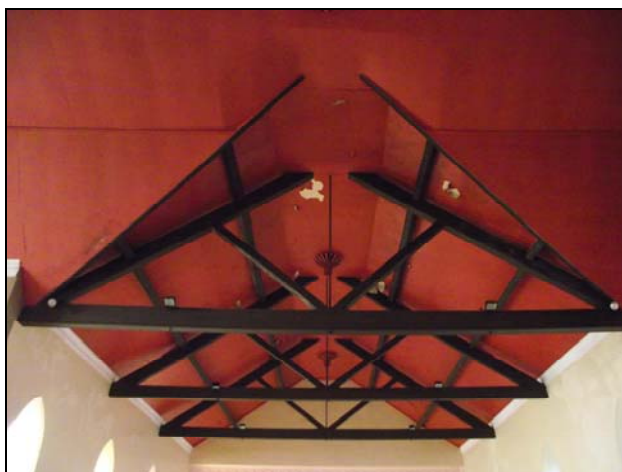
Plate 22, 76: room. 4a, view of the roof (exposed during the late C19th), from the east
