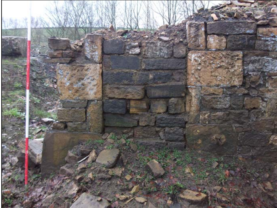
Plate 19, 50: Detail of doorway N (ground floor level) from the NNE
