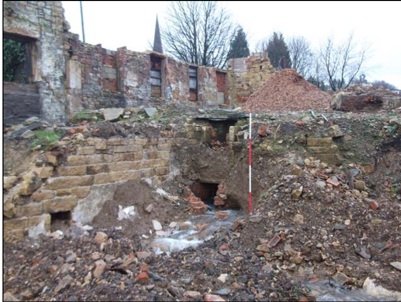
Plate 23, 35: View of the 'internal' walls of the phase 1 mill with later inserted brick culvert, from the south
