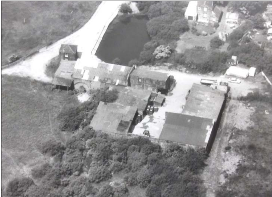
Plate 3: Aerial Photograph of the PDA c. 1980, from the east source: Greater Manchester Textile Mill Survey Archive
