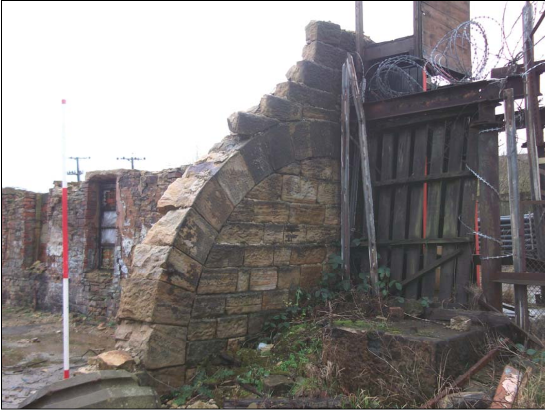
Plate 15, 15: Oblique view with the stone arch (opening M), from the northeast
