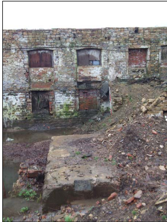
Plate 22, 38: View of the mass concrete machine base, from the southeast
