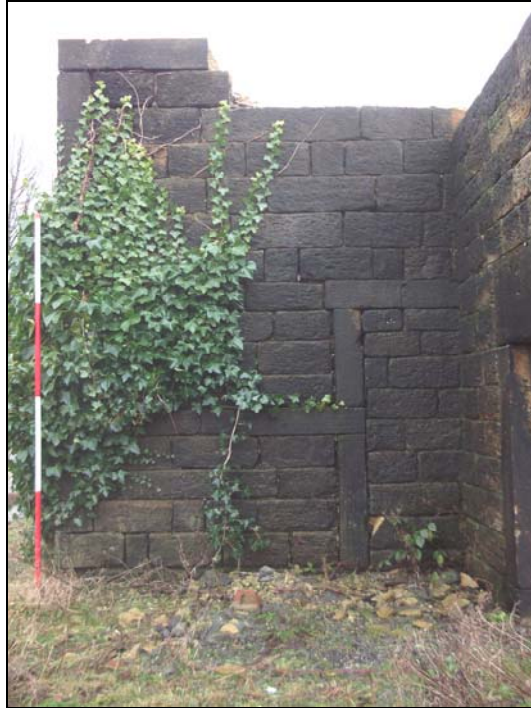
Plate 11, 10: view of the blocked doorway G, from the southwest
