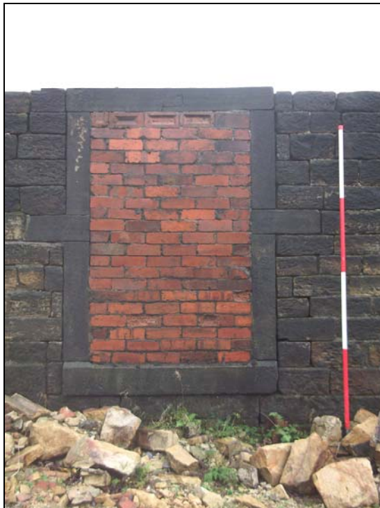
Plate 14, 13: detail of window J, from the northwest
