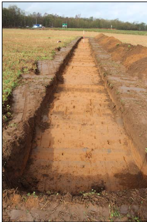
Plate 6: post-excitation view of trench 2, looking northwest
