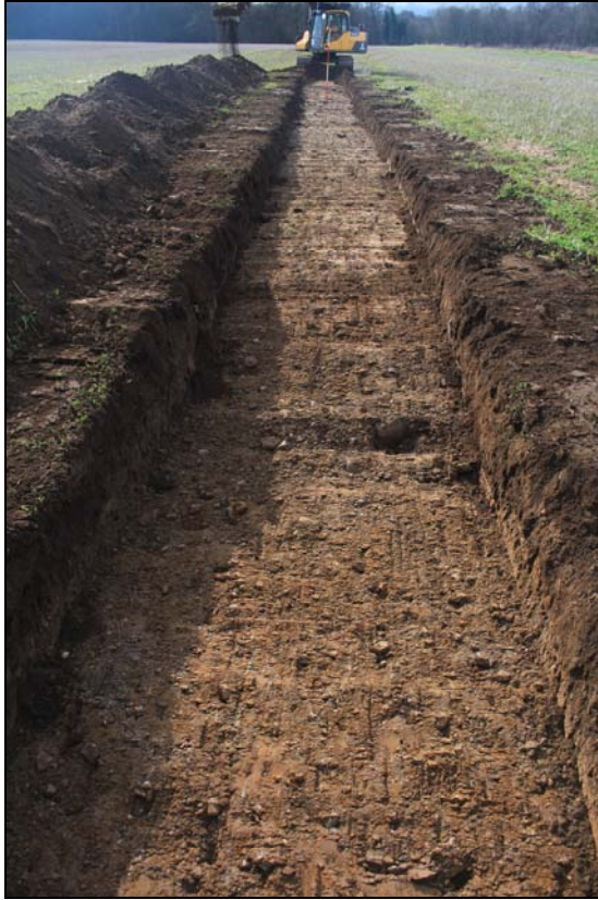
Plate 15: trench 9, general view looking west south-west
