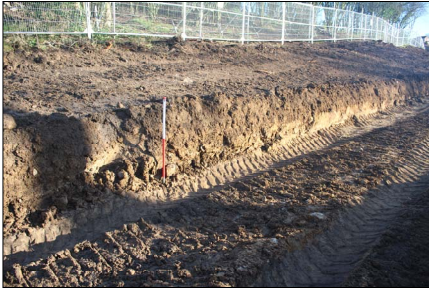
Plate 9: general view of the east-west access road with truncation of colluvial/glacial deposits, looking northeast
