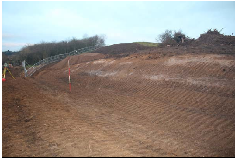
Plate 13: general view, looking northwest
