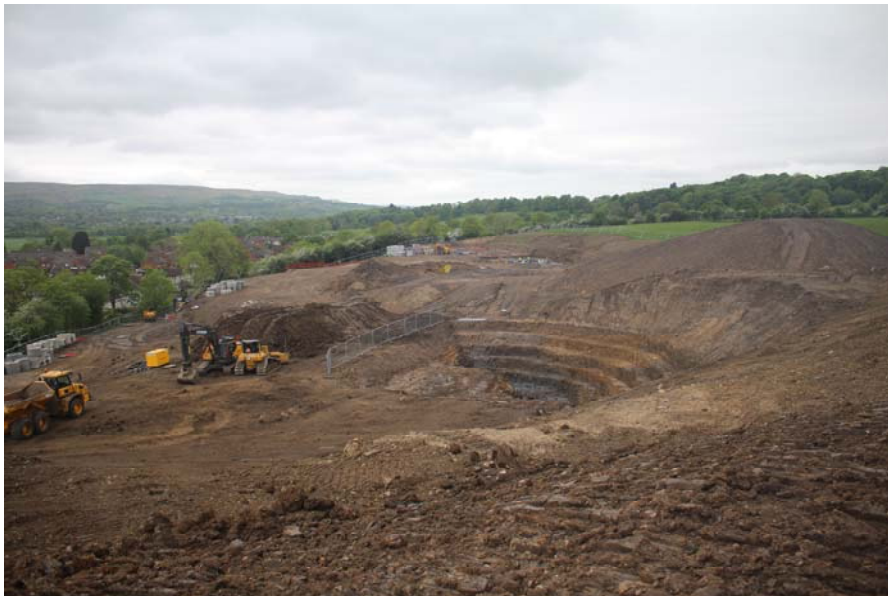
Plate 24: view during earthworks excavations, looking west
