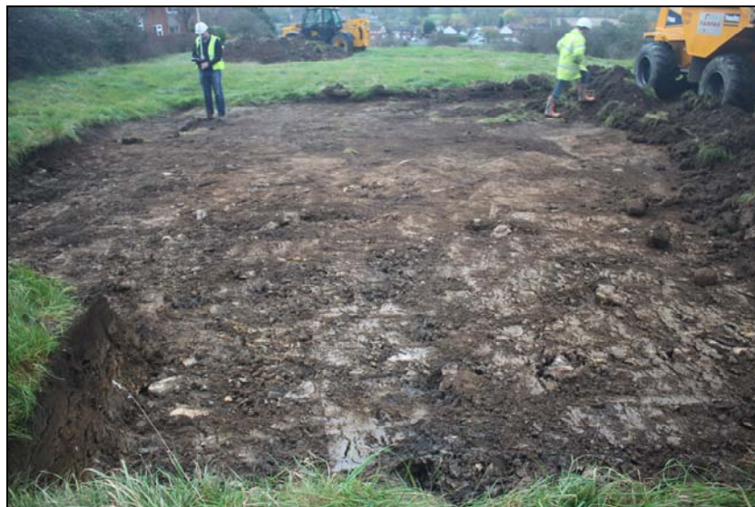
Plate 2: post site strip view of plot 1, looking south
