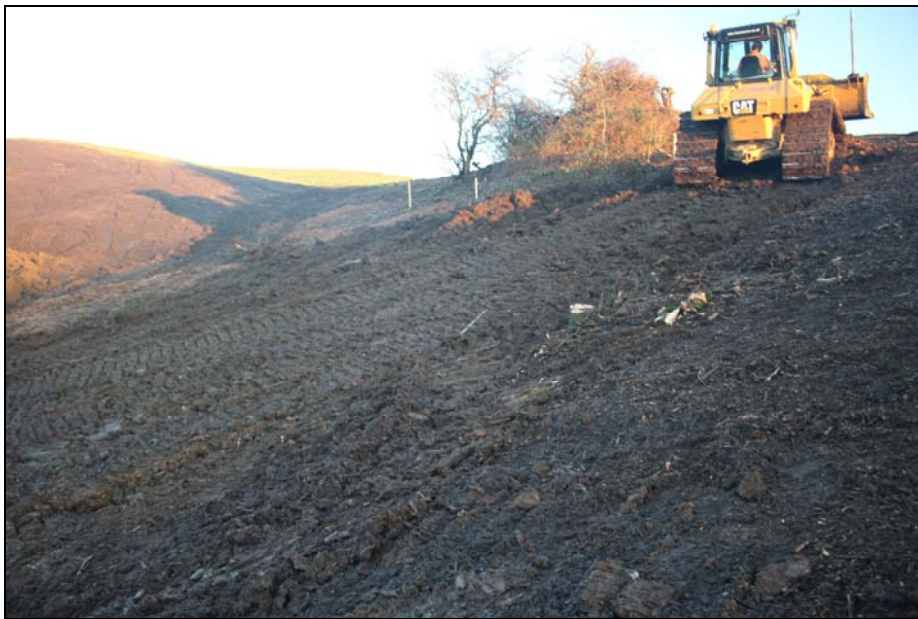
Plate 8: general view of the earth moving operation, looking north
