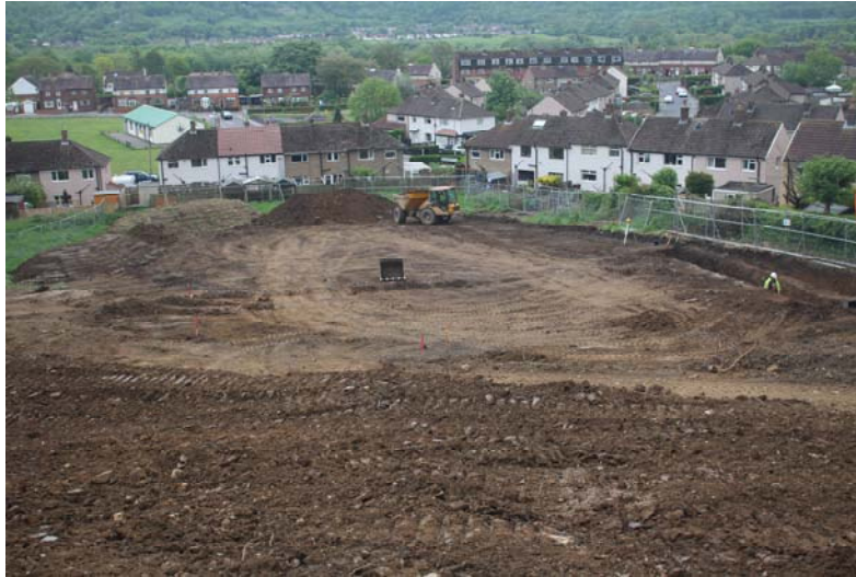
Plate 25: view during earthworks excavations, looking south
