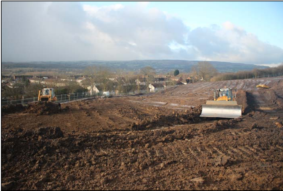
Plate 21: general view during earth re-grading, looking south west
