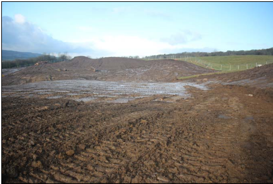
Plate 20: general view following earth re-grading, looking west
