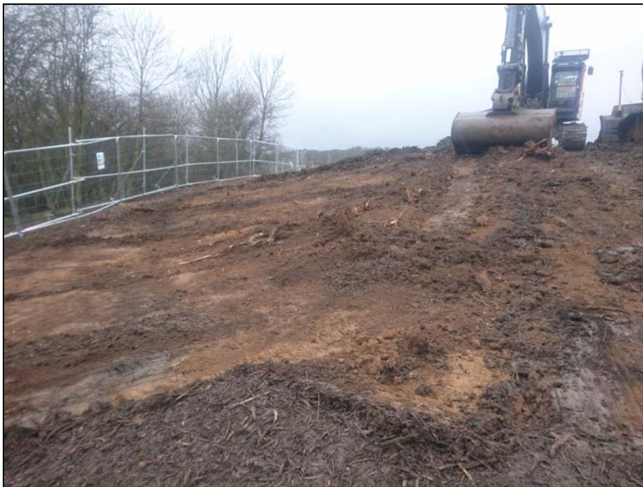
Plate 22: general view during earth re-grading, looking west northwest
