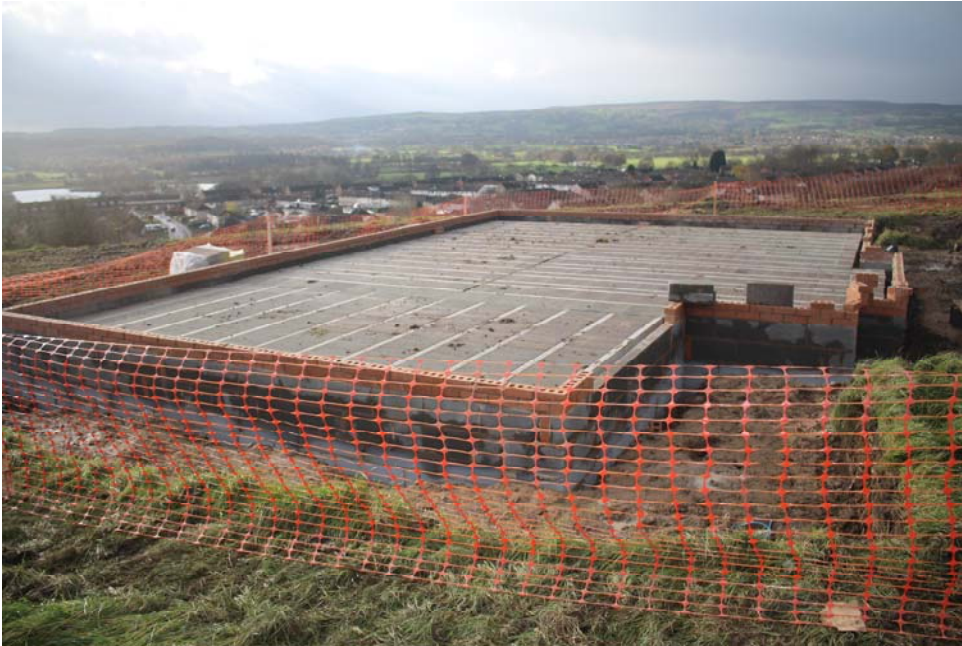
Plate 7: post construction view of plot 1, looking west
