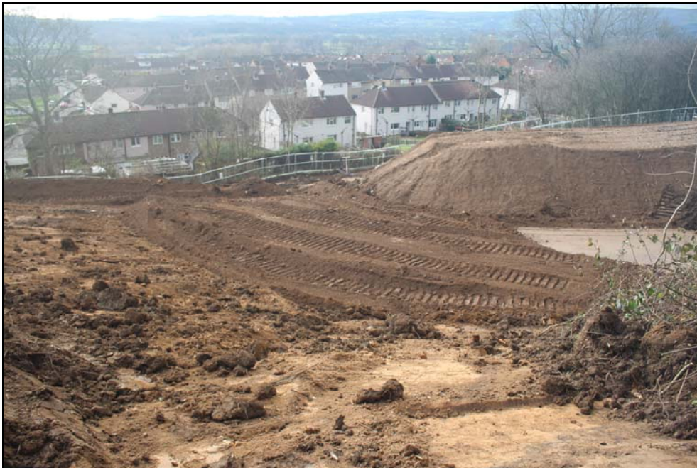
Plate 16: general view, looking southwest
