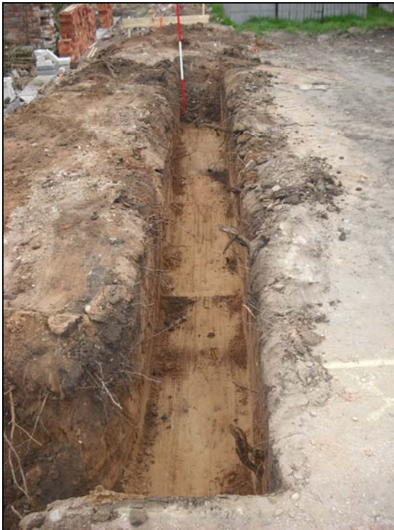
Plate 3, 9: Post Excavation view, looking west northwest
