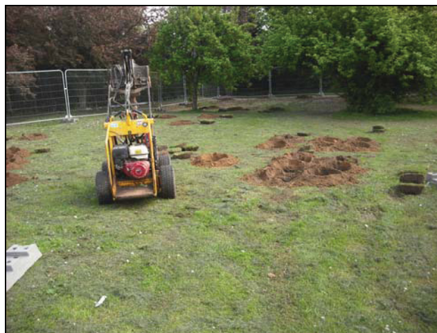
Plate 5, 7: General view, looking northeast
