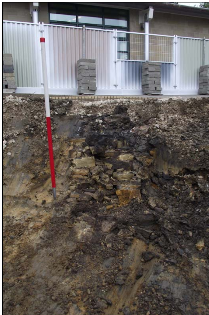
Plate 4, 13: detail of the sandstone walling [005], looking northwest
