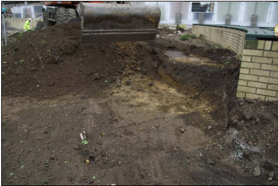
Plate 1, 2: View during removal of overburden, looking northwest
