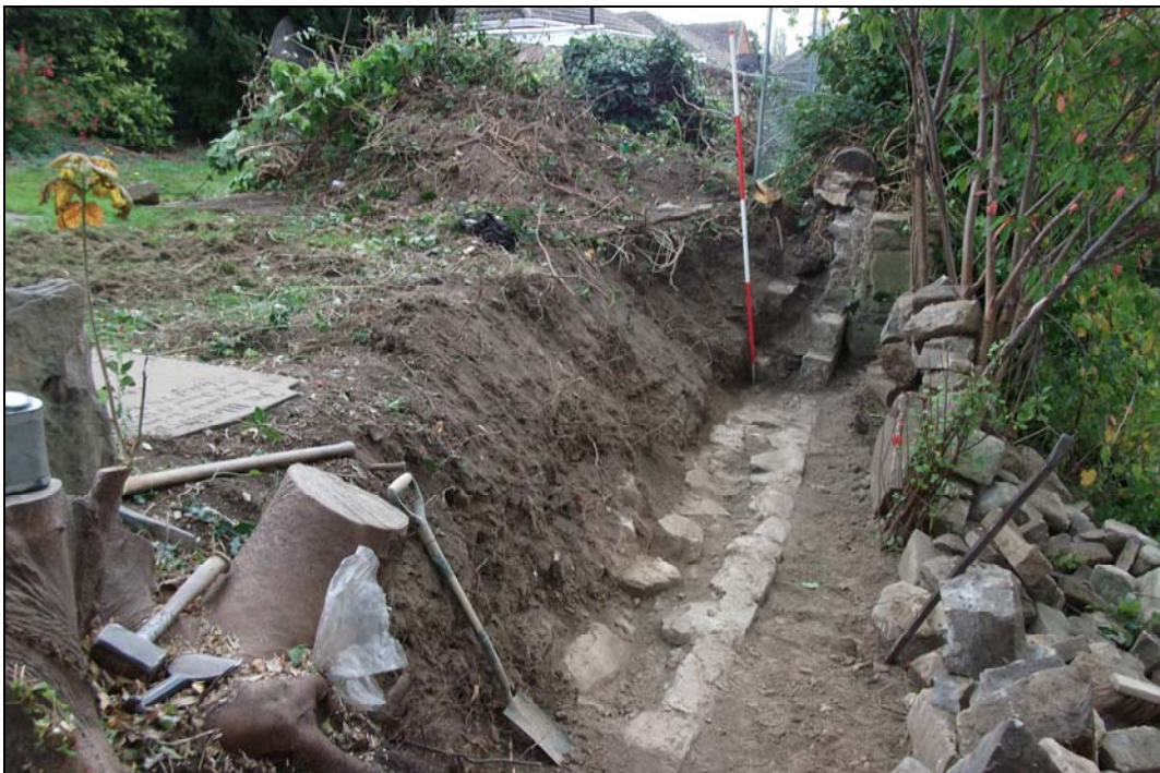
Plate 3: Post-excitation view of the wall during dismantling, looking east
