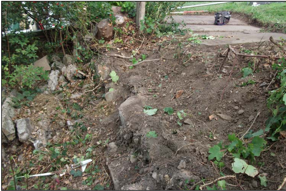
Plate 2: Pre-excitation view of the wall during dismantling, looking west
