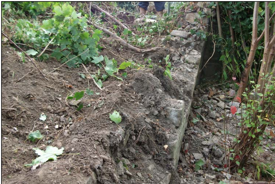
Plate 1: Pre-excavation view of the wall during dismantling, looking east
