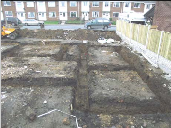
Plate 11, 22: general post excavation view of the site, looking north
