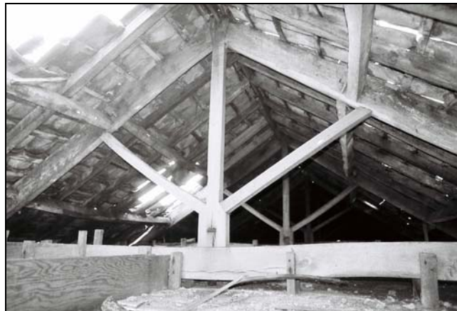
Plate 67 , 310: the shelter shed (Blg.8), general view of the roof with type 1 trusses, from the west
