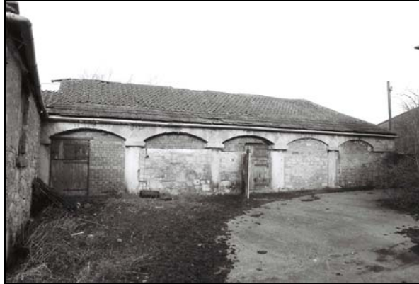
Plate 62 , 273: the shelter shed (Blg.8), view of the front, south elevation with cylindrical piers from the south
