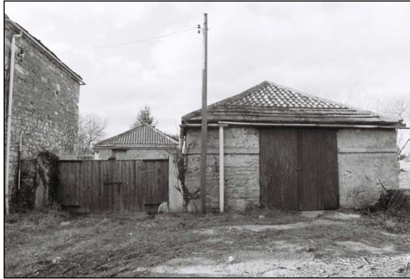
Plate 64, 259: the shelter sheds (Blgs. 8&9), view of the western elevations with string course to building 8, from the east
