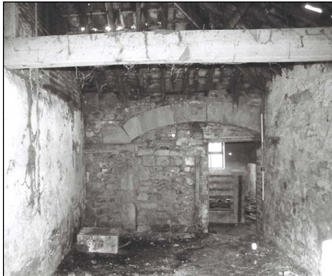
Plate 70 , 264: the shelter shed (Blg.9/48), general view with the blocked arch to the north wall from the south
