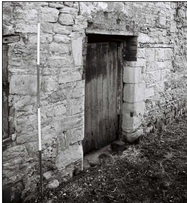
Plate 54 , 279: the barn (Blg.7), oblique detailed view of the chamfered doorway [9], from the north northwest
