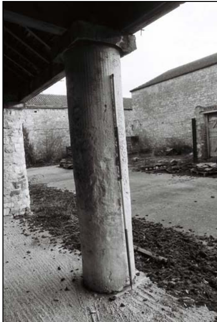
Plate 72, 271: the shelter shed (Blg.7), from the east
